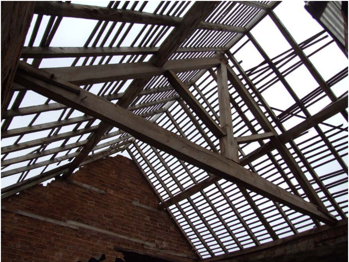
Plate 15: Truss of the two-story eastern extension
