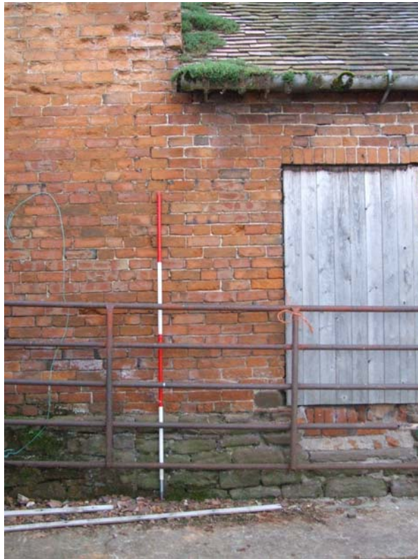
Plate 13: The joint between the original single-storey build of the eastern range and the later two-storey extension (scale 2-metres)
