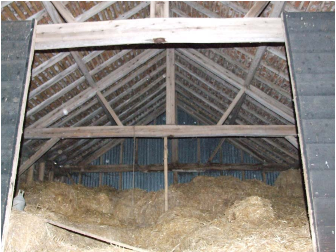
Plate 9: Truss in the timber clad extension
