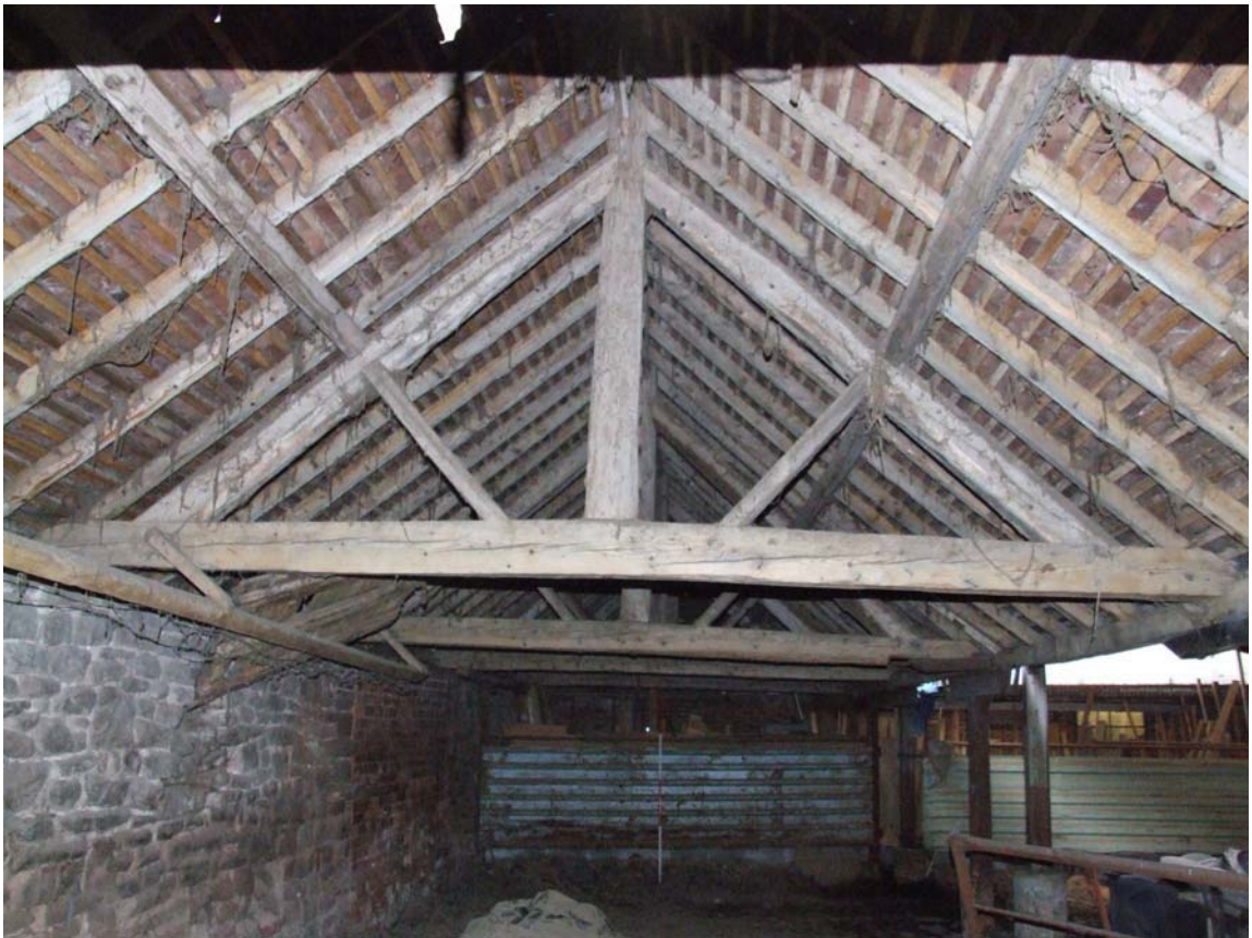
Plate 20: Truss of the northern range
