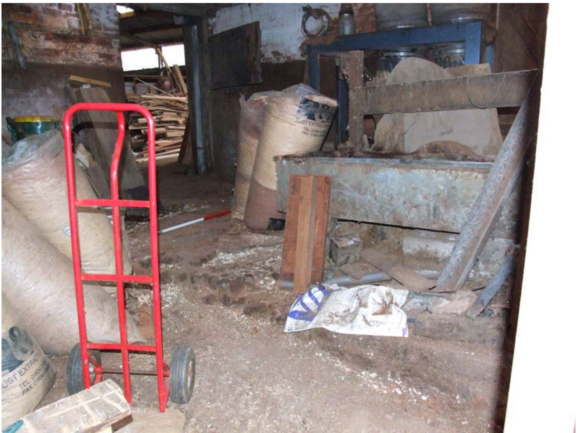
Plate 18: Former cobbled floor can be seen above the later concrete ramp
