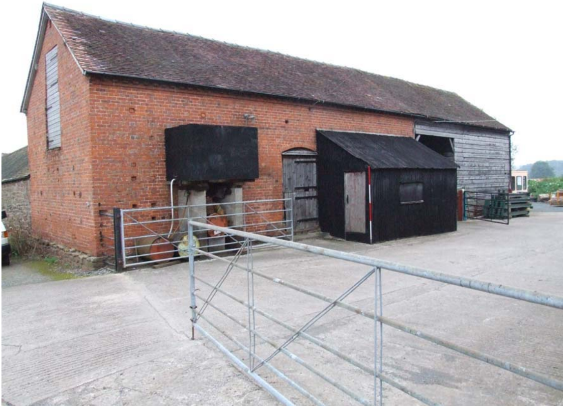
Plate 3: The western range looking south-east (scale 2-metres)
