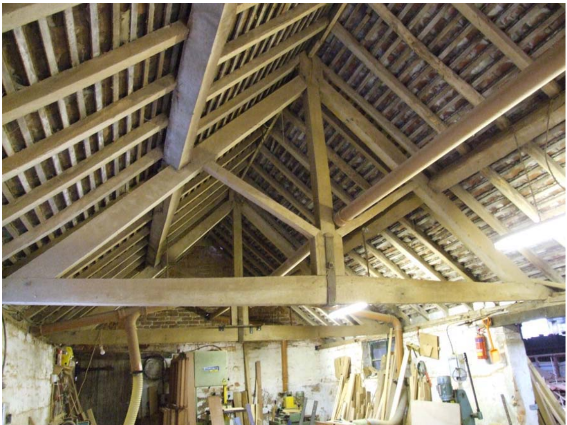
Plate 14: King-post truss in the single storied eastern range
