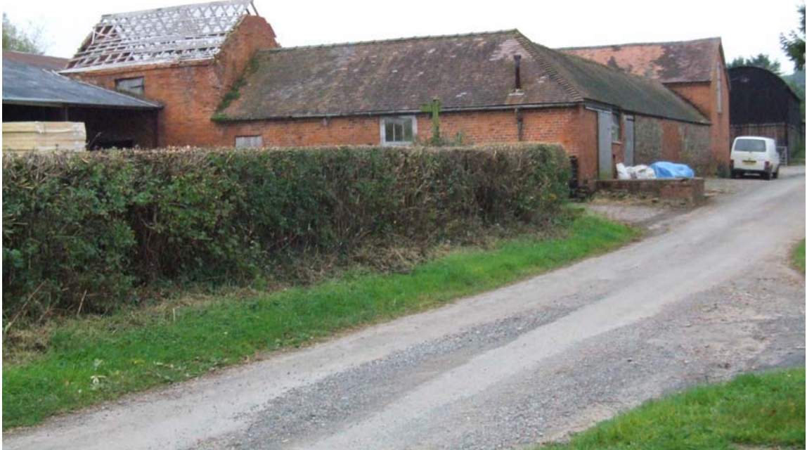
Plate 1: View of the farm buildings complex, looking south-west
