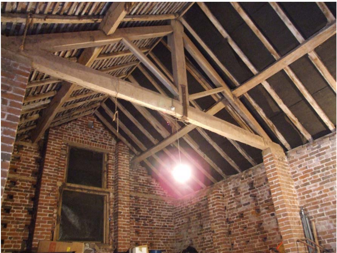
Plate 6: King-post truss in the western range (scale 2-metres)
