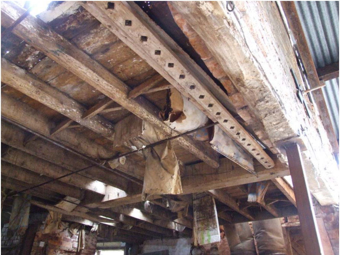
Plate 17: Part of a former hayrack used in the upper floor of the eastern range extension
