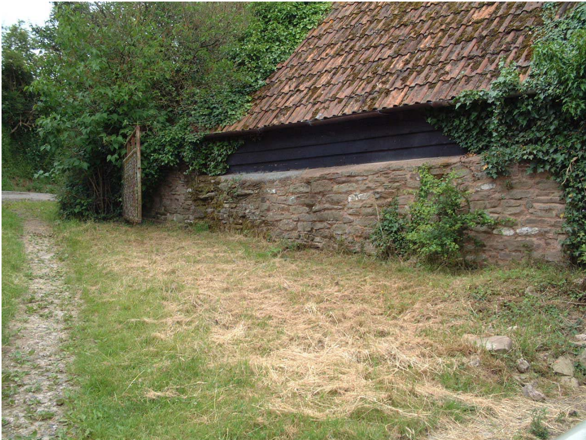
Plate 7: Natural slope of the land against the adjacent farmhouse garden wall, viewed to the east
