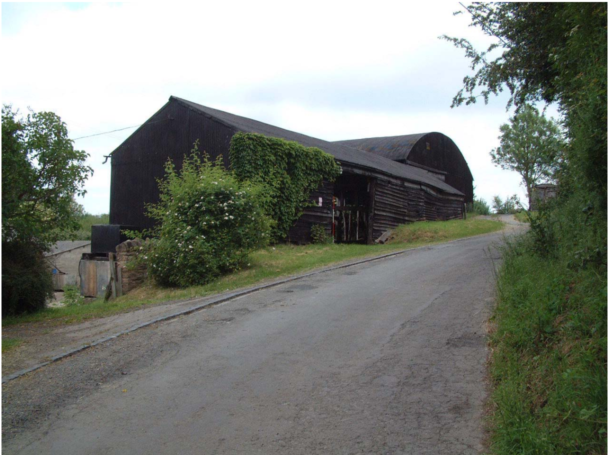
Plate 1: The barn viewed up the slope to the north
