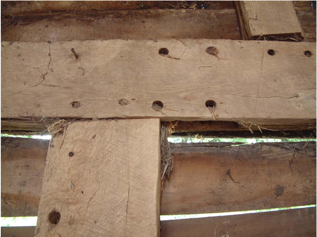
Plate 4: Smaller pegs of the present structure and the larger empty peg-holes of the original build
