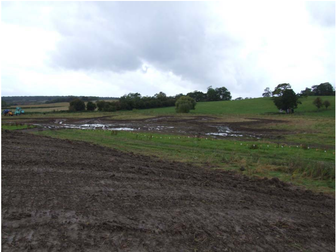
Plate 1: The new reedbeds area under construction, view to the north-west
