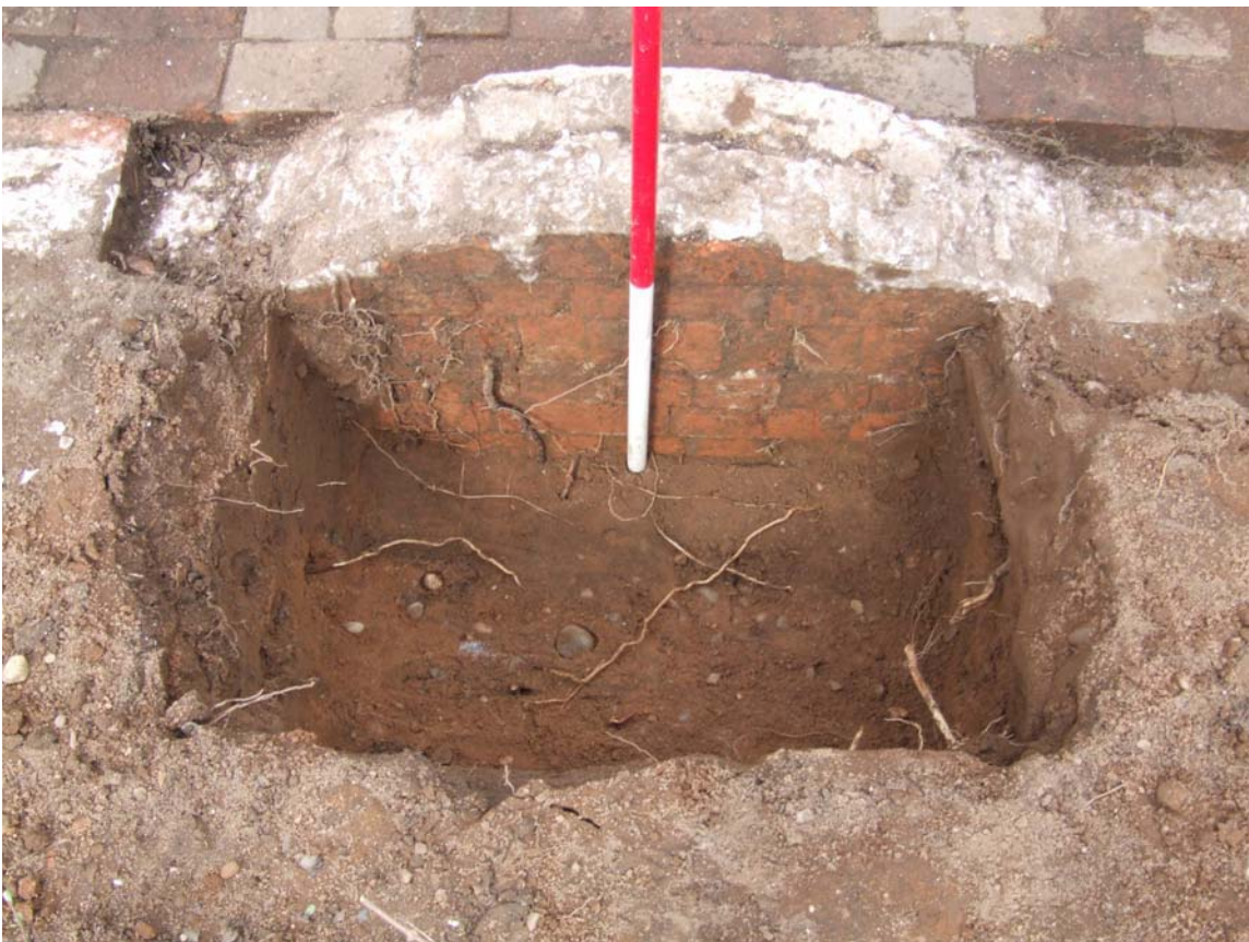
Plate 6: Glasshouse plinth wall foundation trench against the arch
