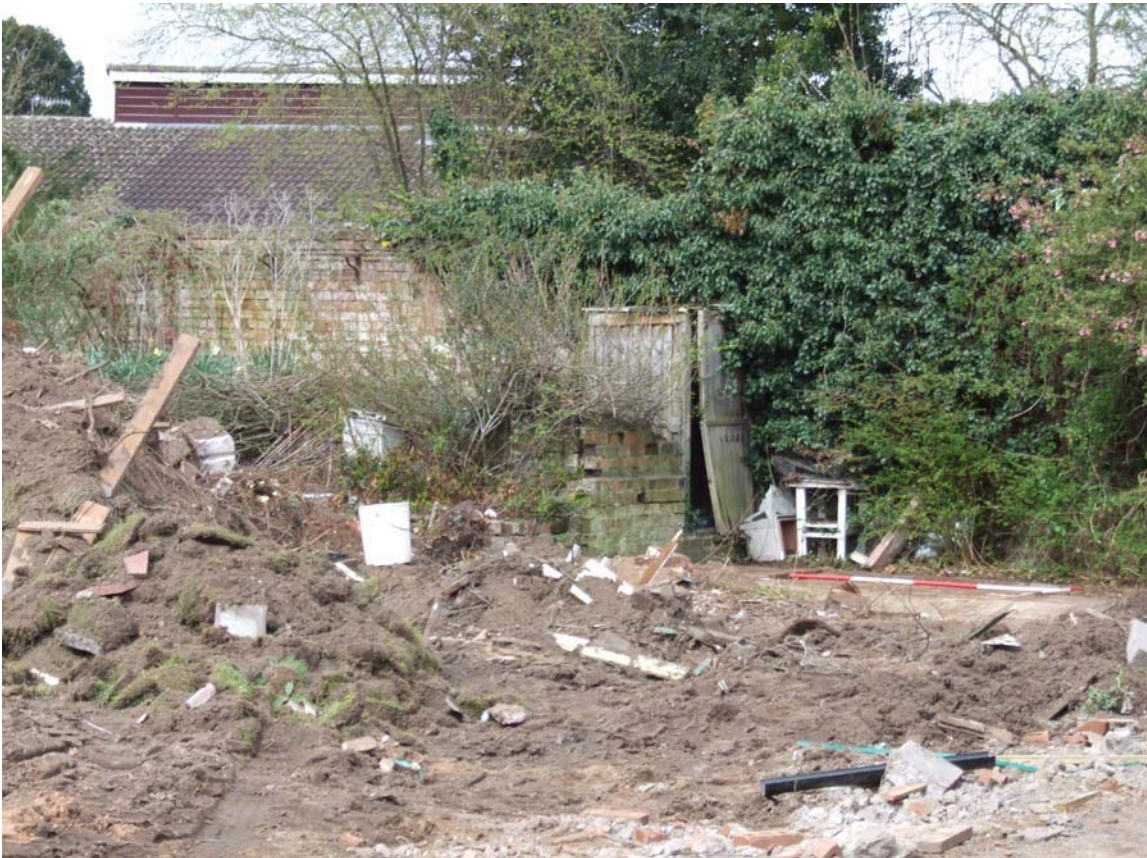
Plate 2: Victorian garden wall to rear (north) of site
