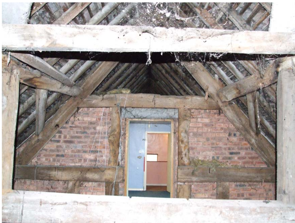
Plate 6: Truss T2 looking north-west. The doorframe cuts through the tiebeam
