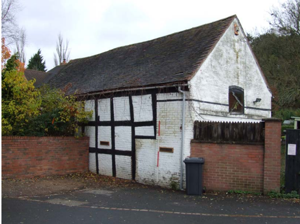
Plate 4: Timber-framing to the south-western elevation (scale 2-metres)
