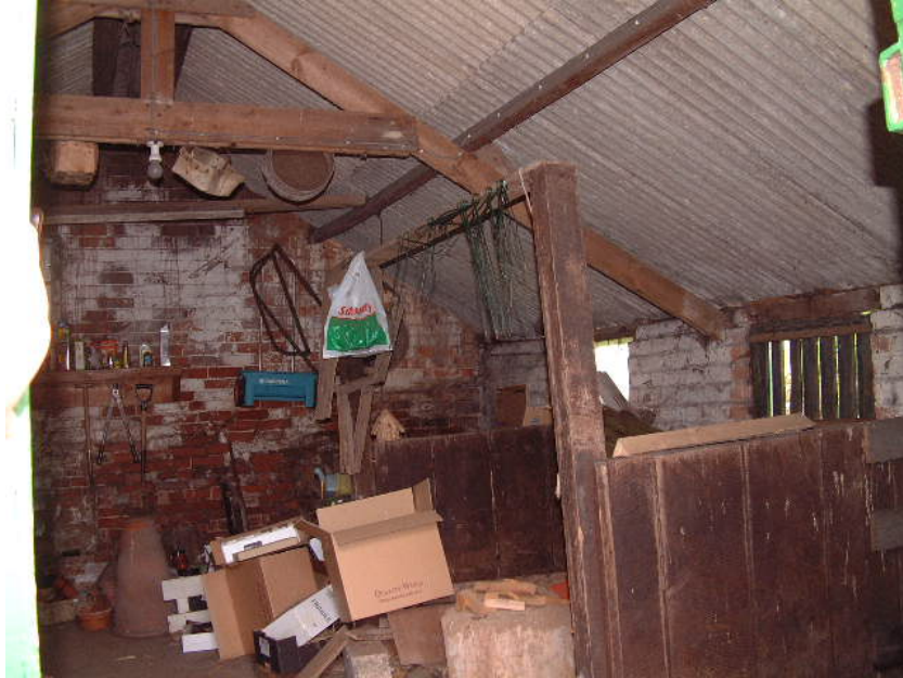
Interior of Building 2 showing stalling
