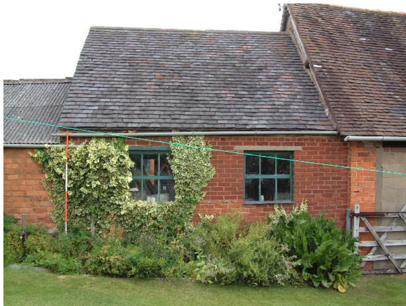
Building 3 viewed to the east (scale 2 metres)
