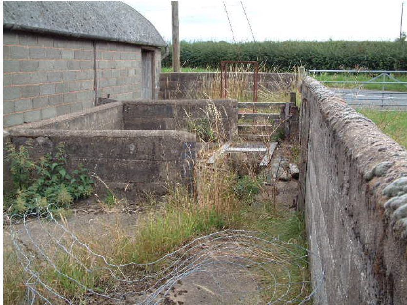
Sheepwash to the rear (south) of Building 6
