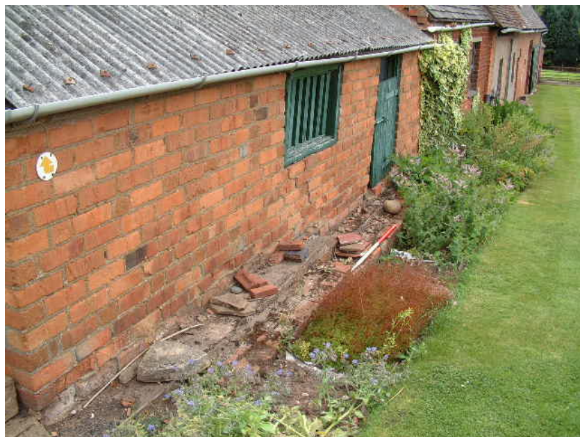
Building 2 viewed to the south-east showing earlier wall (scale 1 metre)
