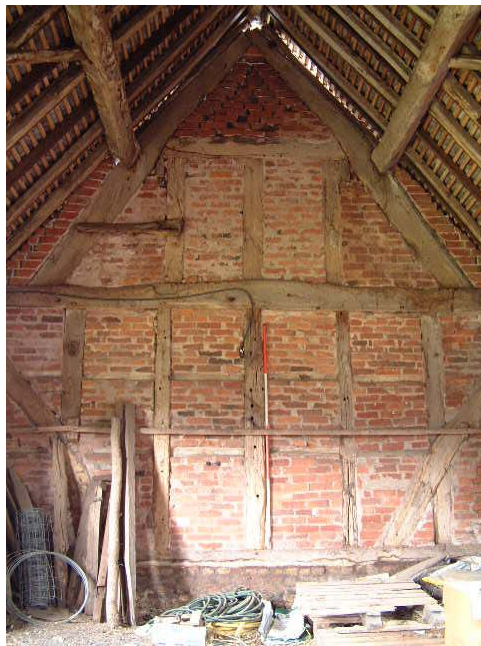
Timber-frame of northern gable end of Building 4, Space A (scale 2 metres)
