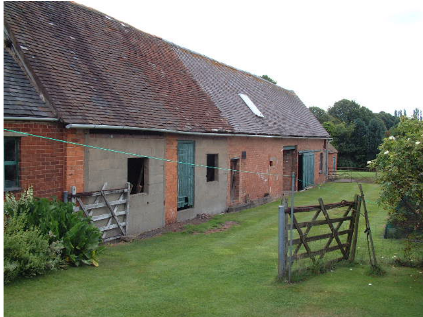
Building 4 view to the south-east (scale 2 metres)
