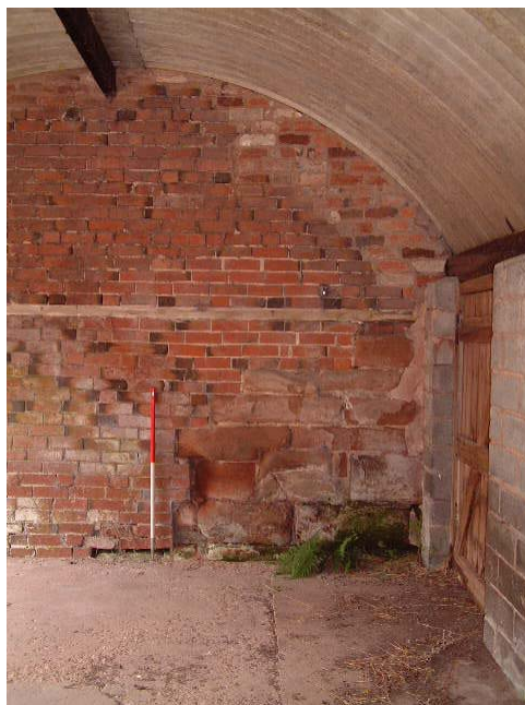
Eastern elevation of Building 6, note the sandstone and the line of a former pitched roof (scale 1 metre)
