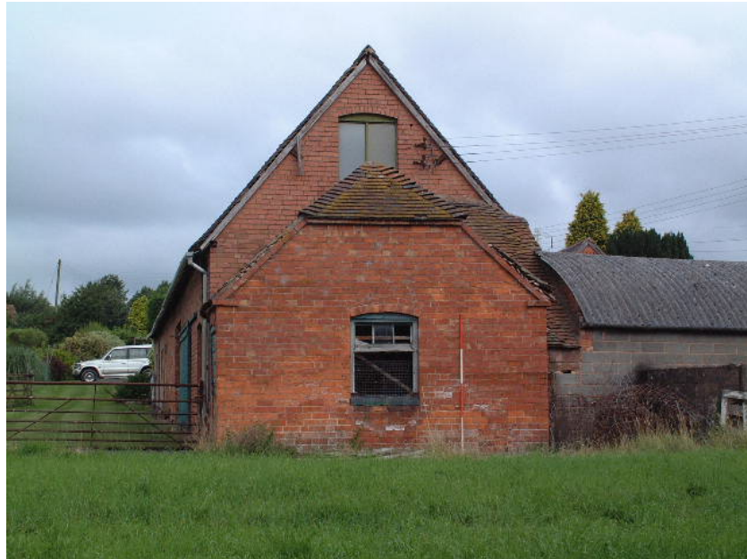
Building 5 at the southern end of Building 4 (scale 2 metres)
