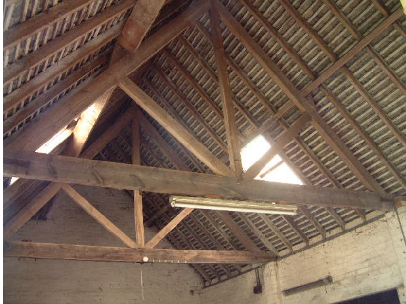
Trusses in Space B of Building 4
