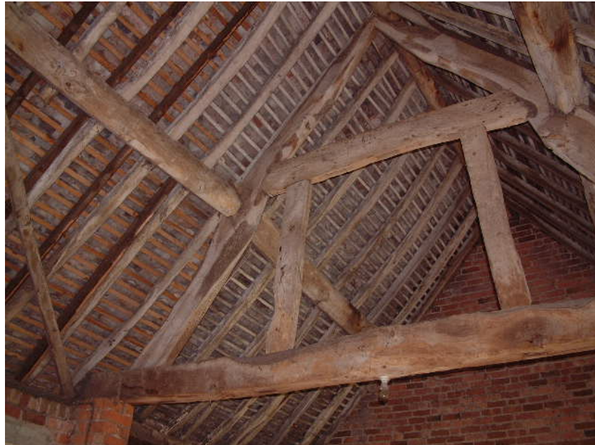
Truss T2 in Space A of Building 4
