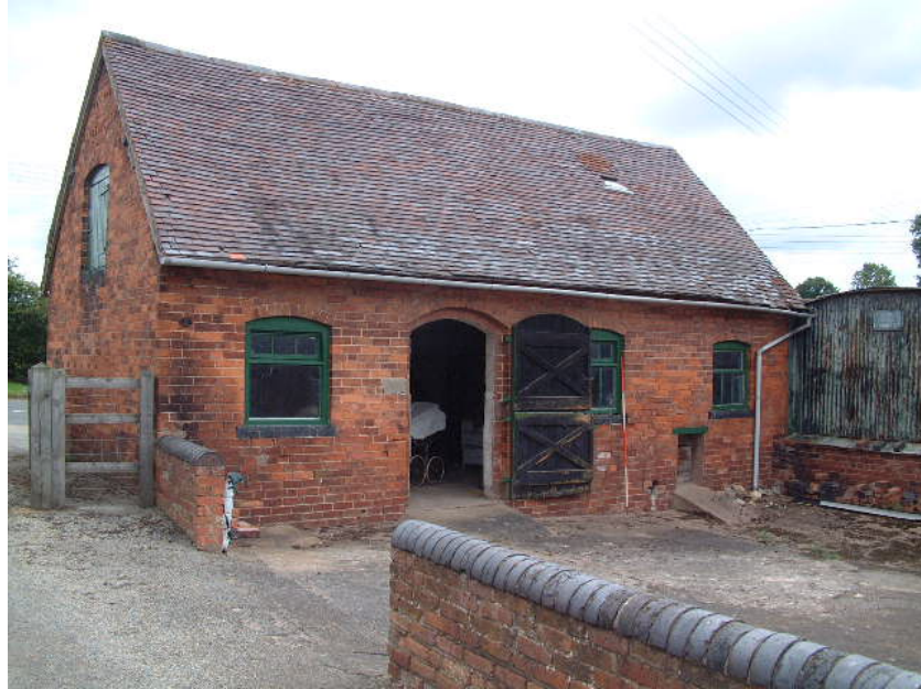
The stable block (Building 1) looking east (scale 2 metres)
