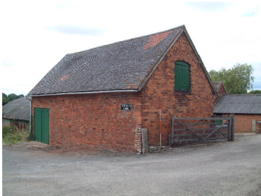
The stable block (Building 1) looking west (scale 2 metres)
