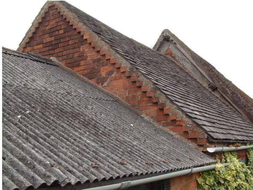
Principal rafters in gable end of Building 4 (far), also note shadow of former roofline on gable of Building 3
