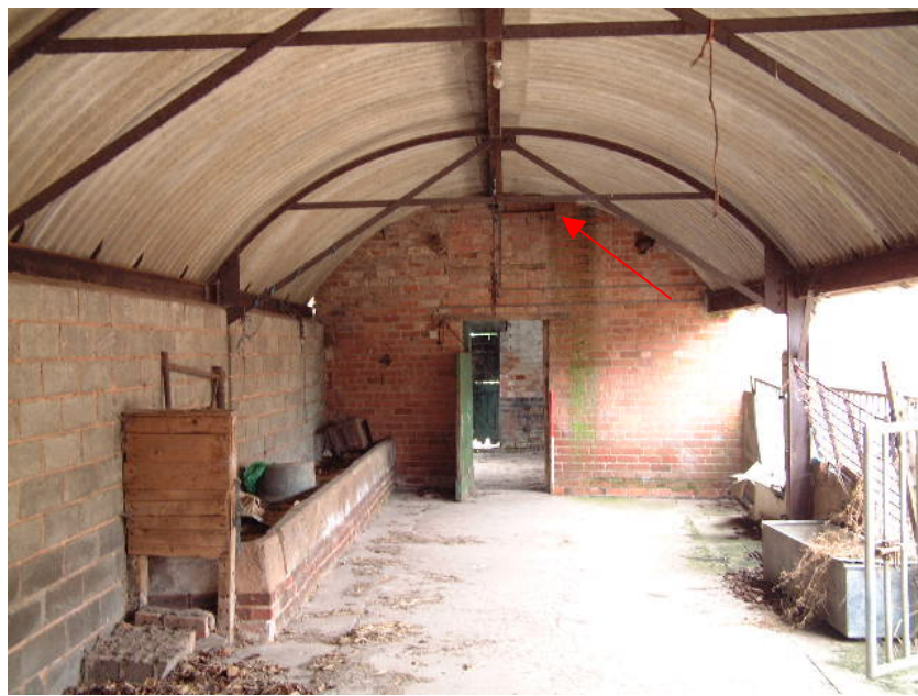
Eastern elevation of Building 4 where Building 6 butts it, note the blocked aperture (arrowed) (scale 1 metre)
