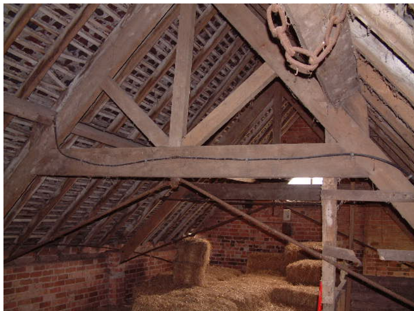
Trusses in Space C of Building 4
