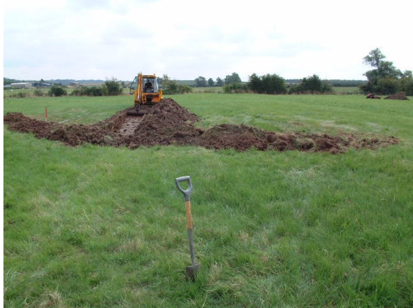
Trench B during excavation, looking south
