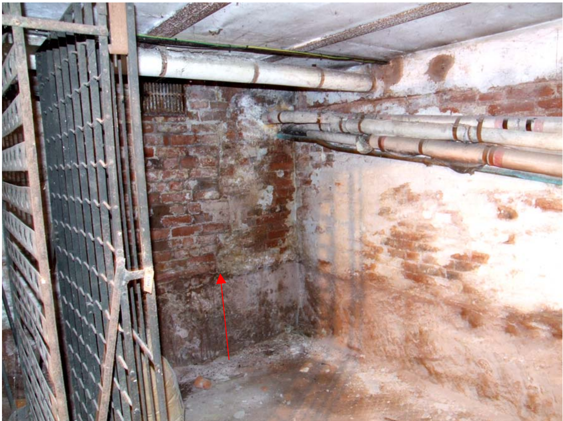
Plate 6: Cellars below the 17 th century wing (bricks to right of arrow are earlier than those to left)
