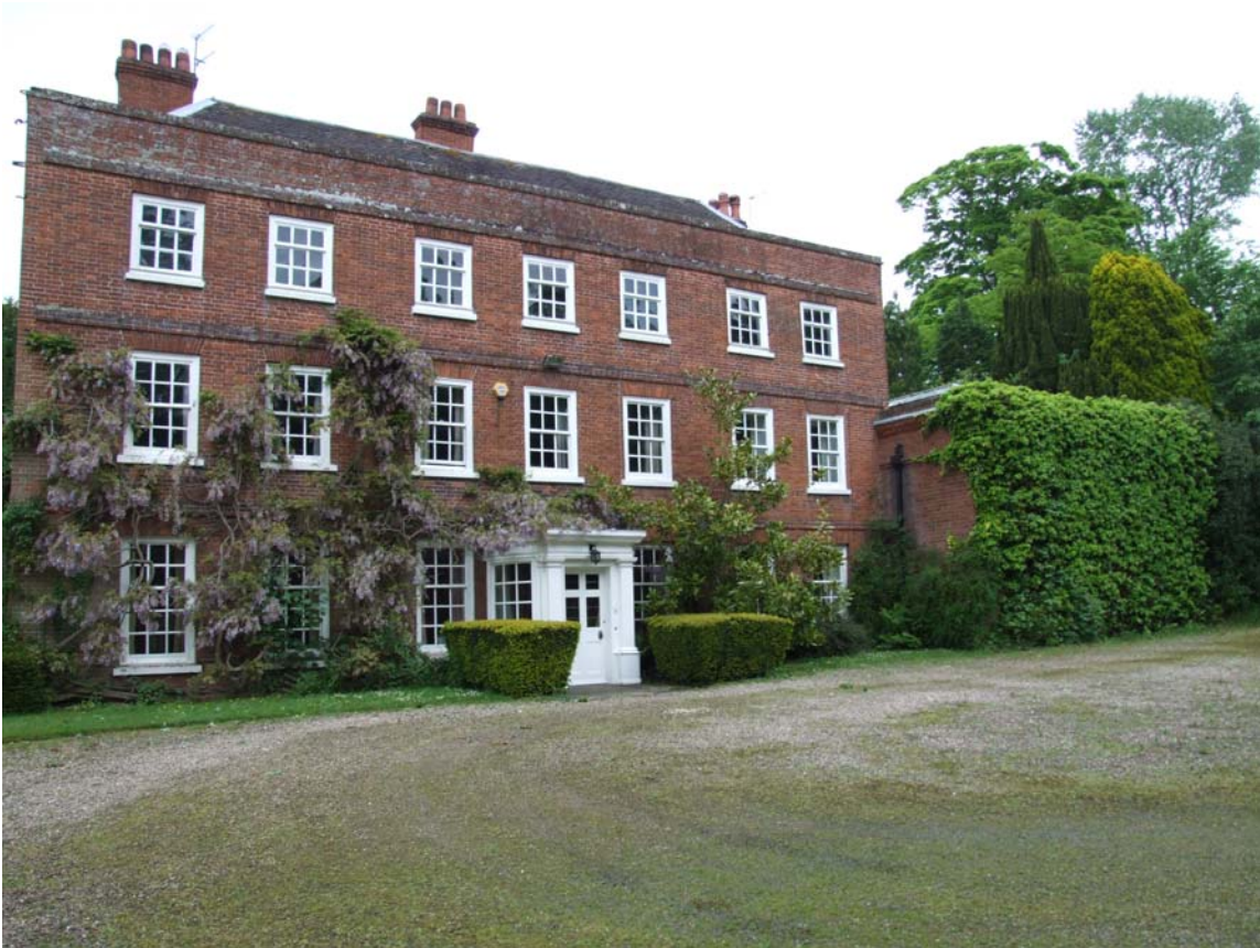
Plate 1: Stone House south elevation looking north-east
