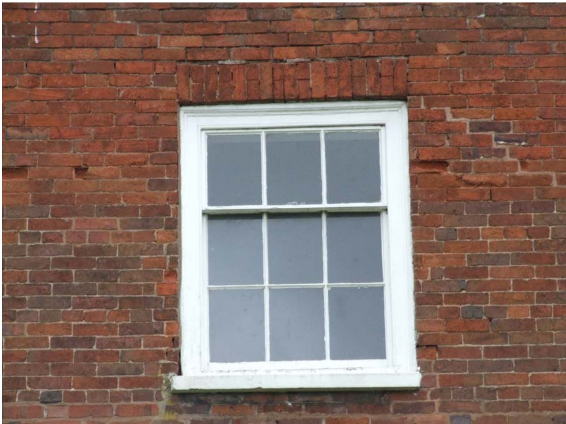
Plate 12: Later replacement sash with slender glazing bars, circa 1860
