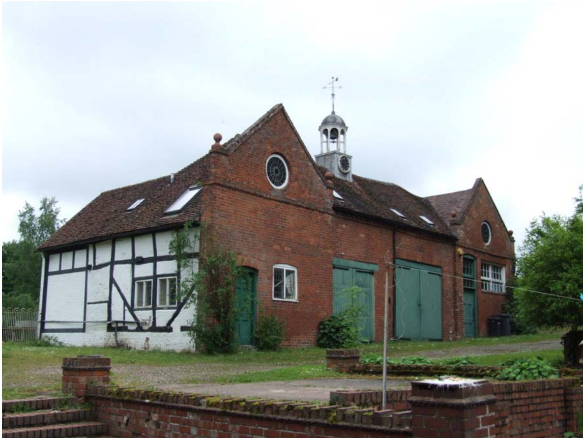
Plate 21: Stable and coach house looking north-east
