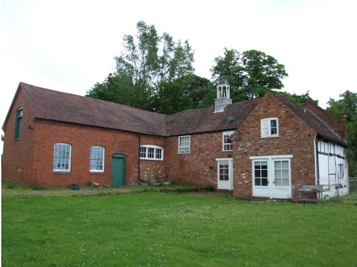
Plate 23: The stables complex looking south-east
