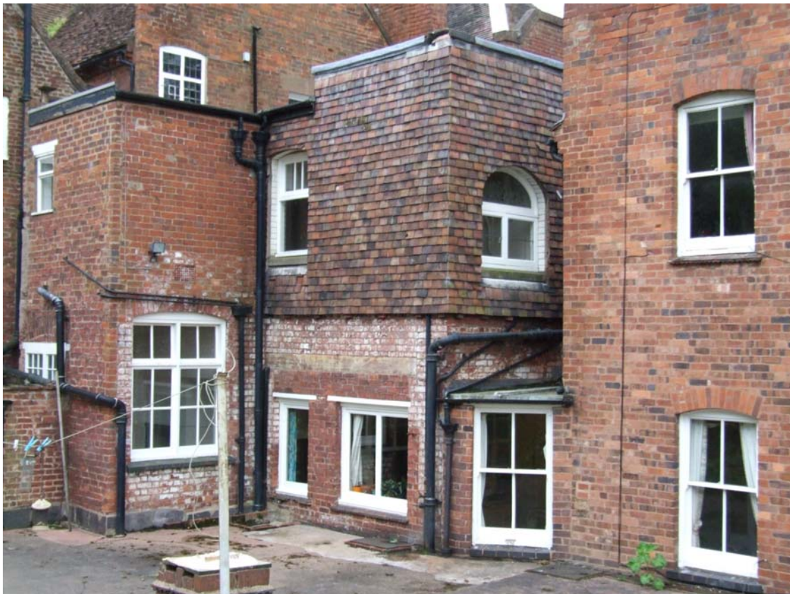
Plate 20: Infilled building of the early 20 th century kitchen (centre)
