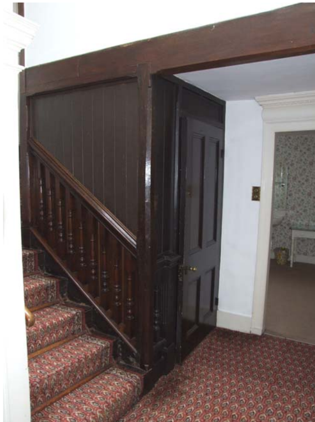
Plate 8: 18 th century rear staircase in 17 th century wing
