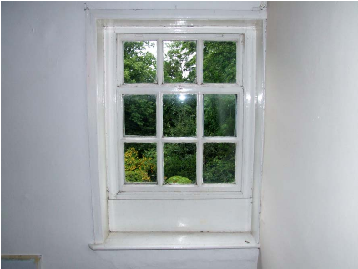
Plate 11: Early sash with wide glazing bars (astragals), circa 1720
