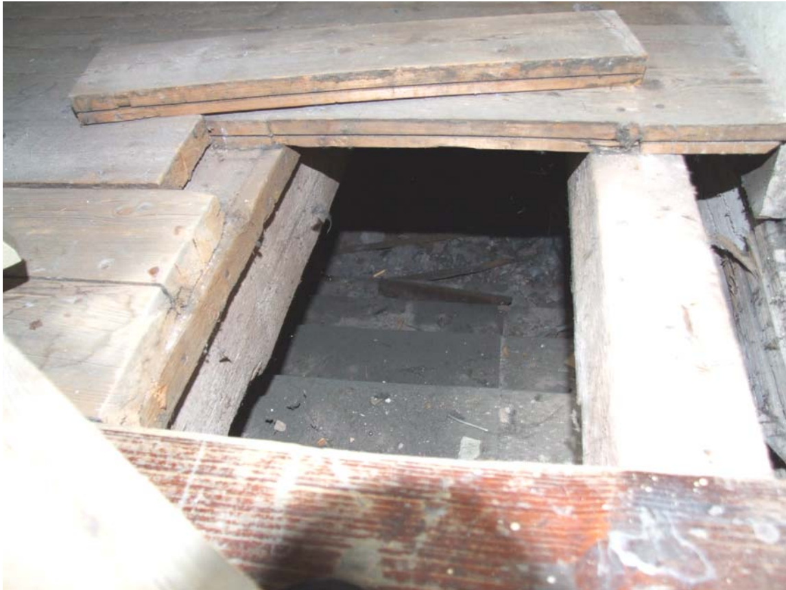
Plate 9: Stair treads below floorboards, possibly 17 th century
