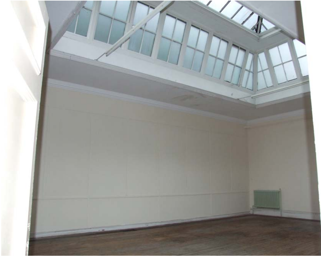
Plate 19: Inside the eastern annexe / gallery
