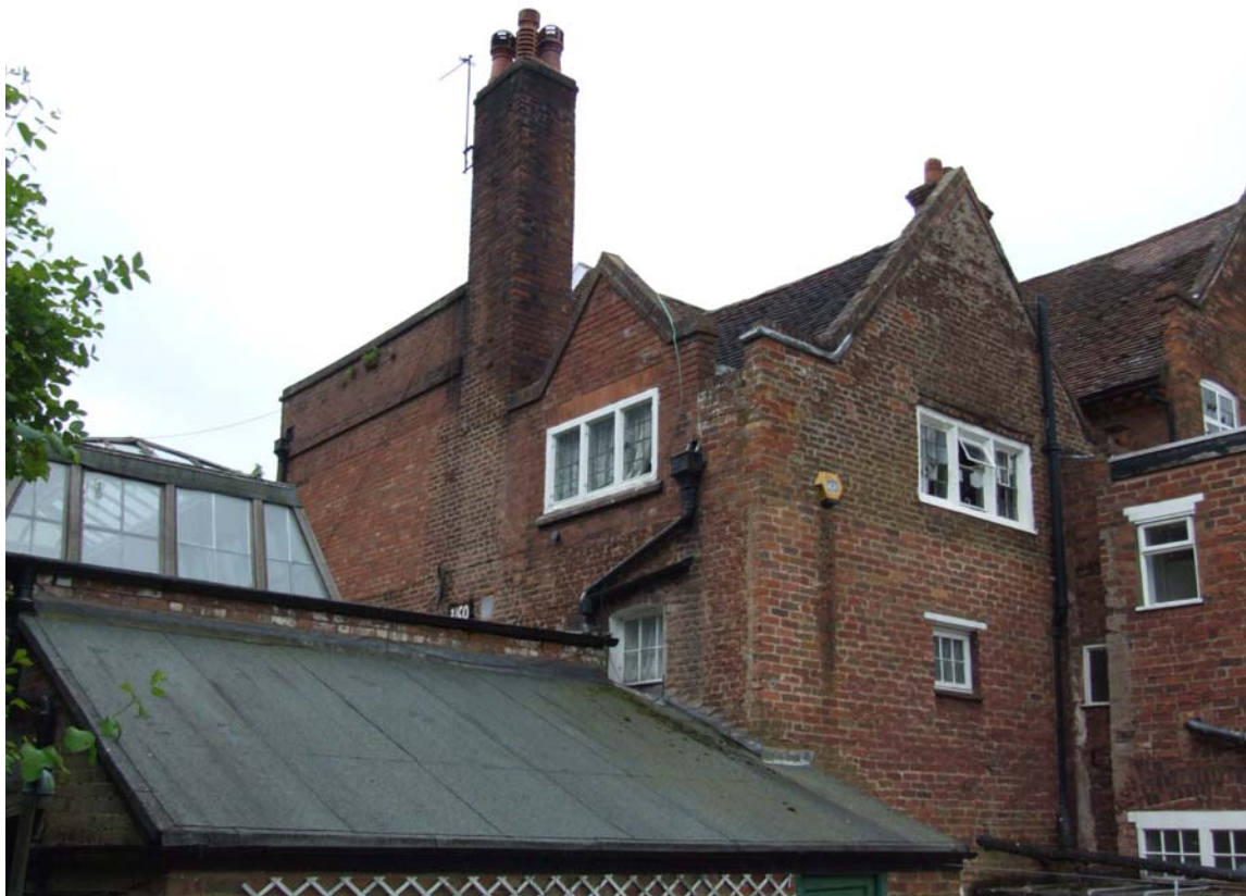
Plate 4: 17th century wing looking south-west
