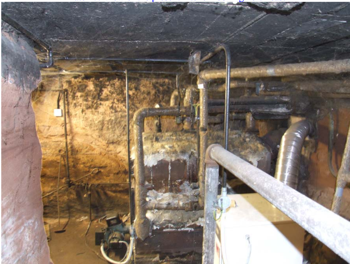
Plate 18: Rock cut cellar below the early 20 th century eastern annexe
