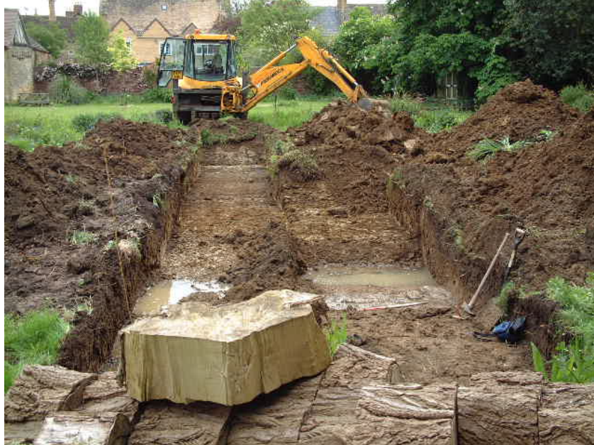
Work in progress looking east
