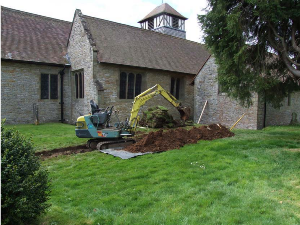
Plate 1: Work in progress, view to the south-west
