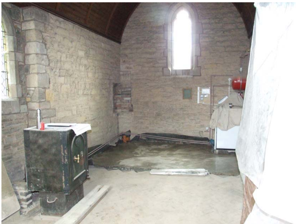
Plate 4: Interior of the vestry following reinstatement of concrete floor raft
