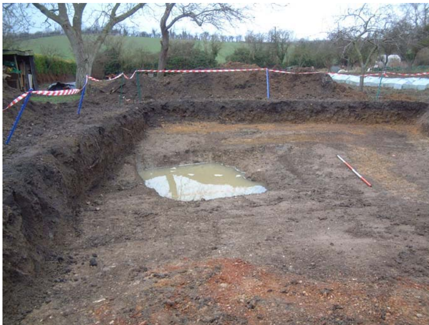
Pit feature [115] with waterlogged test-pit (Scale 2 metres).
