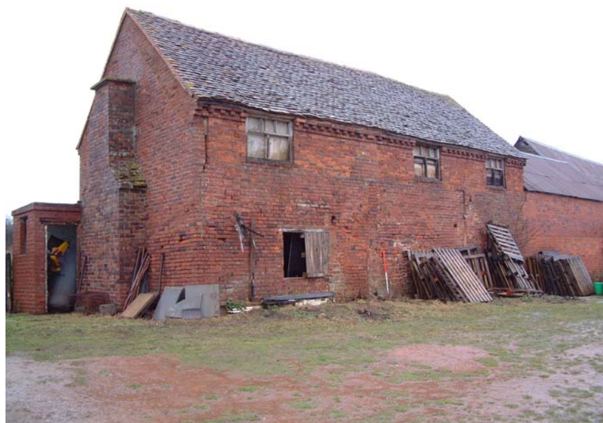
The workers cottage south-east elevation (scale 1 metre)
