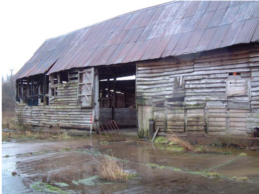
The barn viewed to the west (scale 1 metre)
