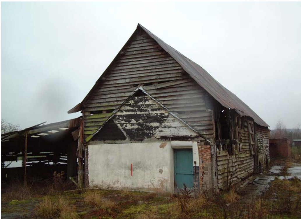
The barn showing location of a former building to the north-east (scale 1 metre)
