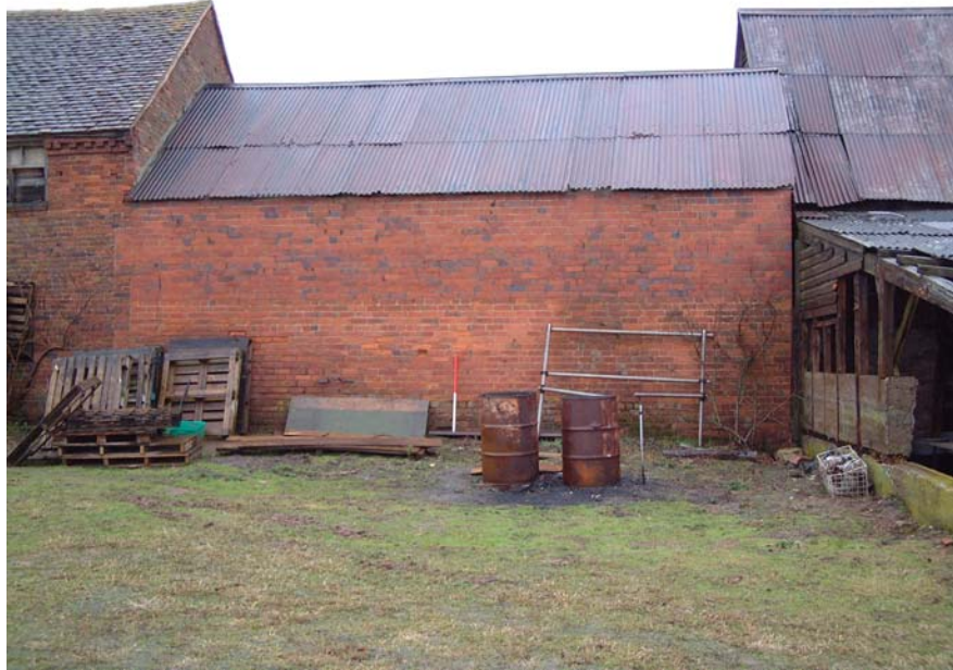
The fodder processing shop south-east elevation (scale 1 metre)
