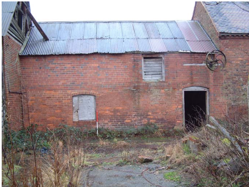
The fodder processing shop north-west elevation (scale 1 metre)
