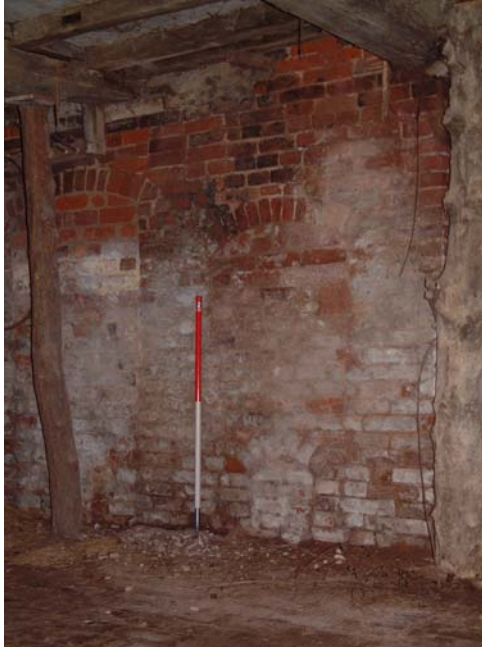
Bricked up doors and 'dog door' in the workers cottage (scale 1 metre)
