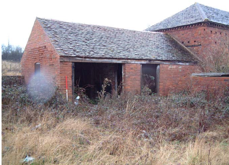
The single storey stable and loosebox (scale 1 metre)
