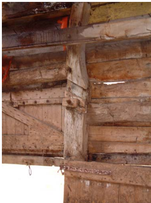
Another re-used section of cruck framing in the barn
