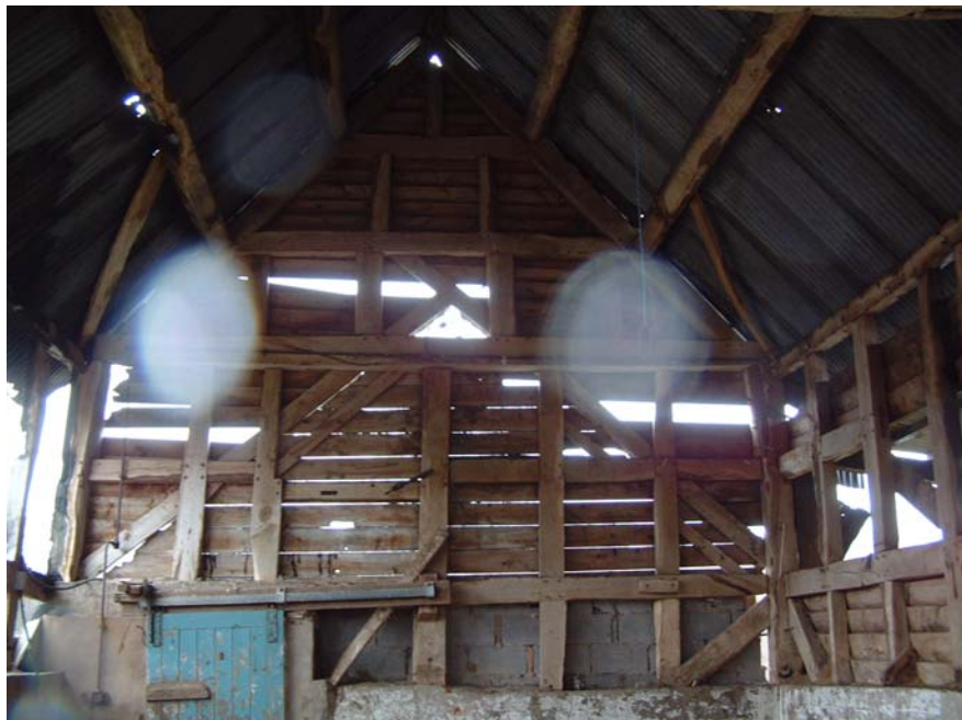
Truss T1 at the south-western end of the barn (scale 1 metre)
