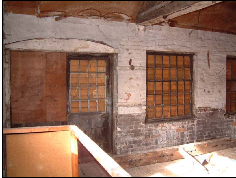
Upper floor of the three-storey build showing the loading doors
