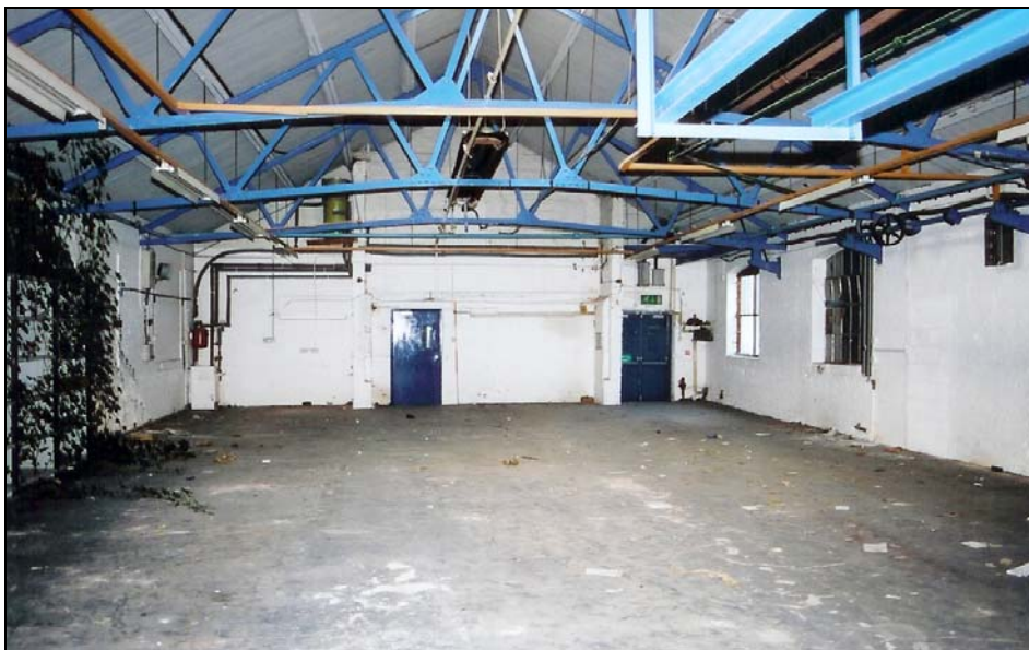
The northern end of the three-storey build where it is butted by the 1915 extension. The side walls of the original mill building project forward, adjacent to the blue doors
