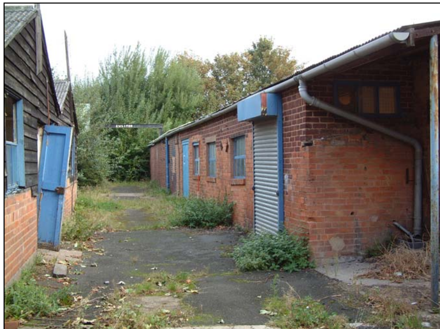
Lean-to building's obscuring the 1958 extension at the northern end
