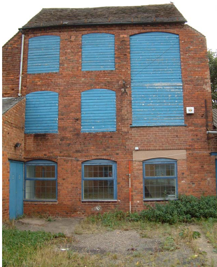
Western elevation of the former three-storey mill building (Scale 2 metres)
