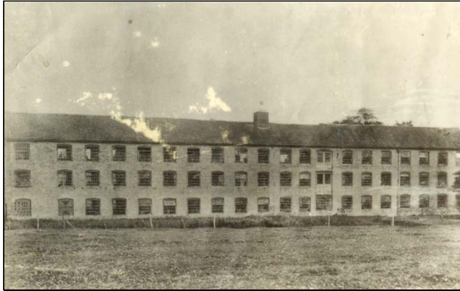
Photograph of The Button Factory taken at the end of the 19 th century (Supplied by Mr E.Waldron)
