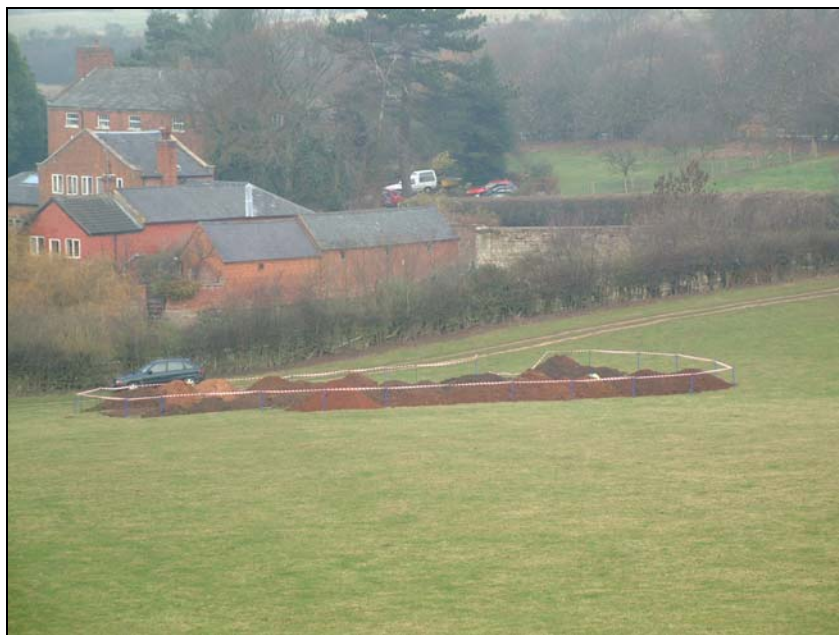
The site, showing extent of trenching; view to the north from Church Hill
