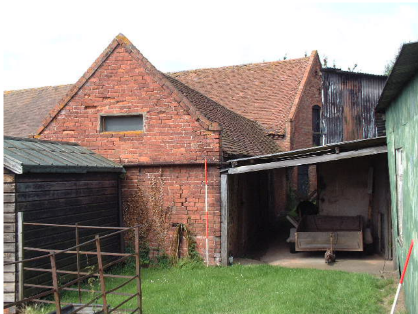
The stables eastern gable (Scale 2 metres)
