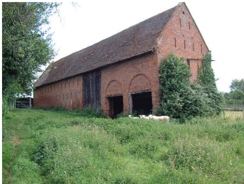
The barn western elevation (Scale 2 metres)
