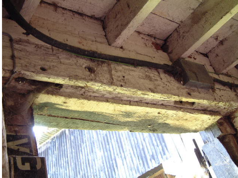
Re-used timber-framing above entrance door in northern gable
