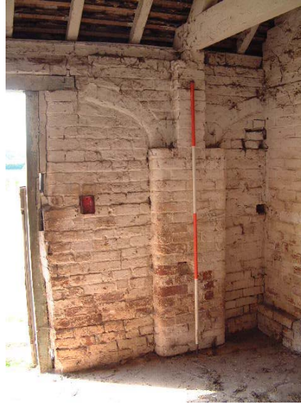
Blocked up entrances inside current stables (Scale 2 metres)
