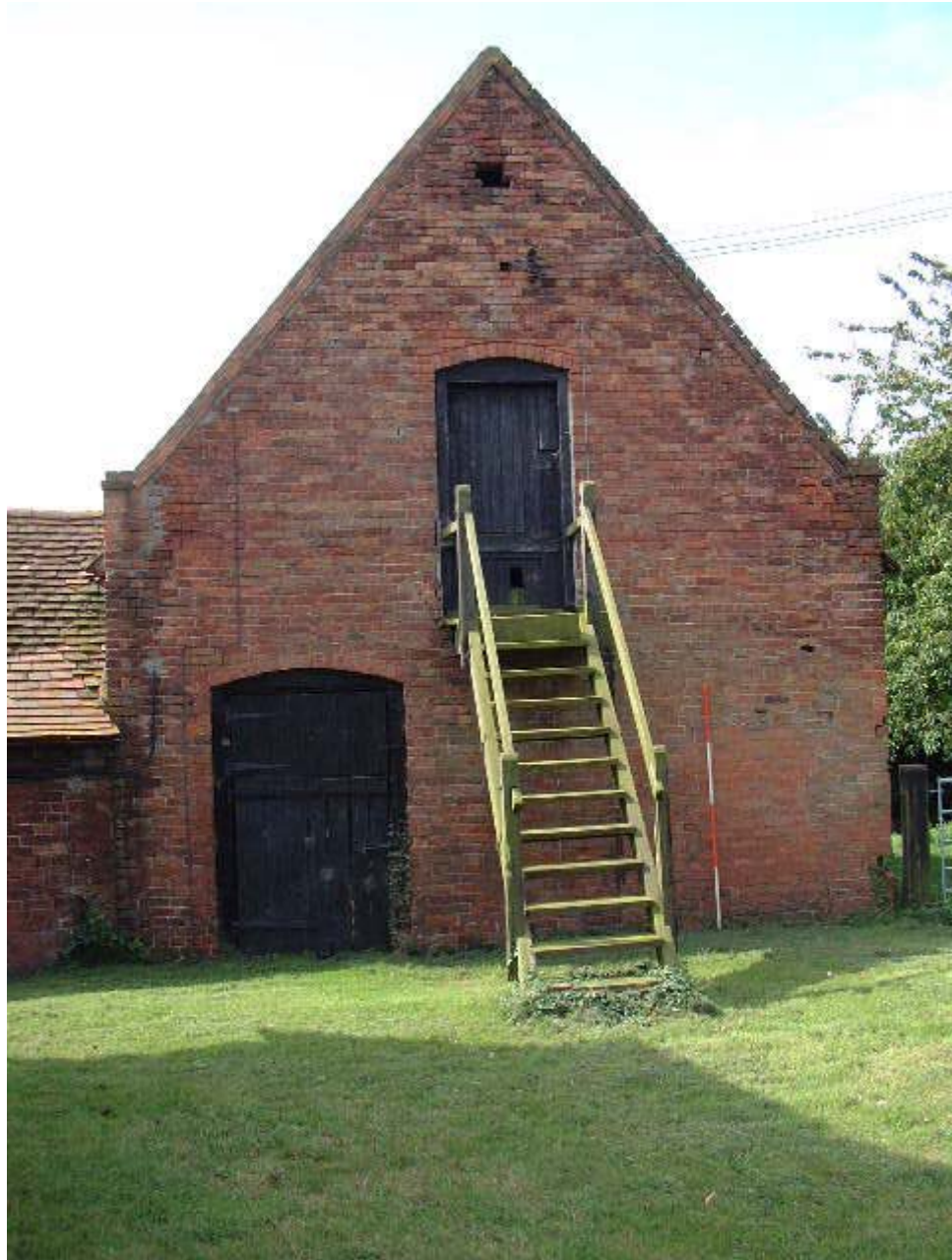
The barn north gable end (Scale 2 metres)
