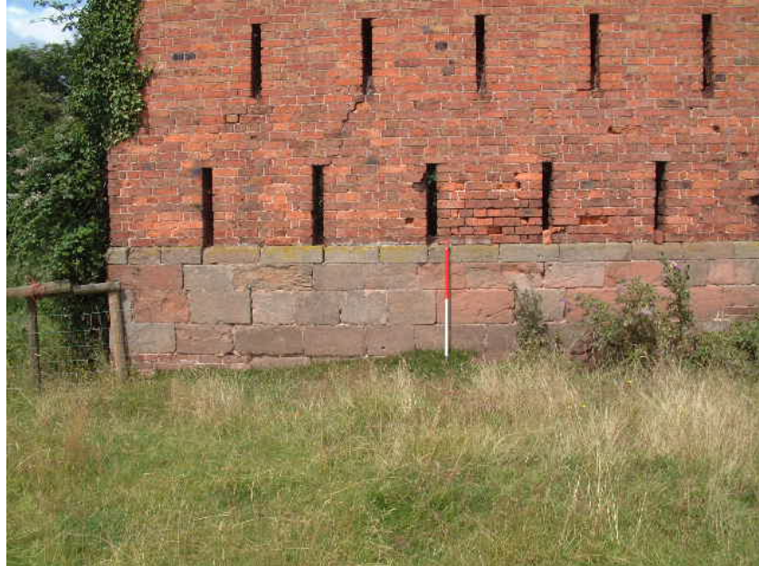
Sandstone plinth at southern end of eastern elevation of barn (Scale 1 metre)
