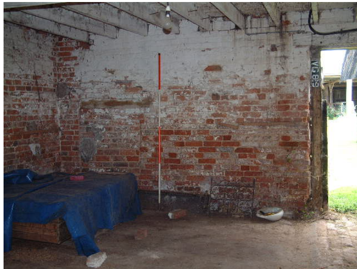
Blocked up doorway in north gable of barn (Scale 2 metres)
