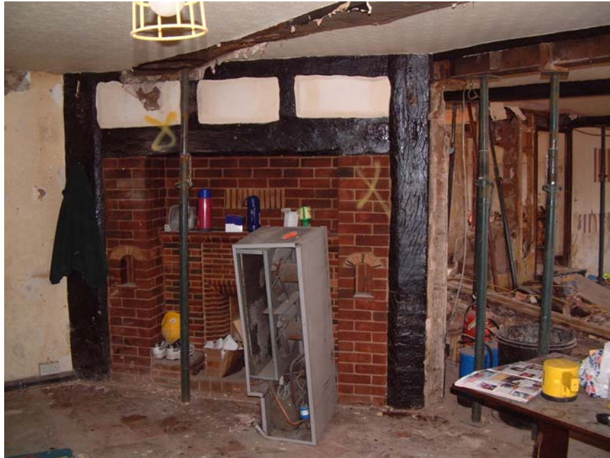
Timber-framing inside the pub
