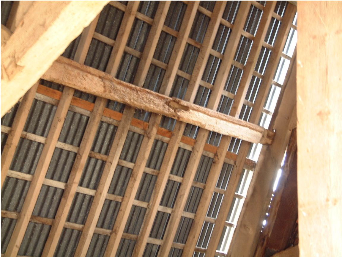
Plate 9: North purlin in bay 3 showing evidence of reuse
