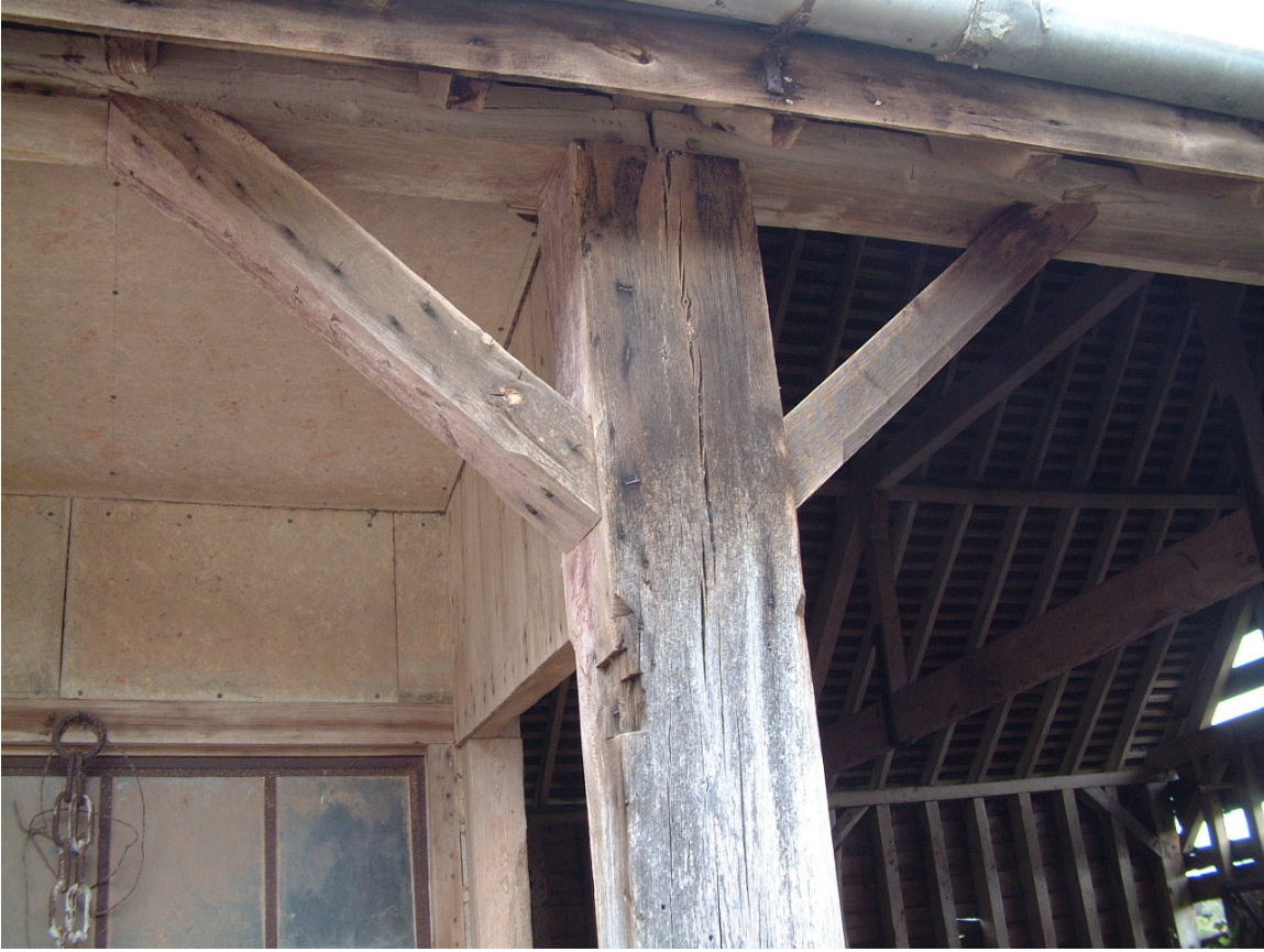
Plate 13: Chamfered and stopped braces and post of the shelter shed
