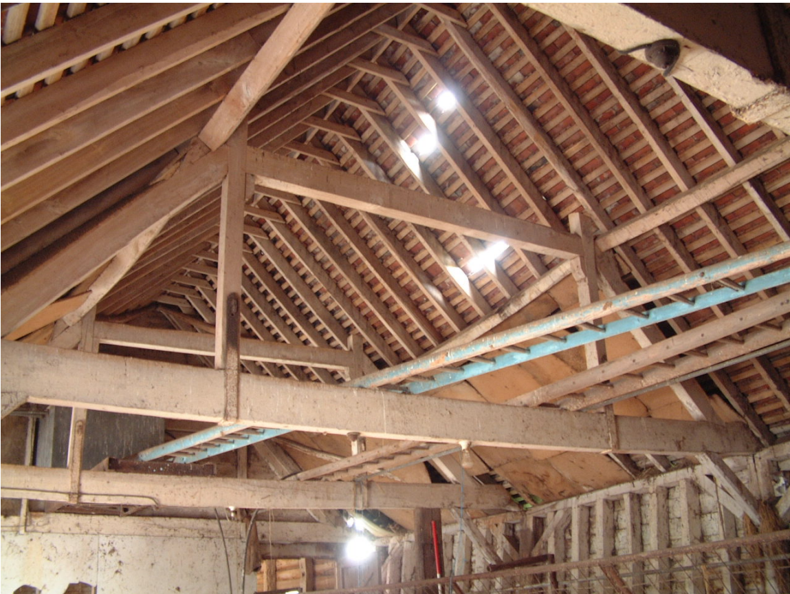
Plate 12: Truss style in shelter shed
