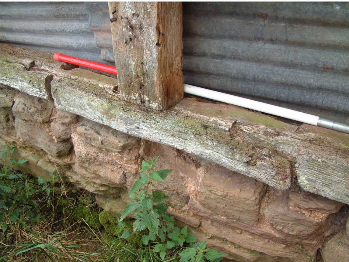
Plate 6: Scarfed in sill section and inserted post; reverse side of Plate 5 (scale 1-metre)
