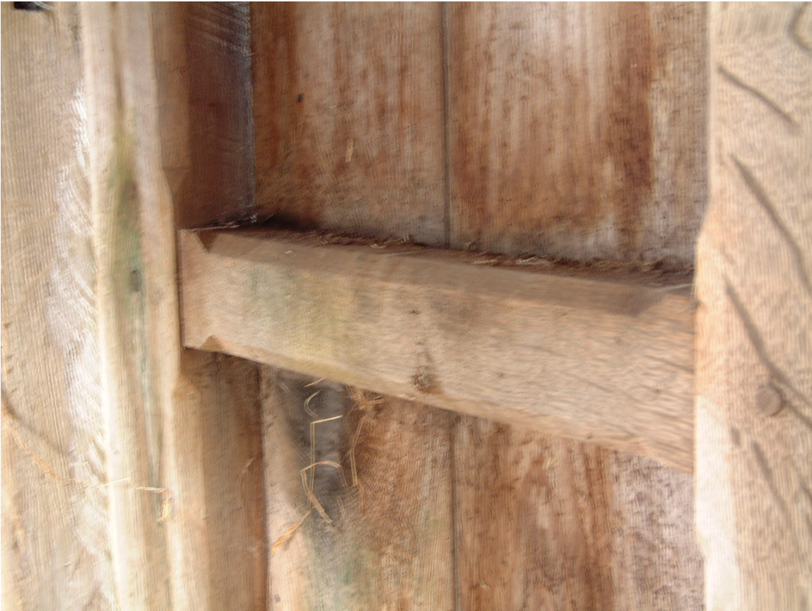
Plate 11: Northern cart door framing; style is similar to that used in shelter shed framing (see Plate 13)
