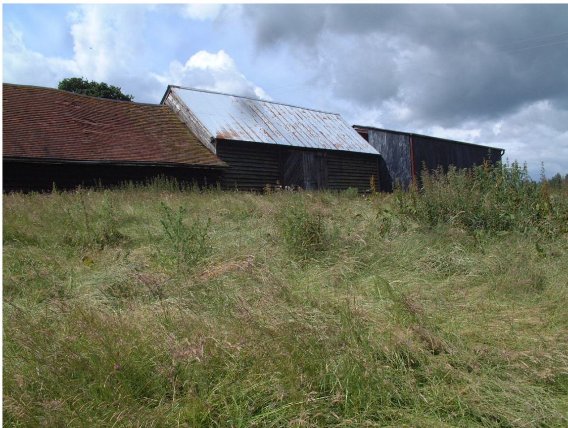
Plate 2: View to the south-west
