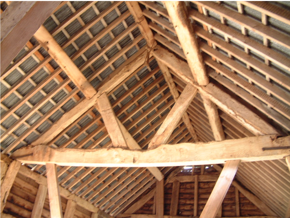
Plate 8: Truss T2 looking west
