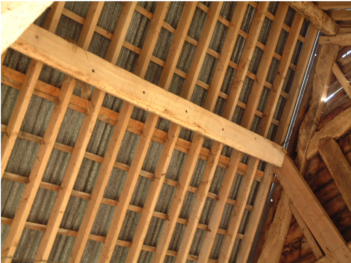
Plate 10: Purlin in bay 1 south roof frame with empty rafter peg holes
