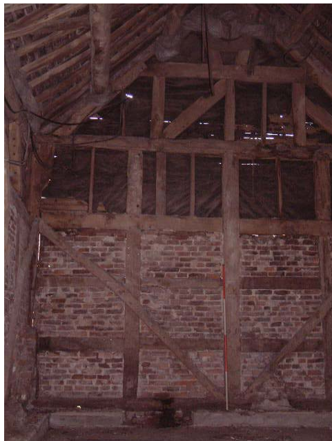
Truss T1 and tension braces (scale 2 metres)
