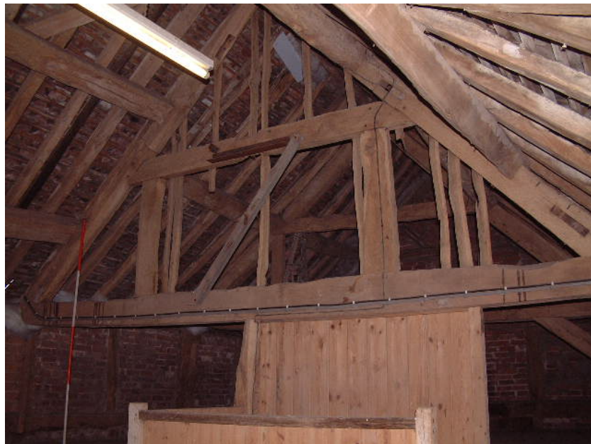
Truss T4 looking into the attached building (scale 2 metres)
