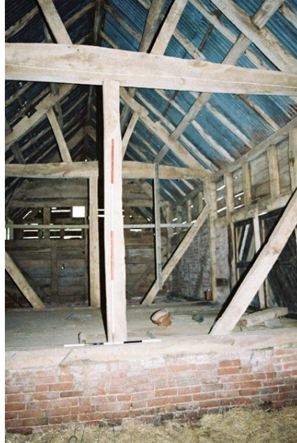
Frames across the threshing bay of a barn at Eastham, Worcestershire, indicating how the frame would have been in the subject barn (scale 2 metres)
