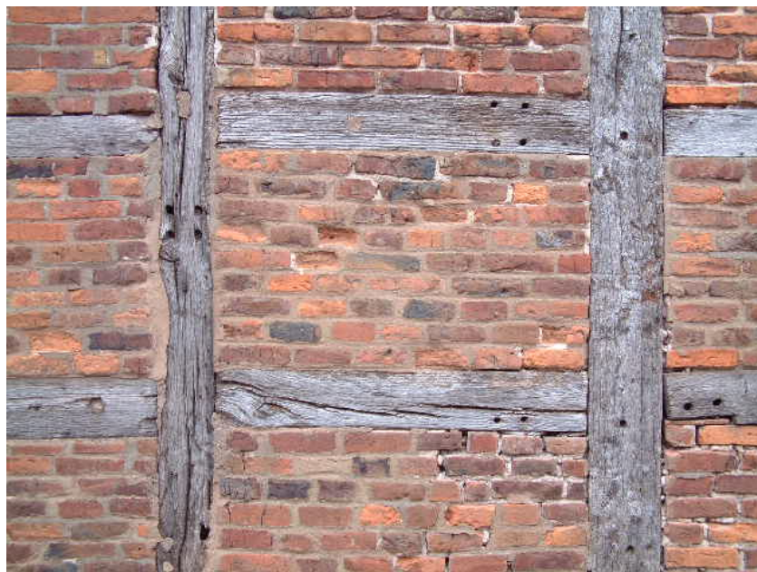
Empty mortises and peg holes in the eastern gable framework
