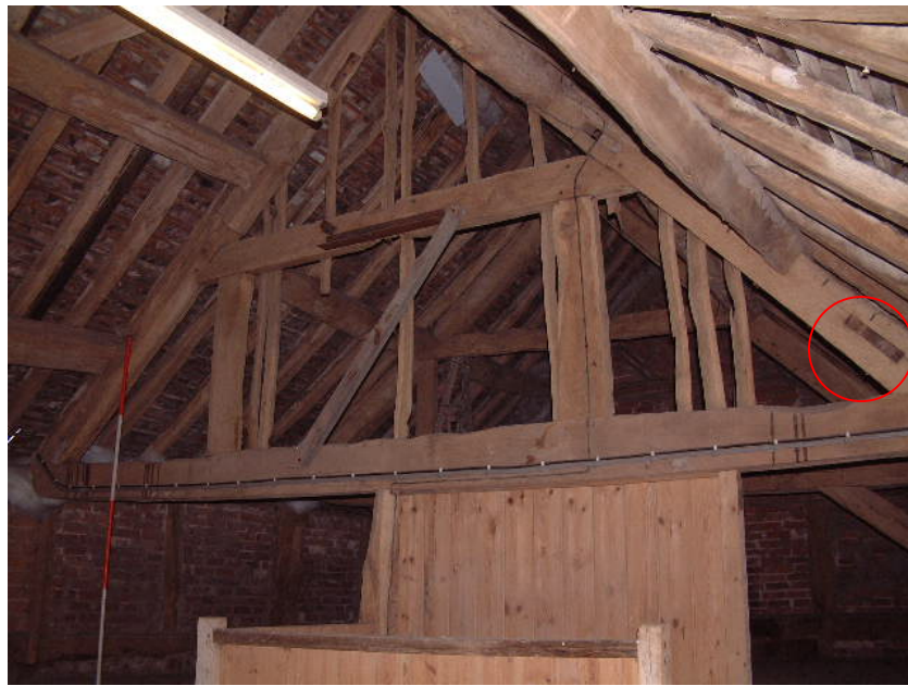
Empty mortise for wind-brace
