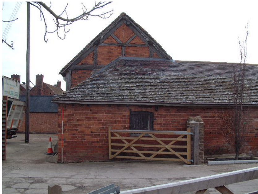
Western elevation frame of the attached (chop house) building (scale 2 metres)
