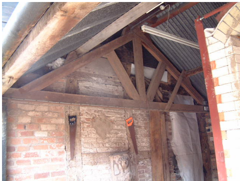
Re-used 19 th century roof truss in the store building
