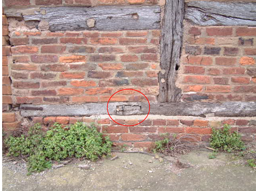
The sawn off tenon in the mortise in the eastern sole plate
