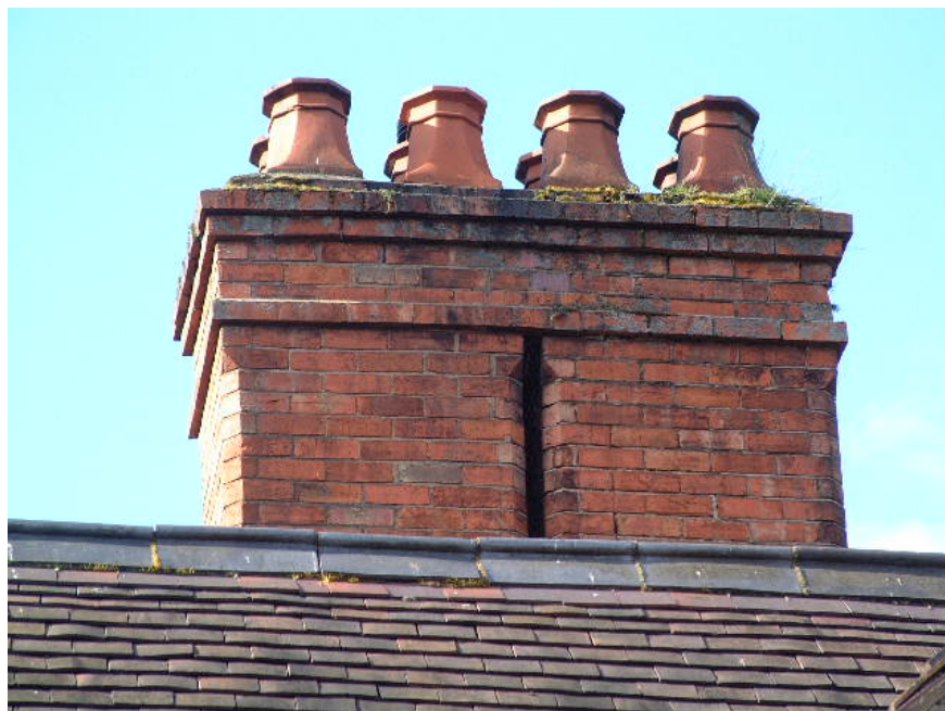
Central eight-flue chimneystack topped with Halifax style pots
