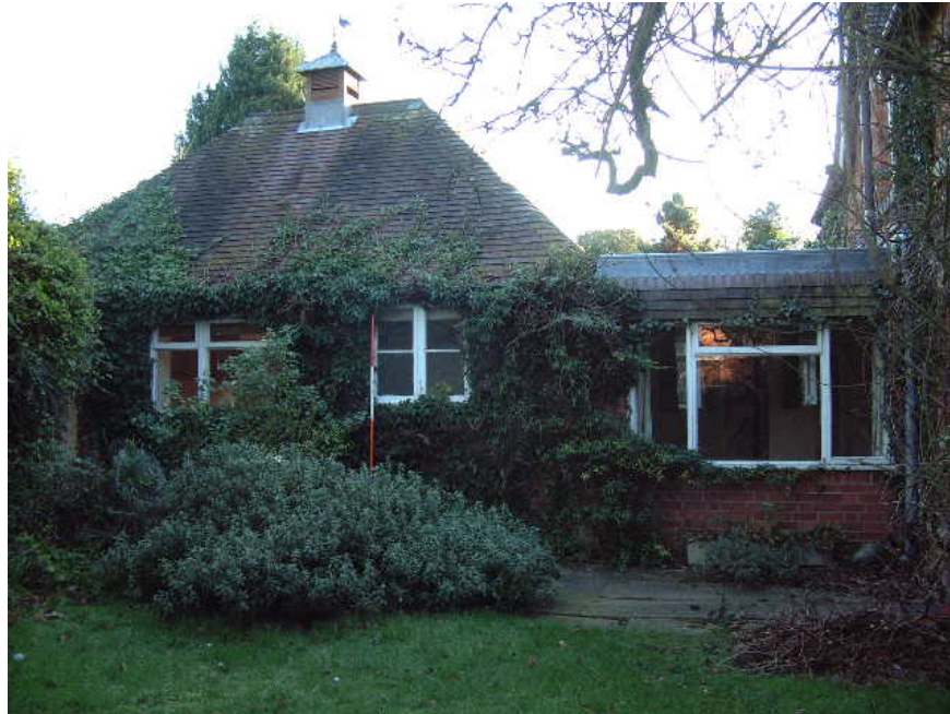
The former outbuilding (right) now connected to the house by a flat roofed extension (scale 2 metres)
