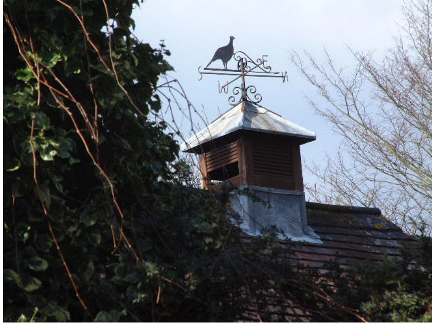
The pheasant weathervane and central roof turret on the former outbuildings
