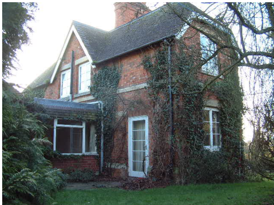
The Building viewed to the south-east (scale 2 metres)
