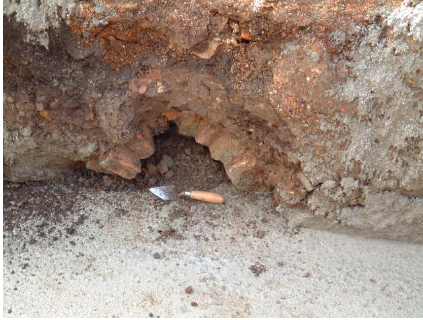
North-south brick arch drain seen at the southern end of the site
