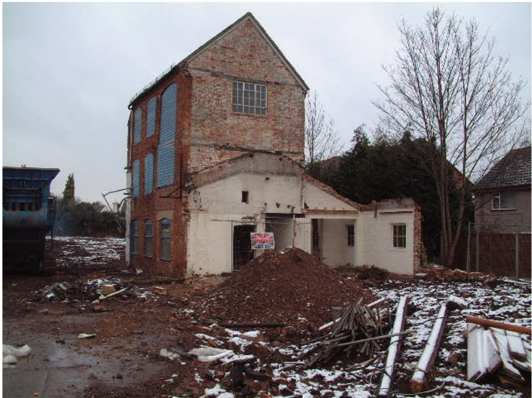
The Button Factory during demolition; view to the north-east
