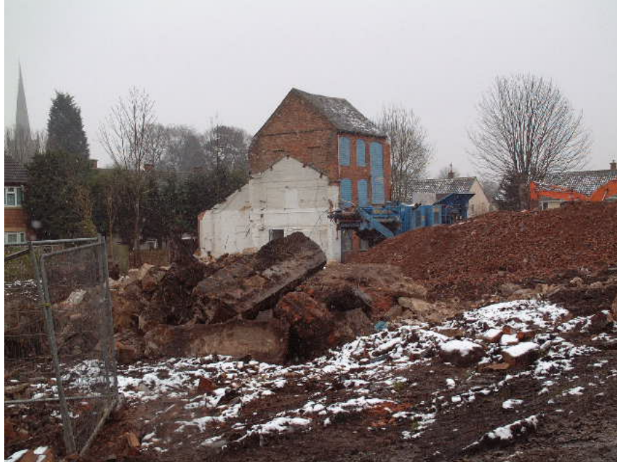
The Button Factory during demolition viewed to the south-east
