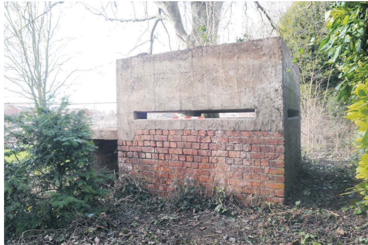
Eastern elevation (Scale 0.5m long)
