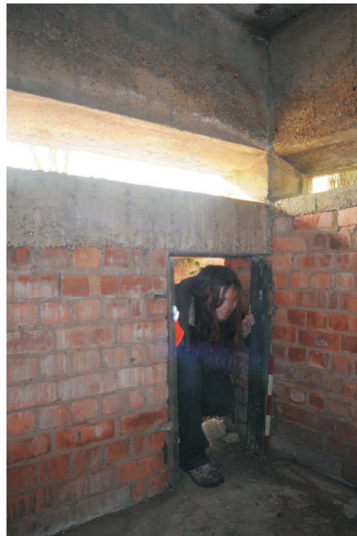
Internal view of doorway
