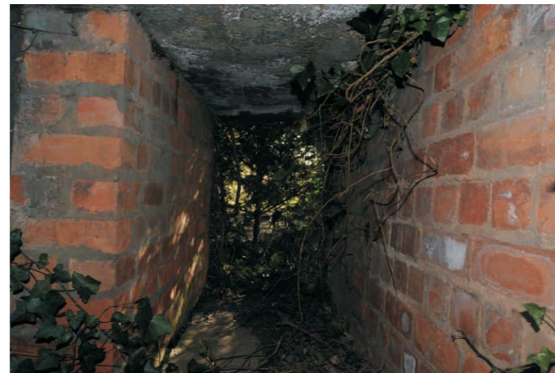
Entrance crawlway prior to clearance
