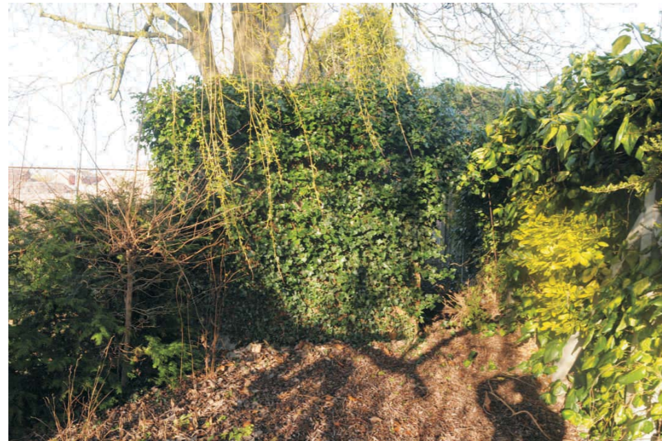
East elevation prior to removal of ivy and undergrowth
