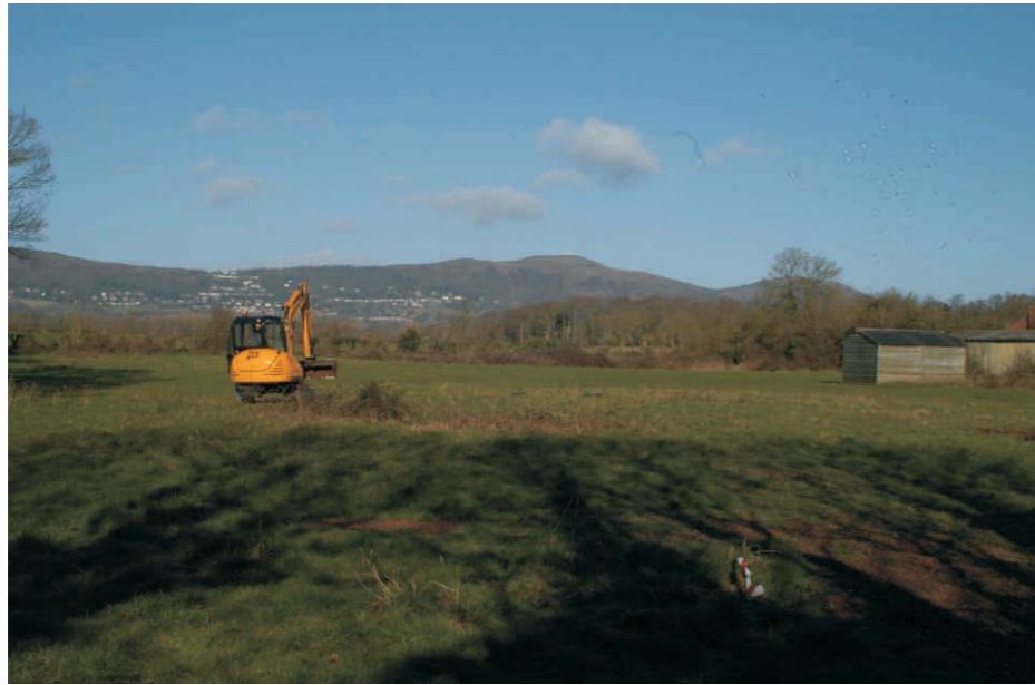
General view of site prior to trenching (facing north-west)
