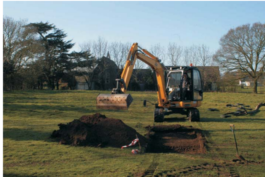
Machining Trench 3 (facing south)
