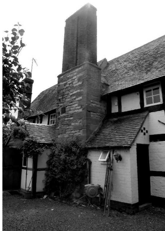
17th C Chimney stack on eastern elevation
