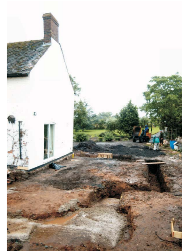
Area of new extension facing south
