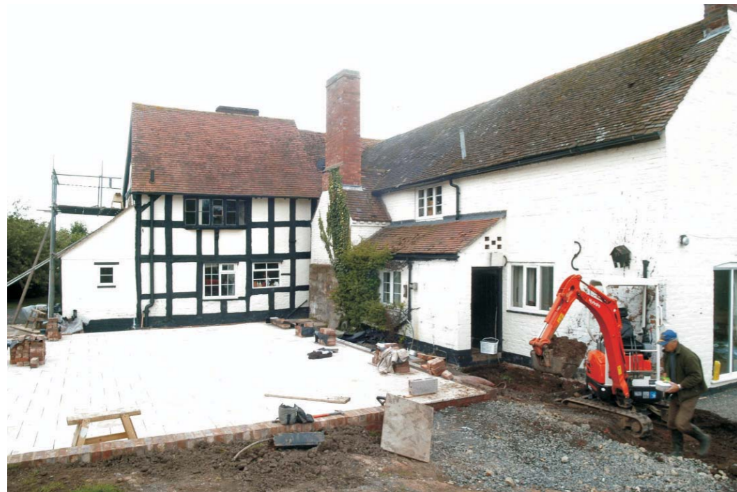
Rear elevations, and newly paved area
