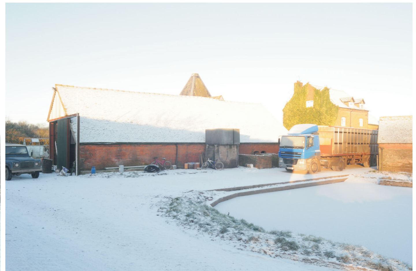
View of granary range from the east (farmhouse and pond visible to right)
