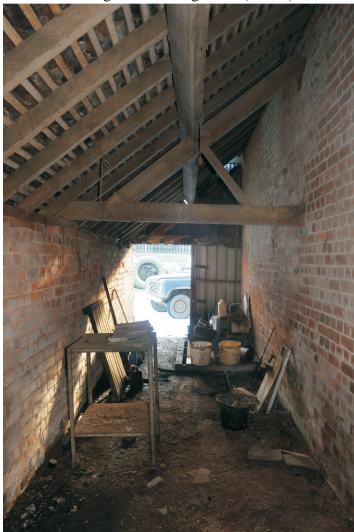
Interior of “long store” facing south (below) and north - note inserted block wall of spray/chemical store
