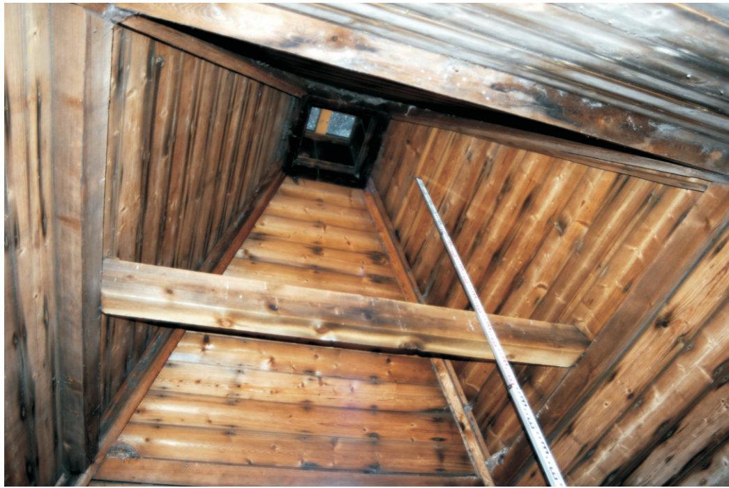
Apex of roof
