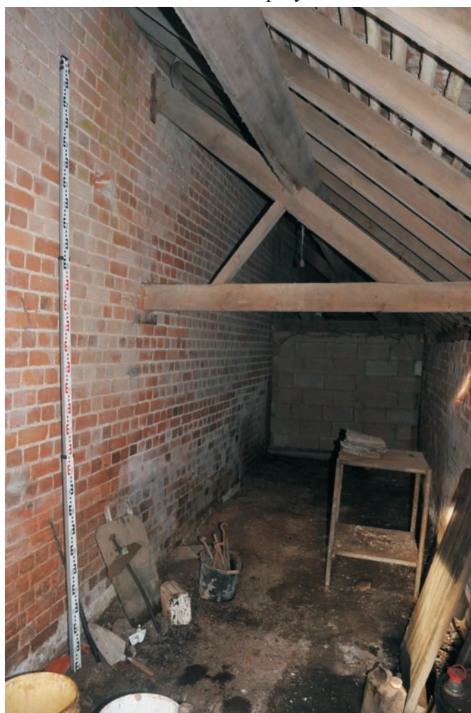
Interior of “long store” facing south (below) and north - note inserted block wall of spray/chemical store
