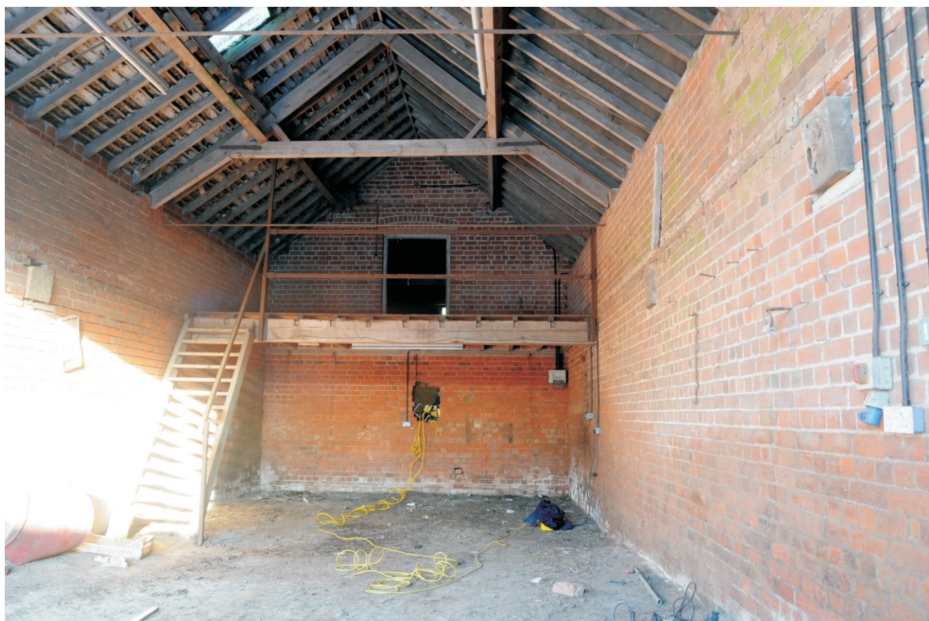
“Granary” facing north - note truncated former upper floor bridging beams
