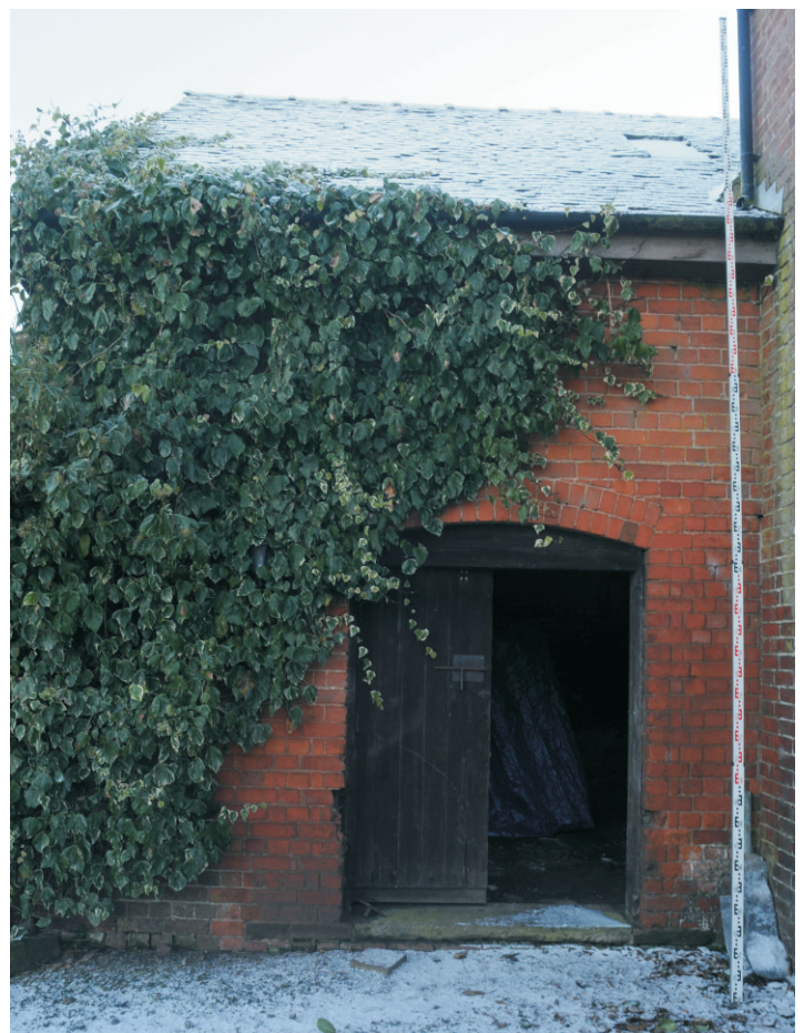
Northern end of Western elevation
