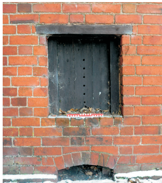
Northern elevation of hop kiln with detail of vent and flue (above)
