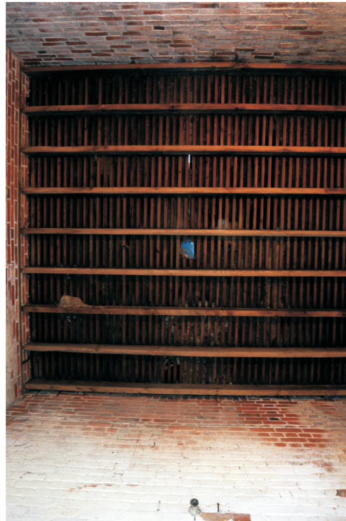
Underside of drying floor
