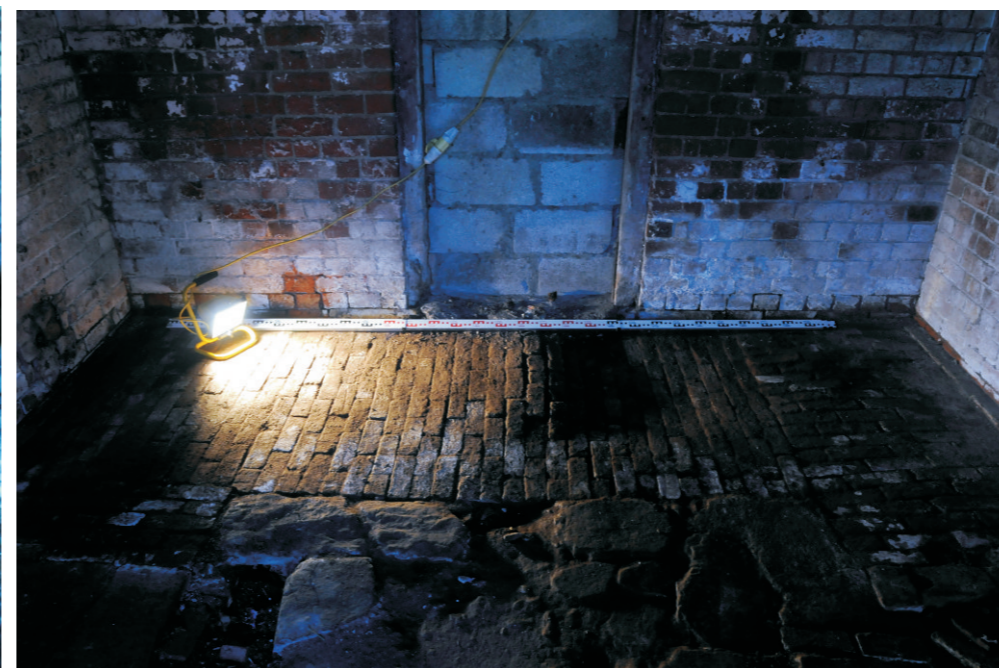
Kiln floor facing east, showing subsidence in front of doorway, probably over a flue
