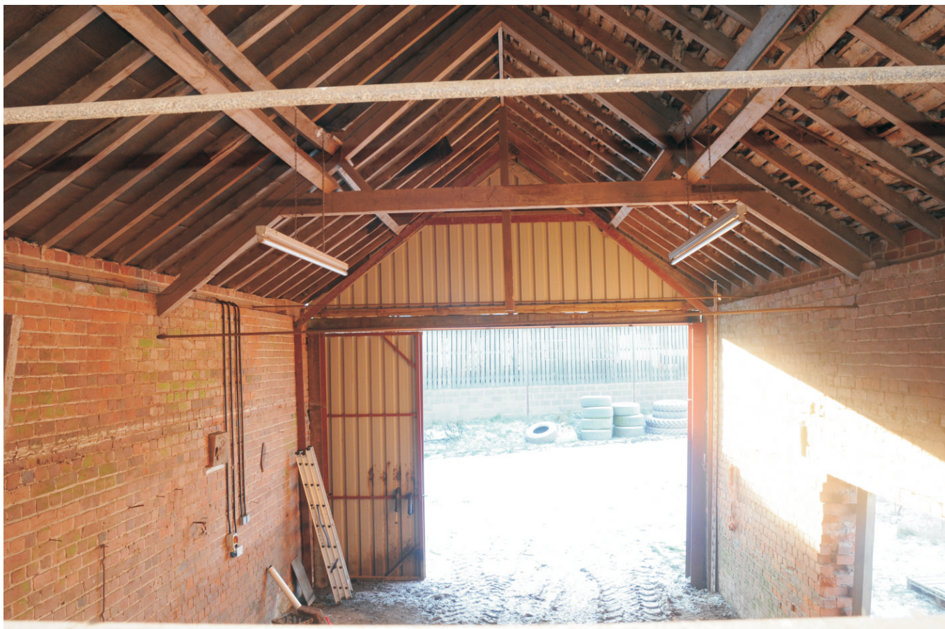
“Granary” facing south - note white line marking former upper floor level
