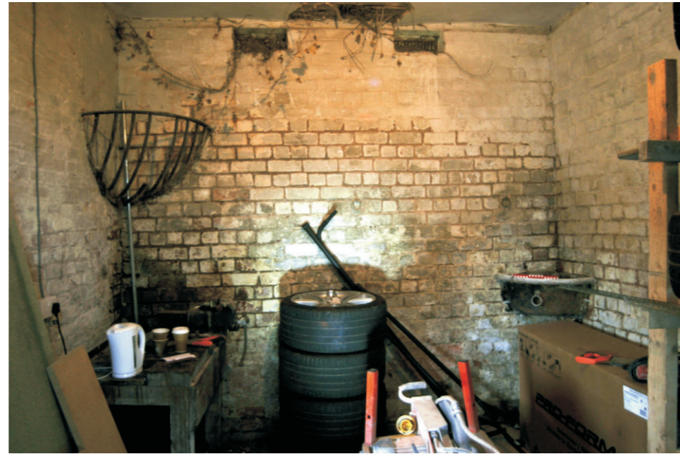
South-western end of stable, note hayrack and level vents
