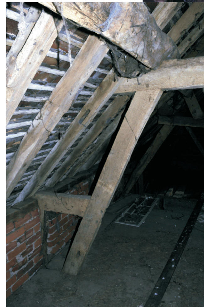
Detail of open truss principal
