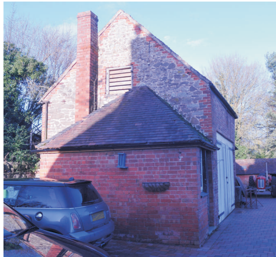
View from SE showing tack room extension
