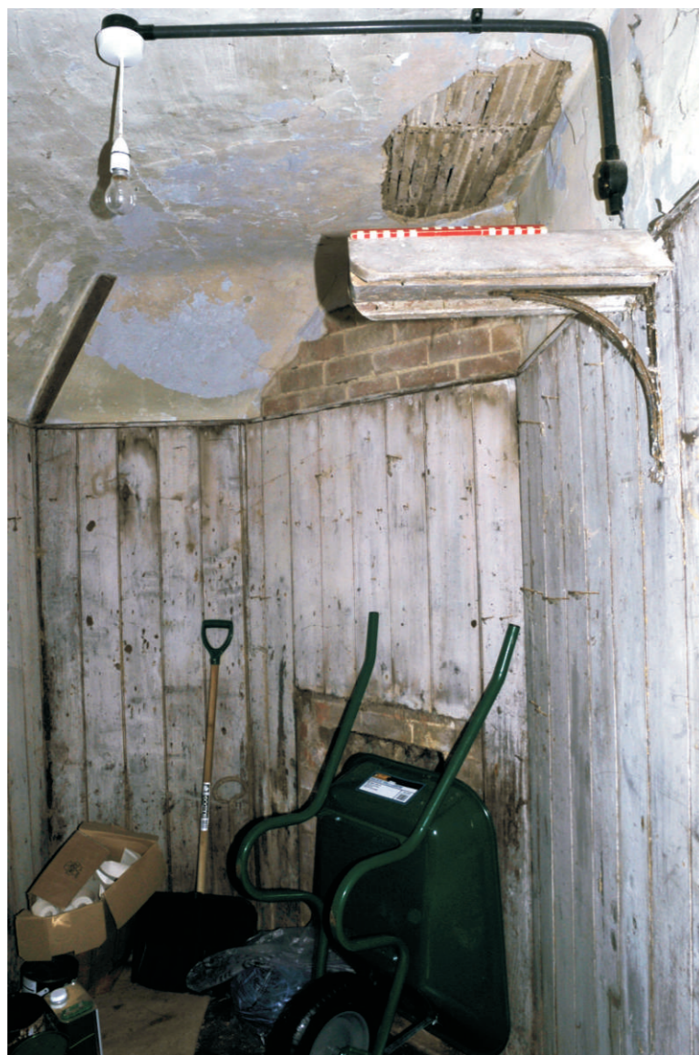
Above and below - Tack-room -note saddle bracket and fireplace
