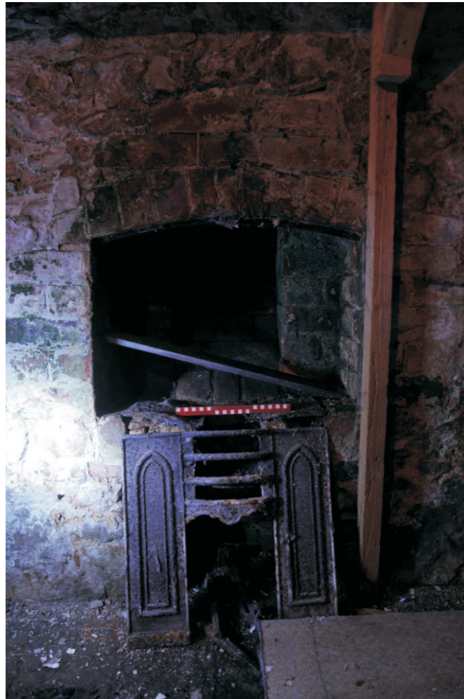
Detail of small hob-grate in coach-house
