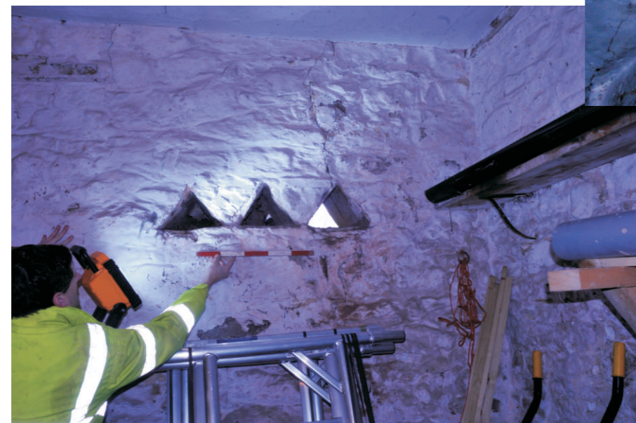
Detail of triangular vents
