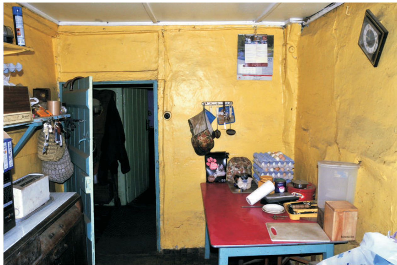
"Larder" now used as kitchen, view facing west
