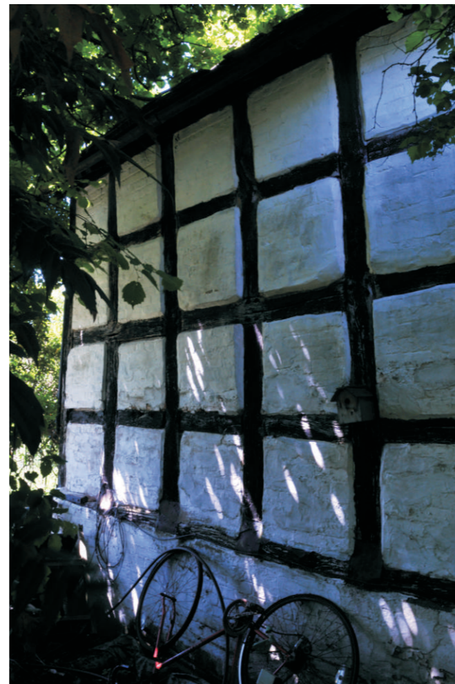
Western end of southern elevation; cellar access concealed beneath bicycle
