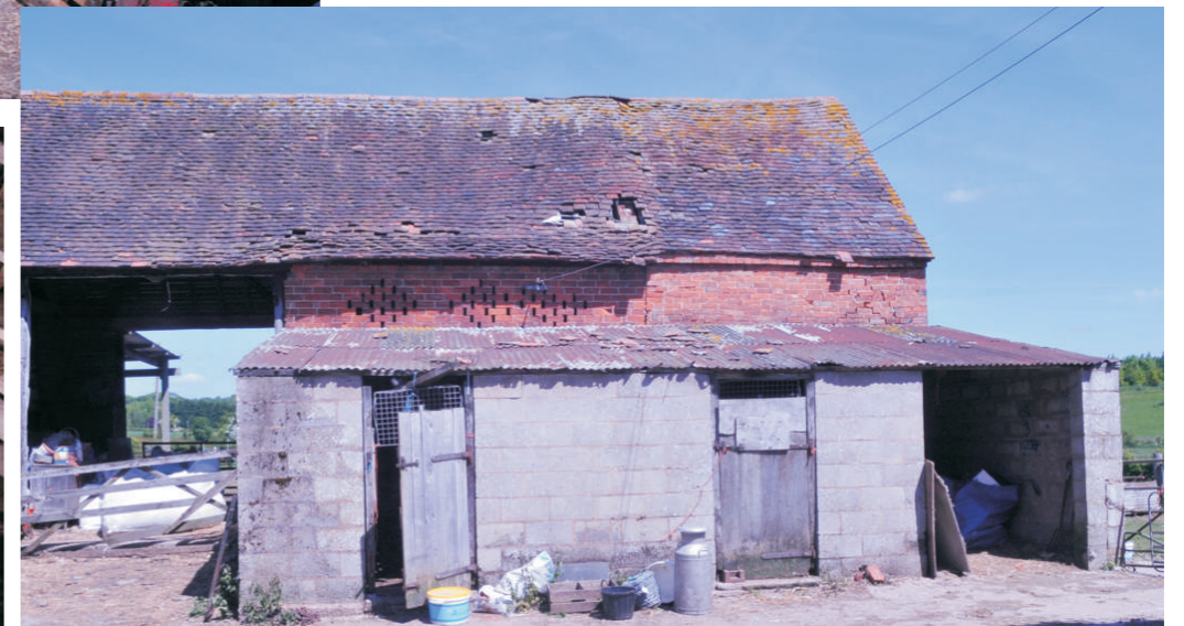
Concrete block built poultry house, note break in construction between barn (to rear) and the brick built bay to the right, which appears to be the earlier structure
