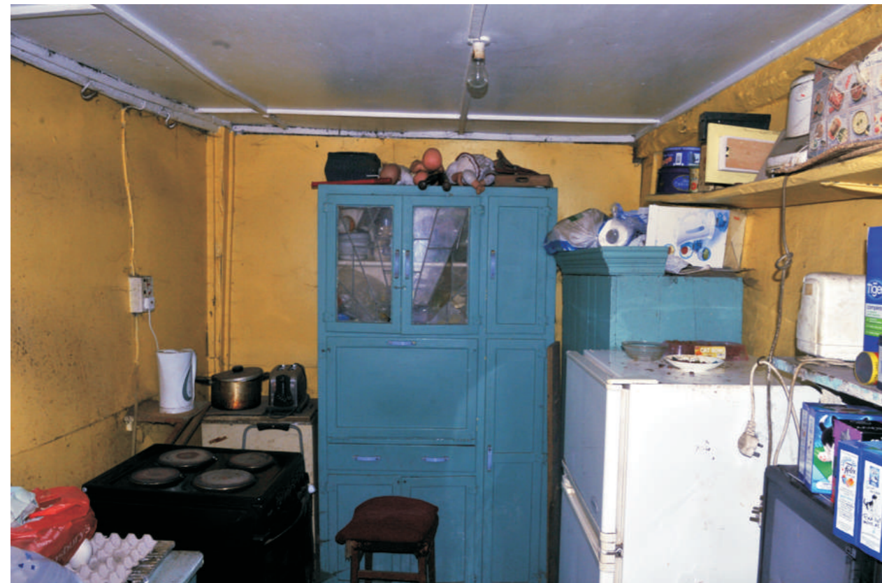
View facing east, note hardboard lining over framing and concealing ceiling
