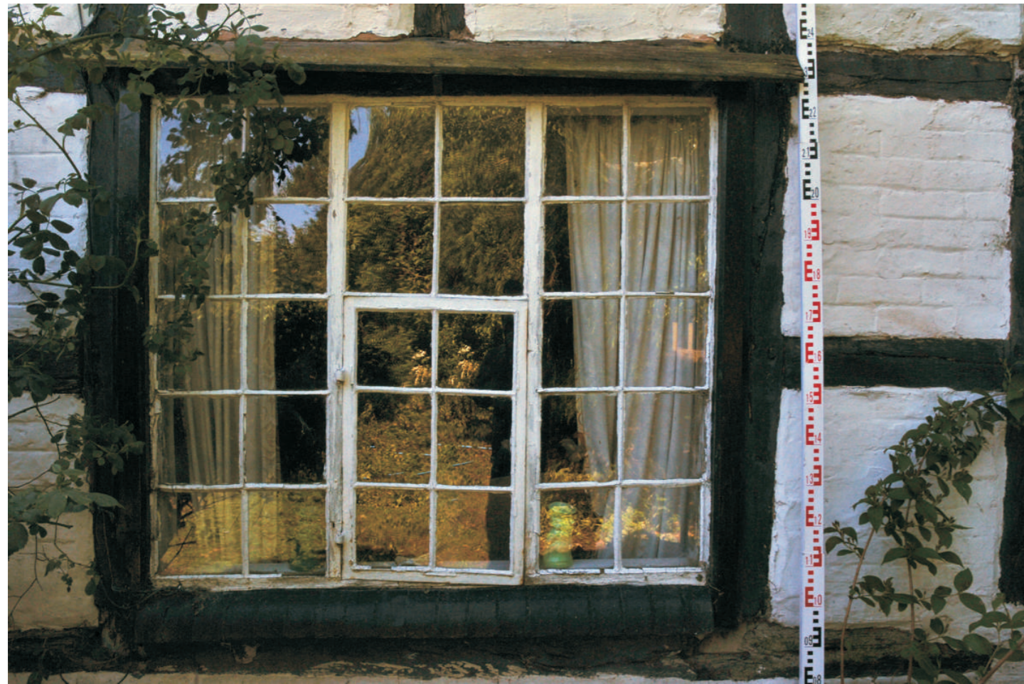
Metal framed window to western bay - this type of window is not closely datable, but probably early-mid 19th C, retaining its highly refractive hand made glass - note the quality of reflection
