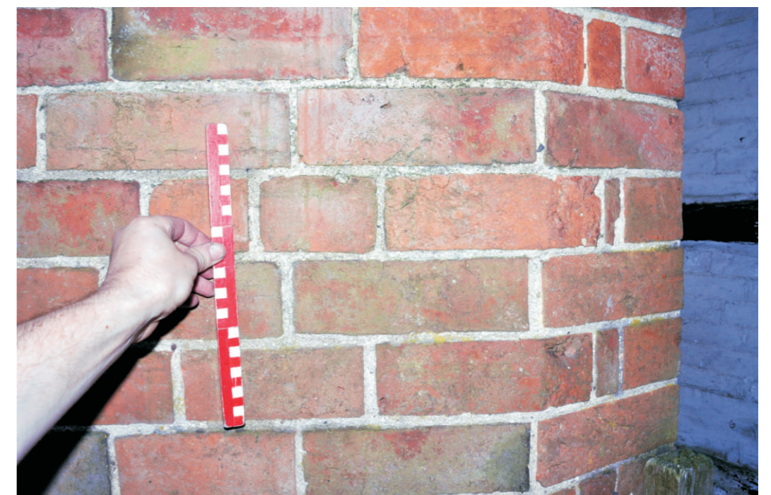
Brickwork detail, north wall of pigsty
