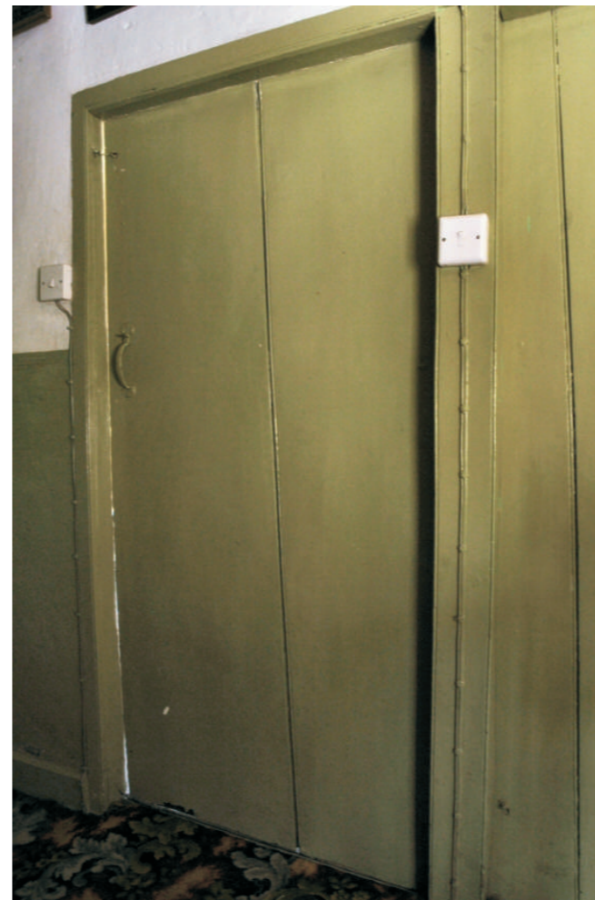
Two plank ledged door to bathroom
