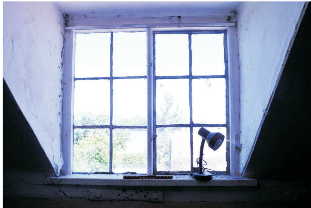
Detail of dormer interior, eastern bay
