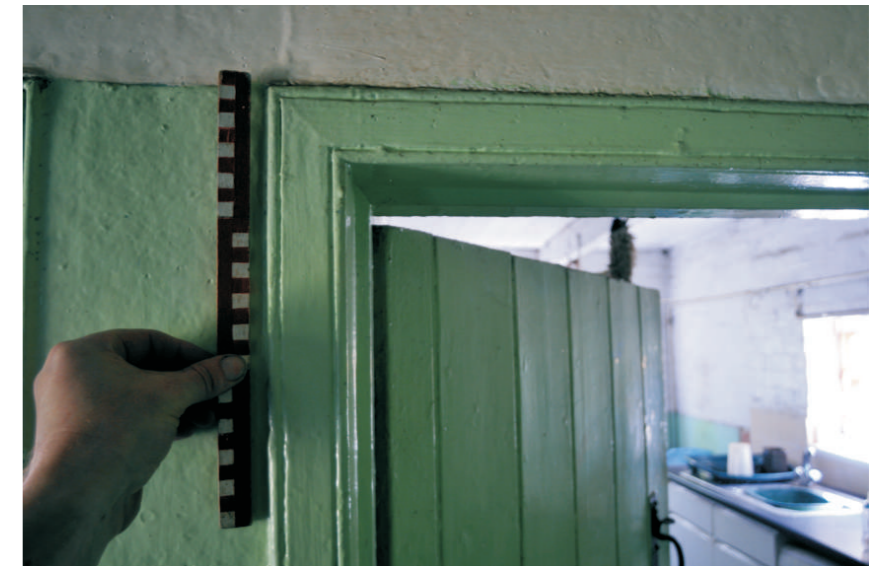
Detail of architrave, scullery door
