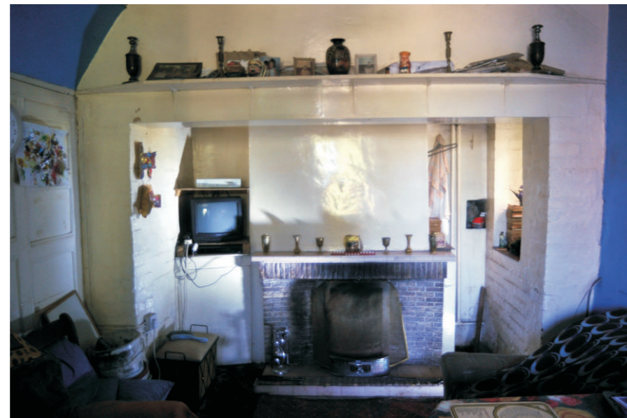
Modified inglenook fireplace in central bay (former kitchen)
