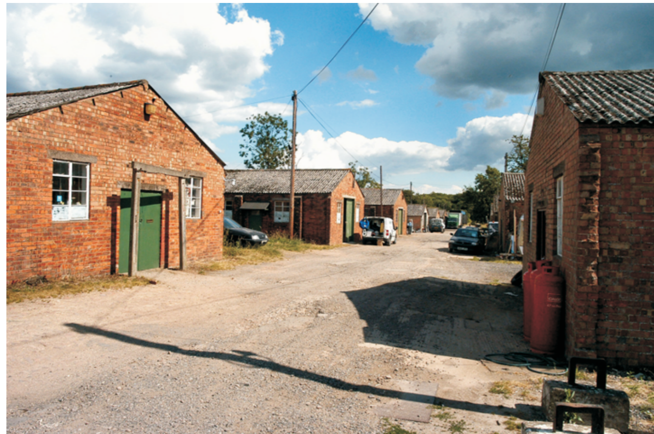
2005 "Walkway 1" between surgical wards view facing south-east
