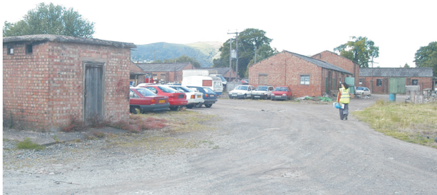
2005 - view from northern corner of "X2" facing north-west (boiler house "X4") is the taller block beyond figure
