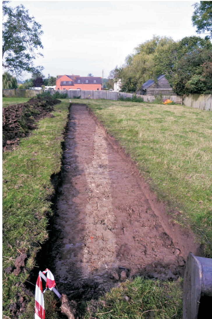
Trench 1 view facing west (note watermain trench) and detail of small sondage cut into watermain trench fill (below)
