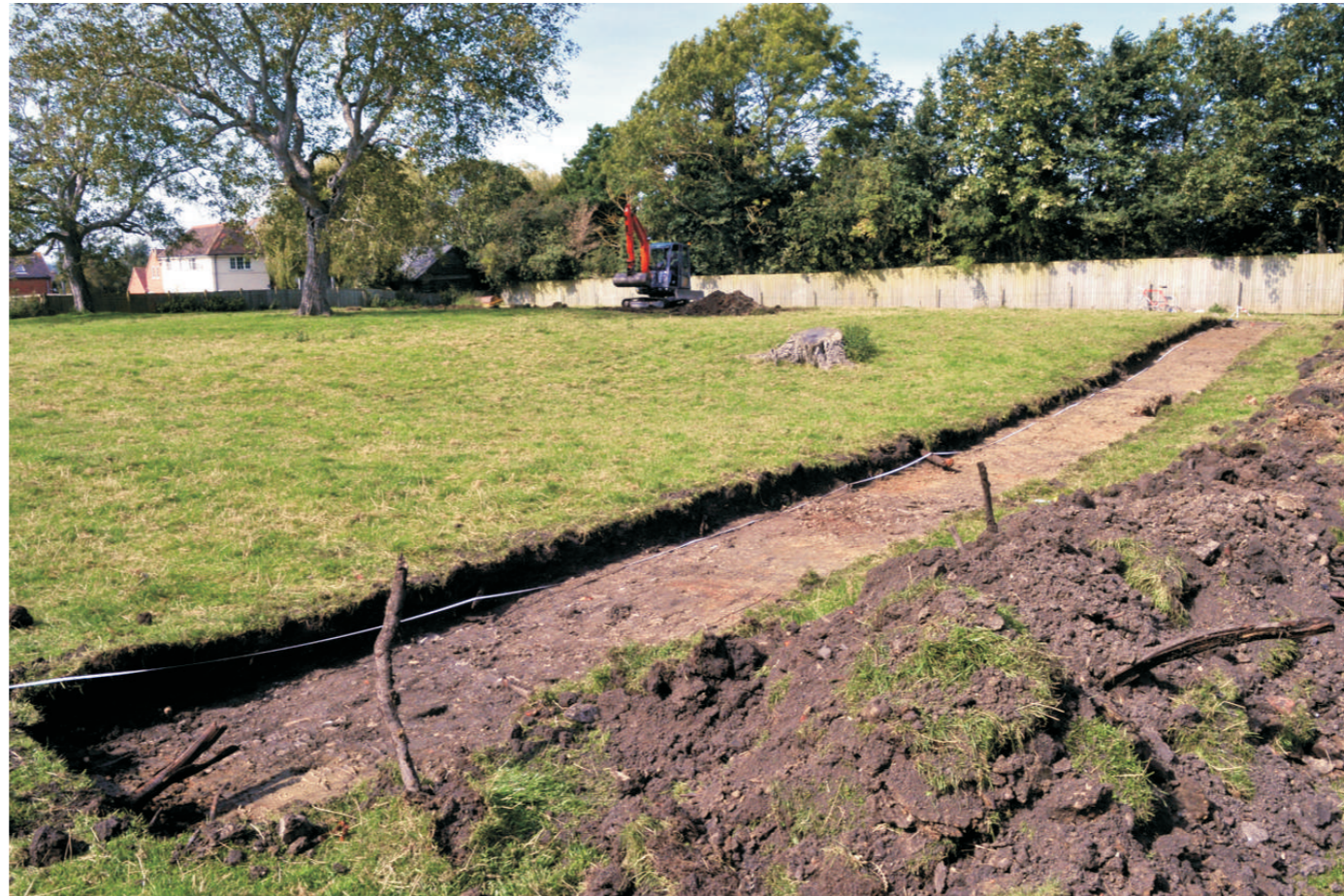
General view of Trench 3 facing north-west
