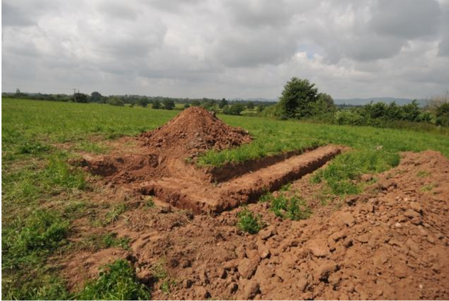
View of trench facing north-west
