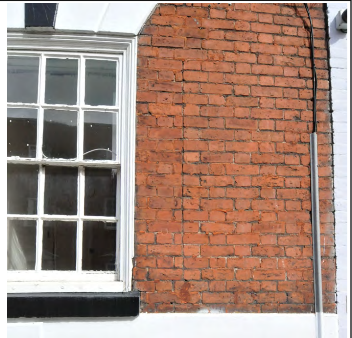
Area of brick infill of former window opening - note vertical joint
