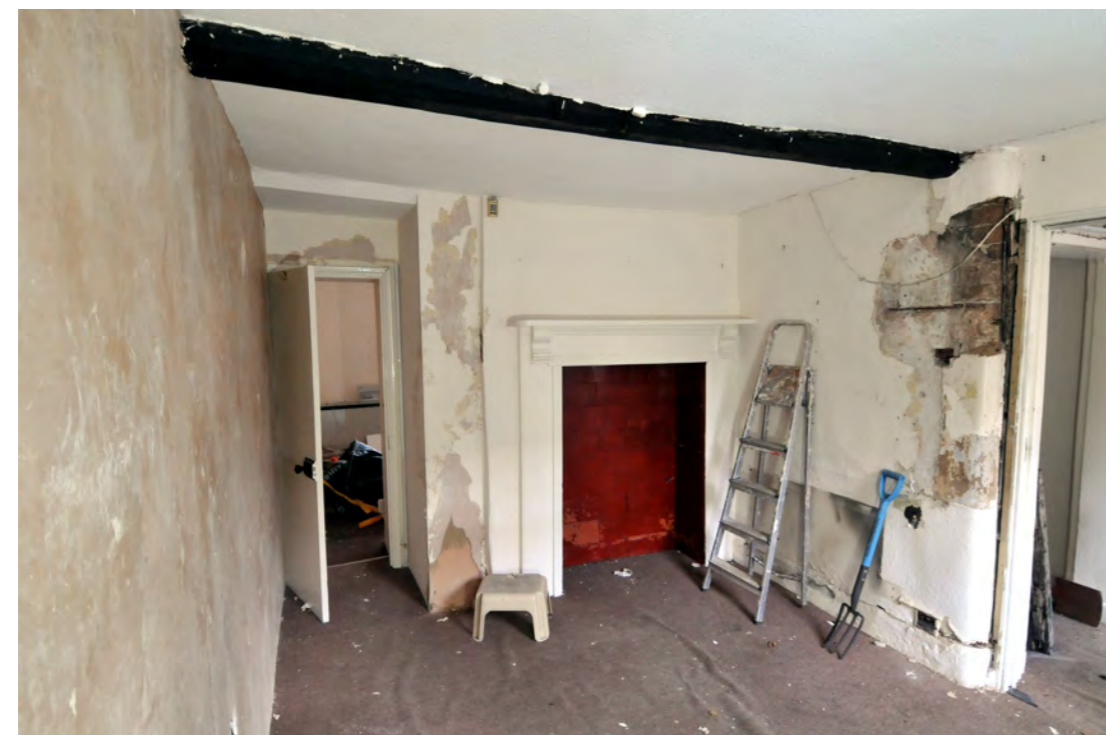
Southern rear room (inserted doorway to front room)
