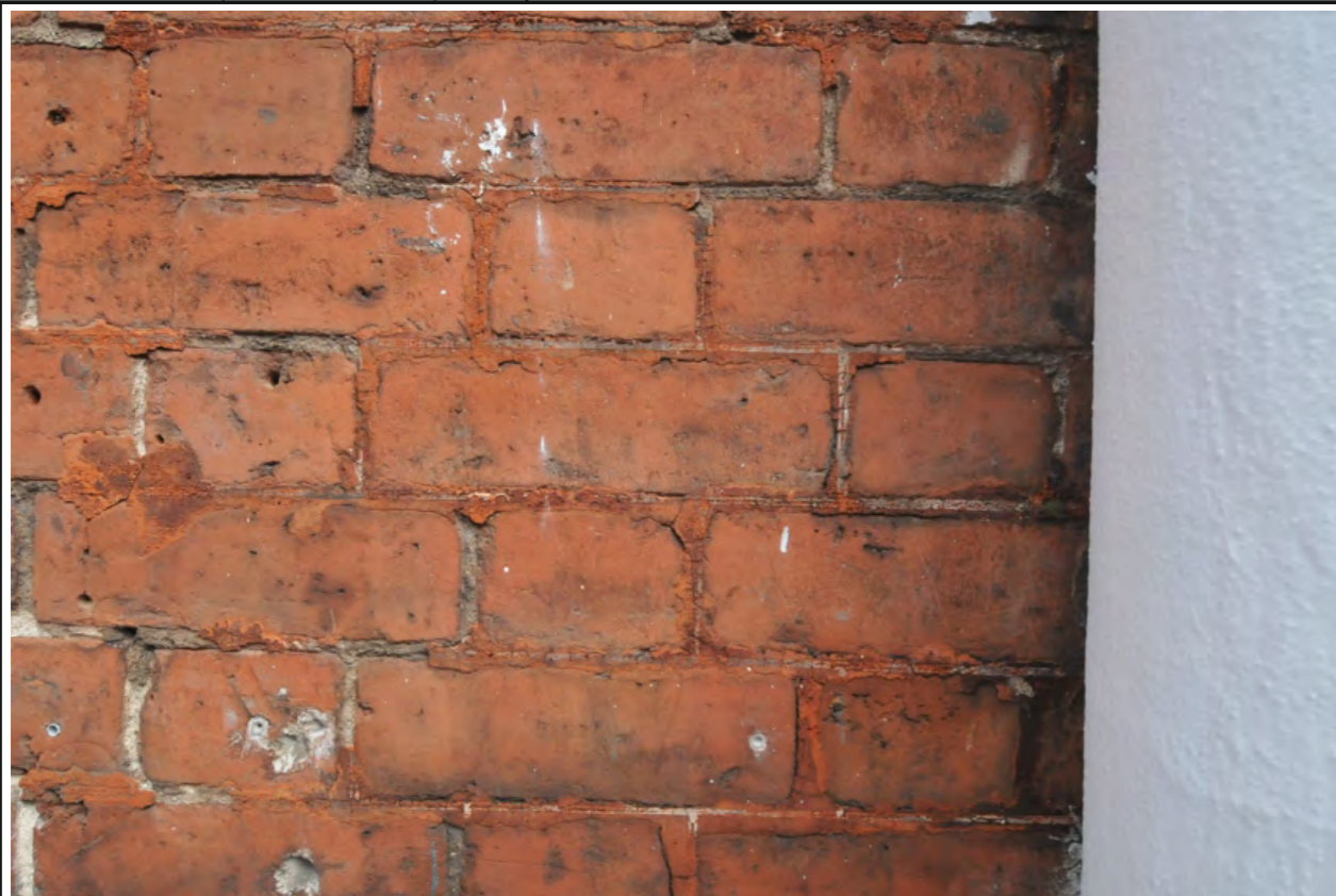
Detail of struck false jointing and brickwork colouring
