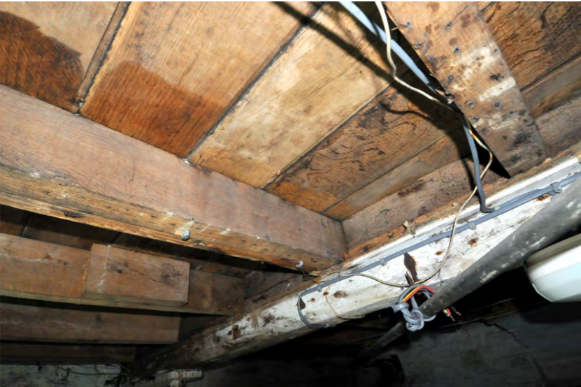
Underside of oak boarding
