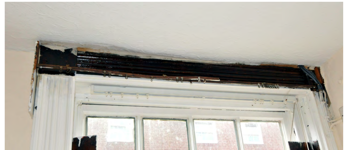
Front southern room window with evidence of former vertical sliding shutter
