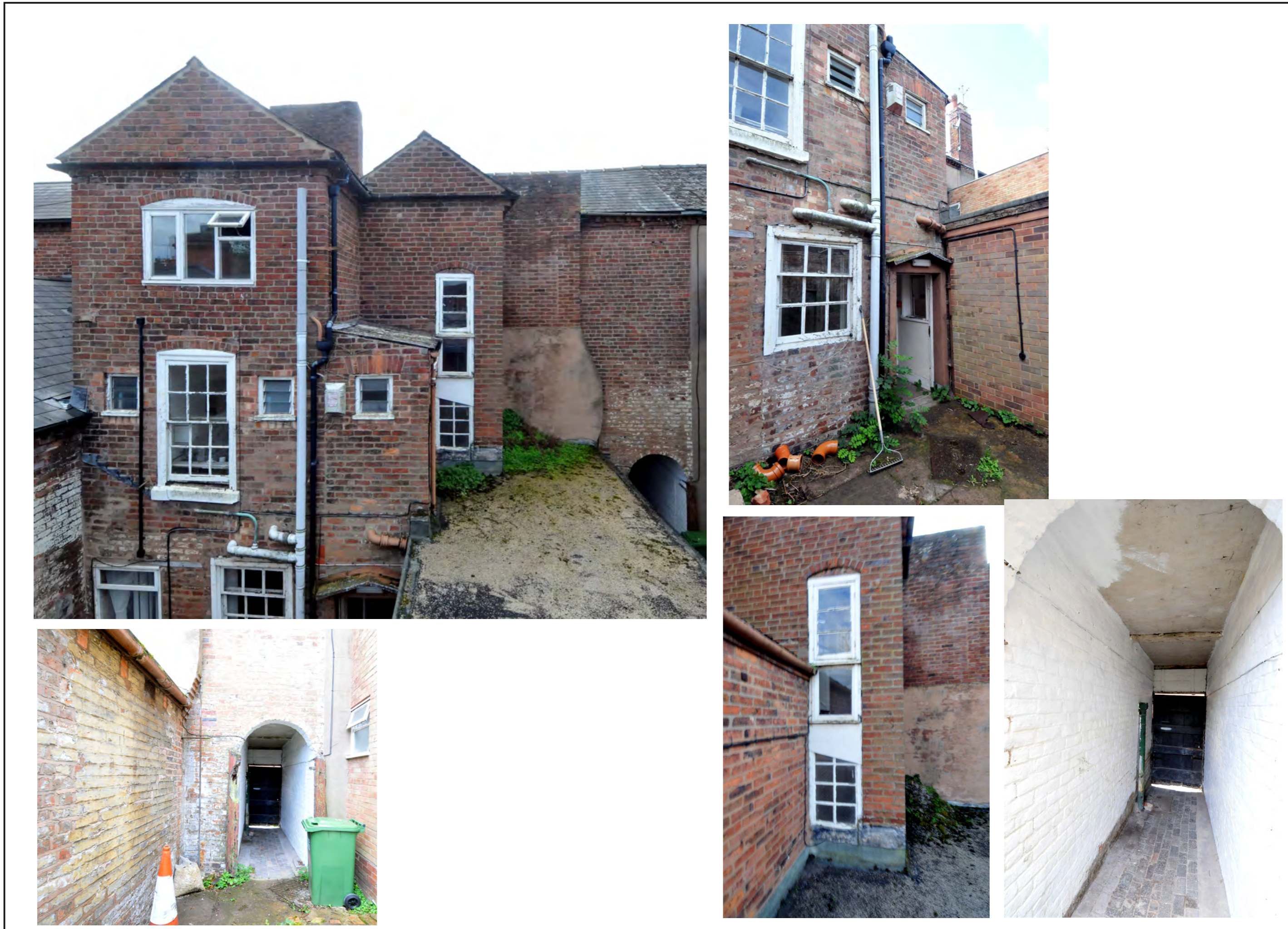
Figure 4: Rear elevation and side passage
