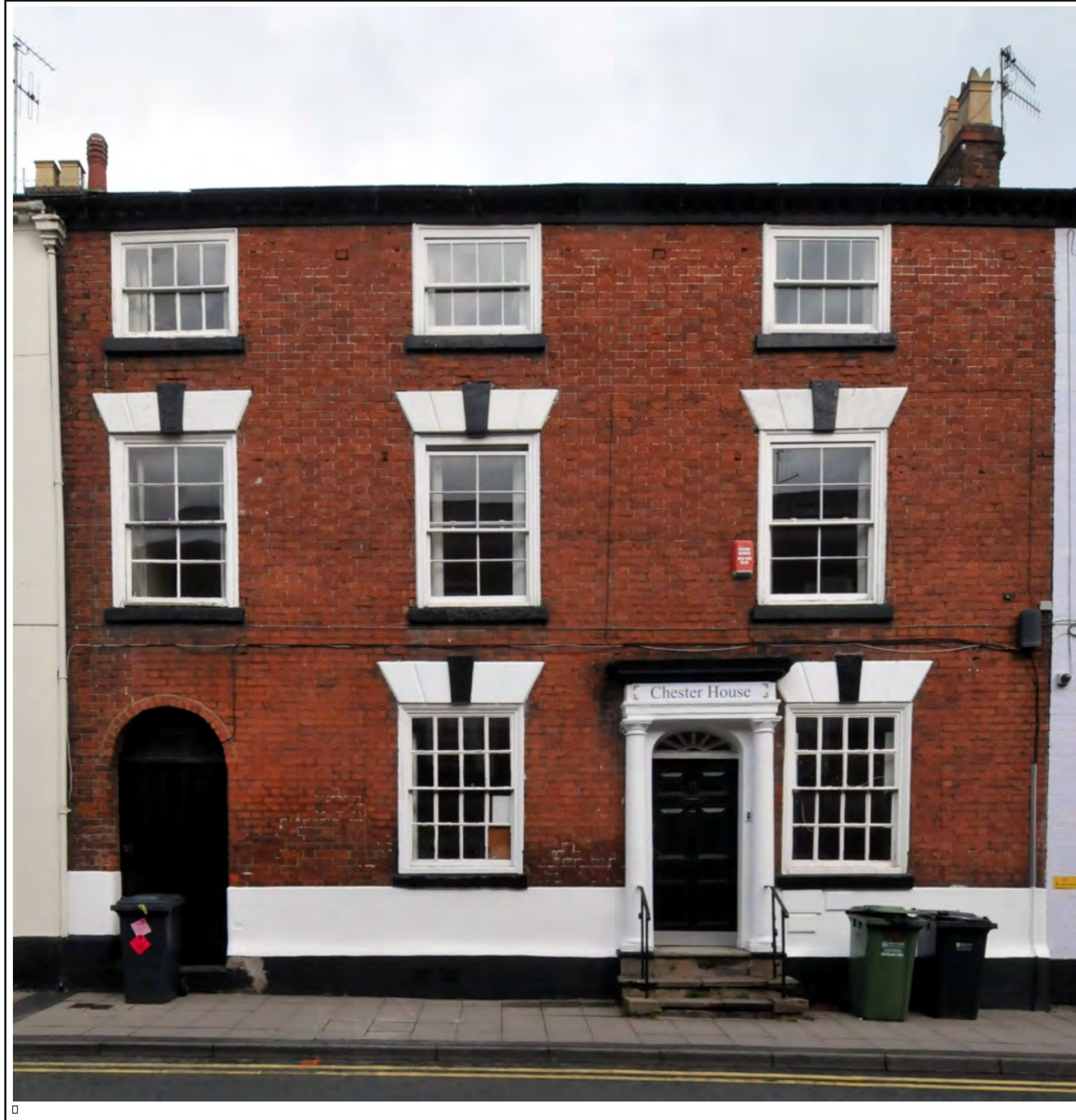
Figure 2: New Street elevation - note imbalanced ground floor fenestration and re-located window openings
