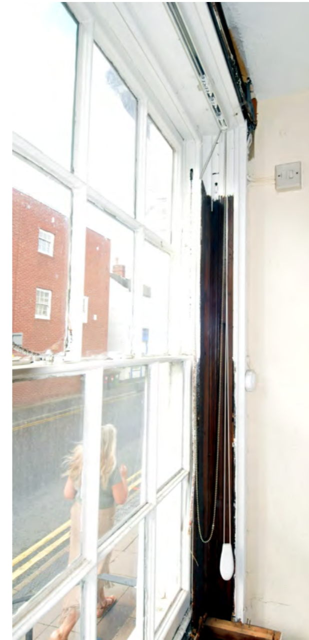
Front southern room window with evidence of former vertical sliding shutter
