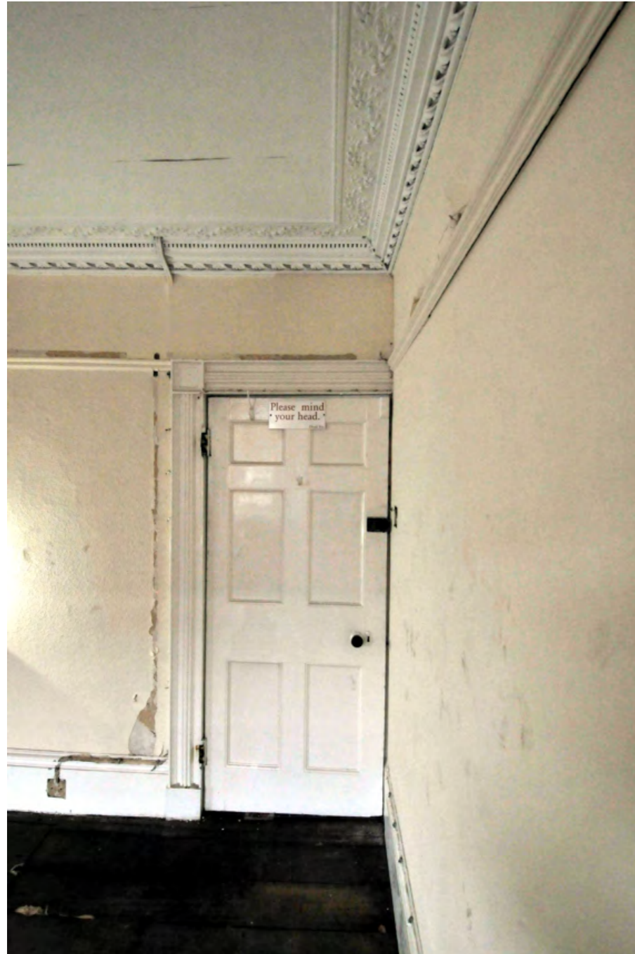
Doorcase detail note scar of removed patera
