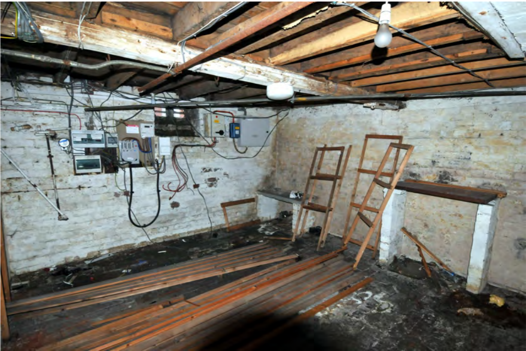
Northern cellar facing north-west
