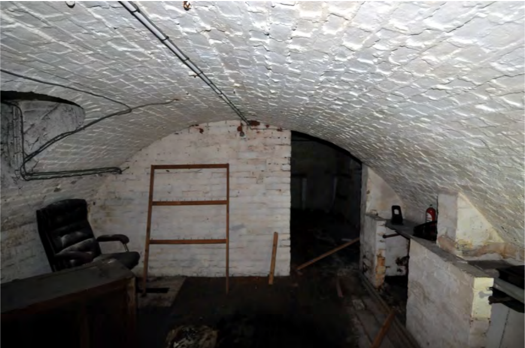
Southern cellar facing north
