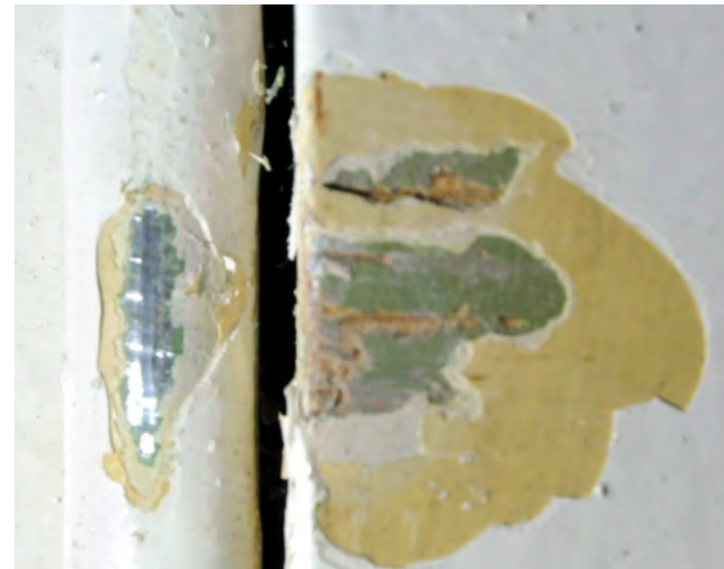
Paint scrape showing original green paint of window-case
