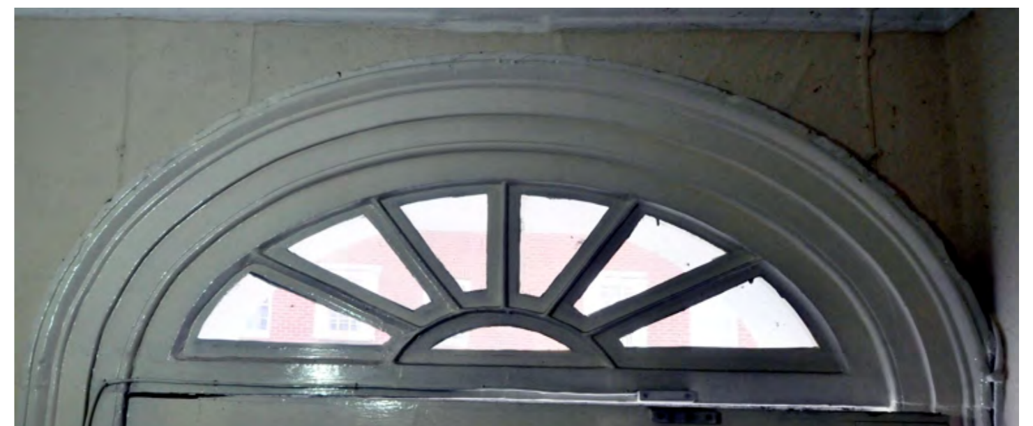
Detail of interior of cast iron fanlight glazing bars
