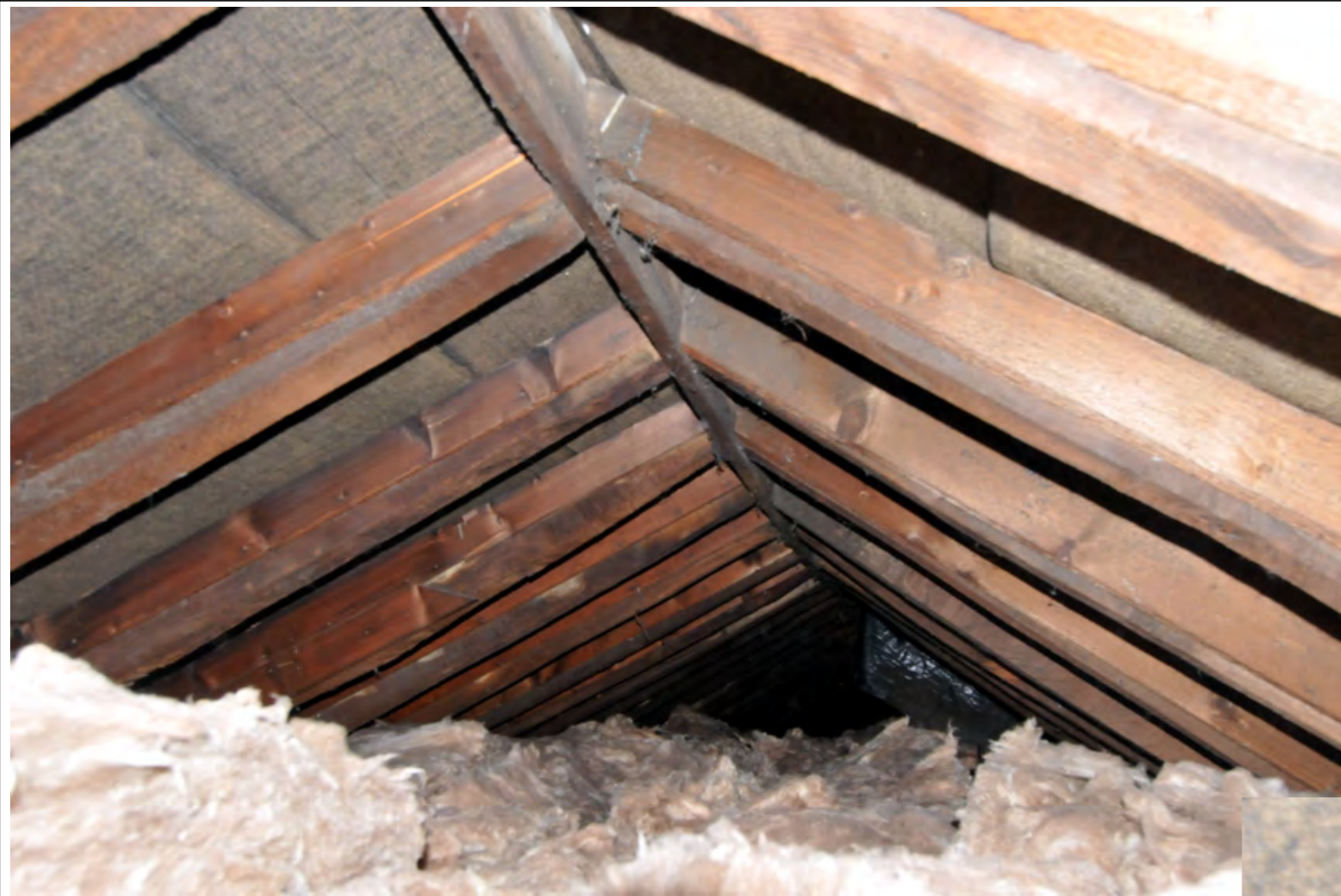
Roof structure (mill sawn paired common rafters on Baltic softwood purlins)
