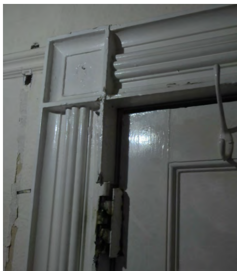
Figure 12: First floor front northern room details - nb the wrought steel panels conceal former recessed lighting
