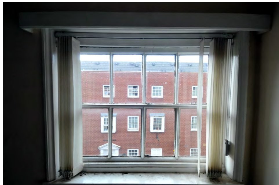
Second floor front (south) window detail
