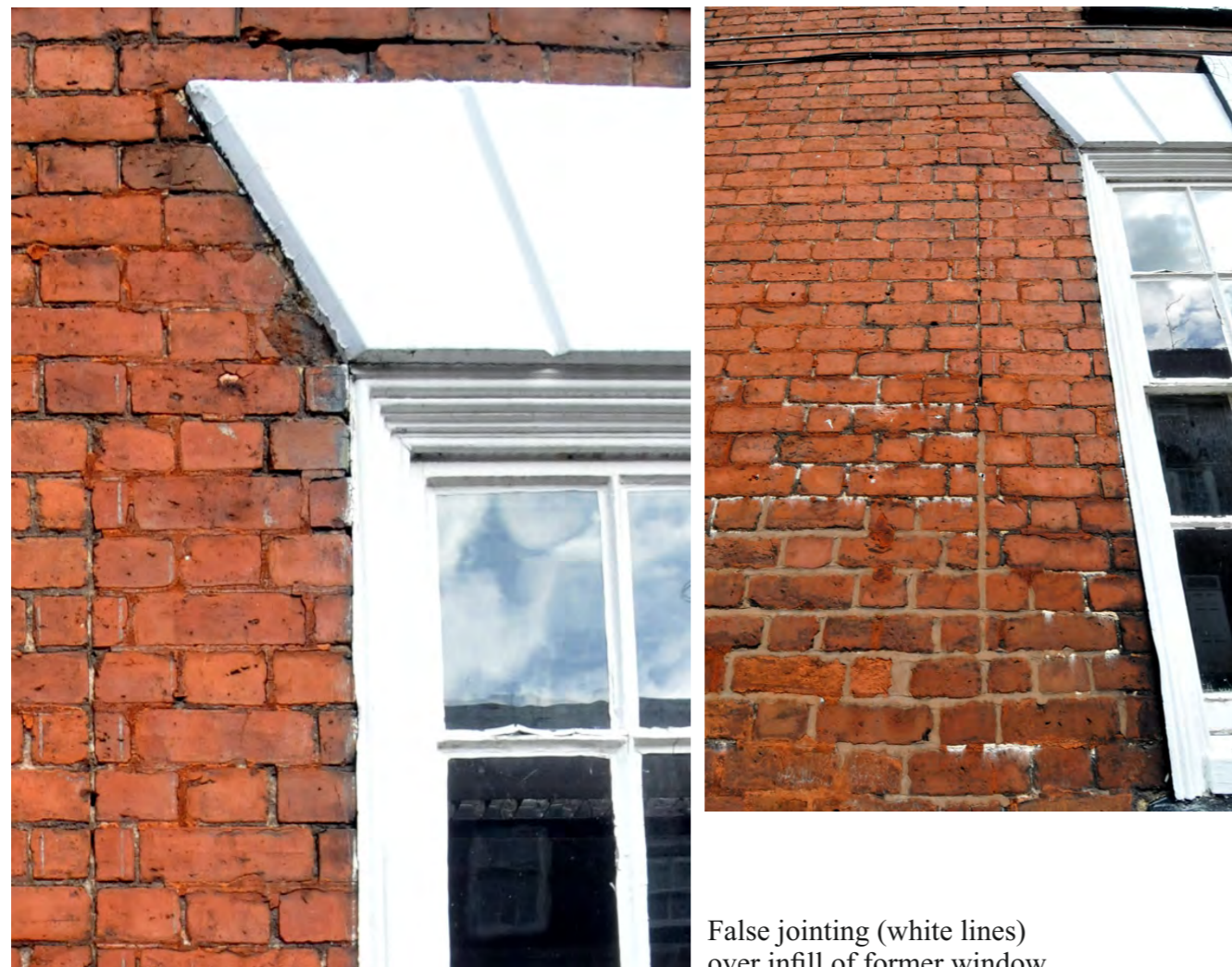
Area of brick infill corresponding to former window position
