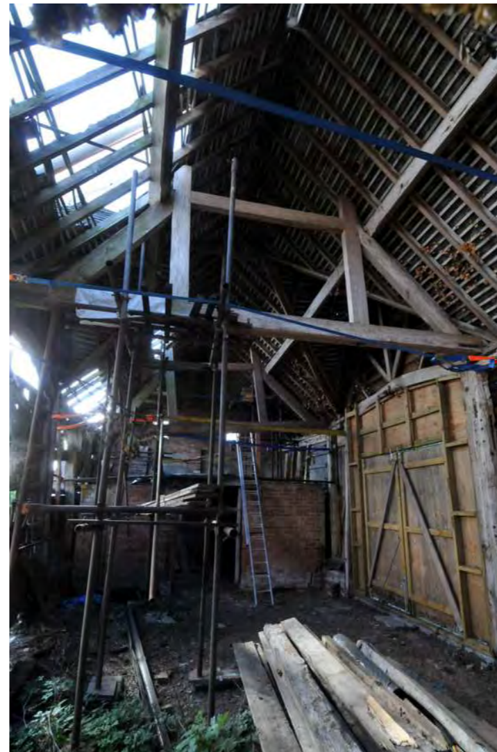
Figure 5: Barn interior - framing includes some re-used elements of a late 17th-early 18th C framed barn but represents a total rebuild with new roof and doorways of circa 1810-30 (Baltic softwood trusses)
