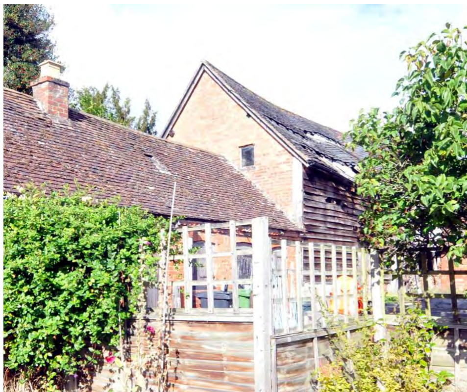
Southern rebuilt gable end
