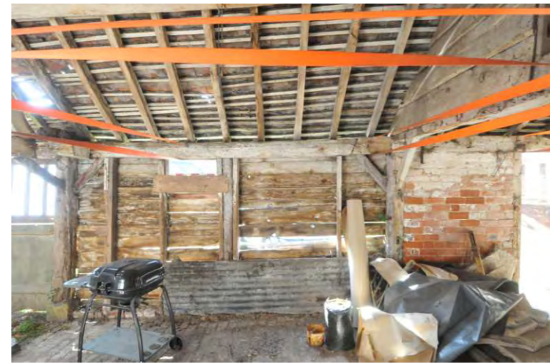
Infill of former open south front
