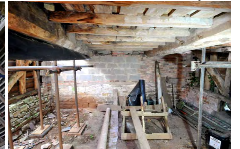
Under-side of hayloft at southern end
