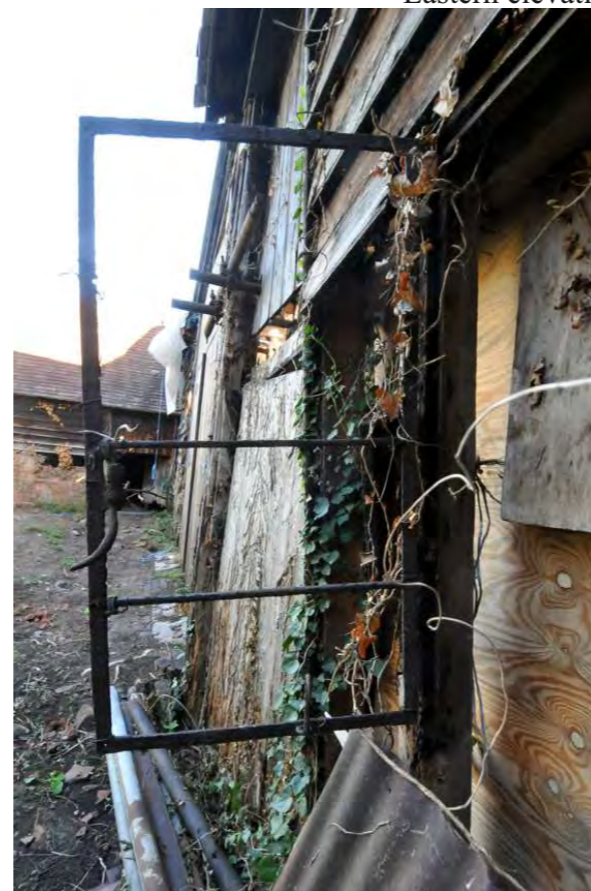
Re-used early 18th C casement (west elevation)
