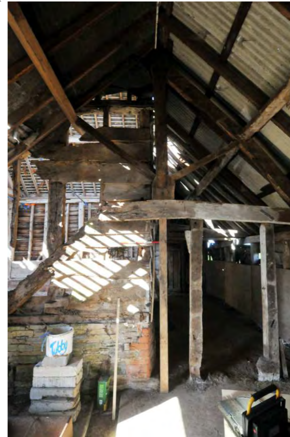
NE corner of barn
