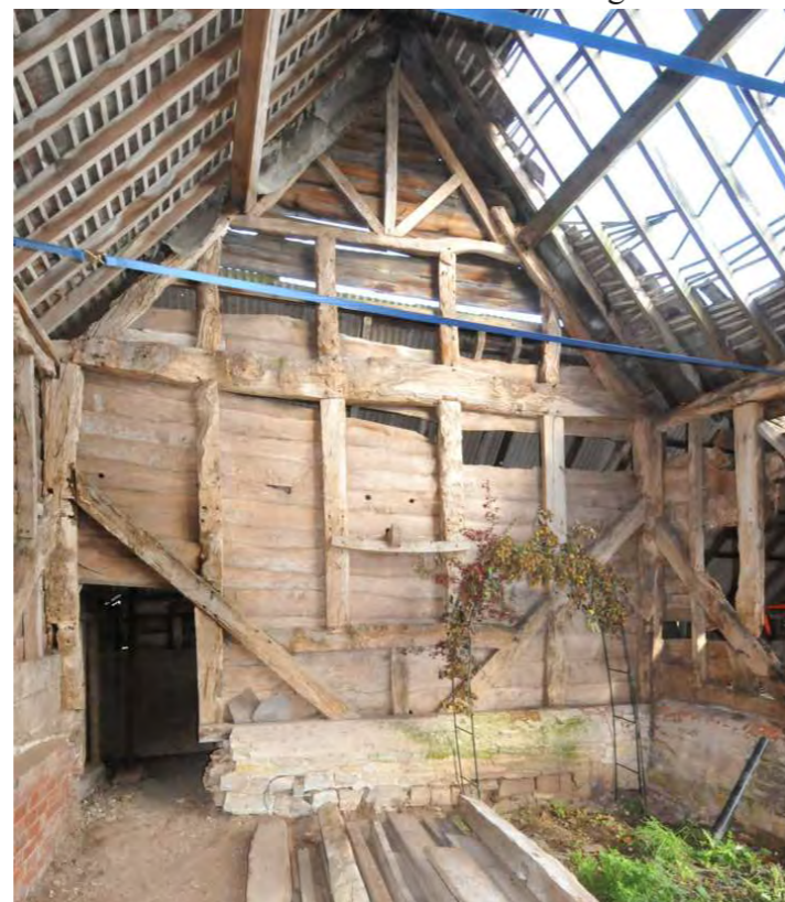
Figure 5: Barn interior - framing includes some re-used elements of a late 17th-early 18th C framed barn but represents a total rebuild with new roof and doorways of circa 1810-30 (Baltic softwood trusses)
