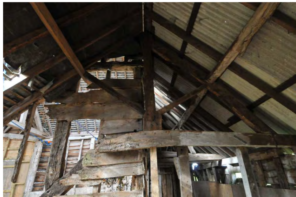
Early 19th C truss in "dairy" against NE corner of barn
