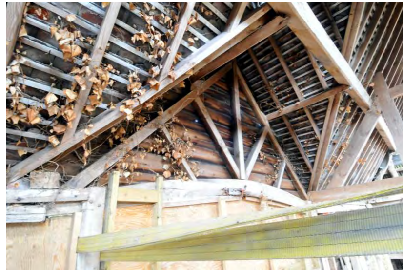
Truss over western door
