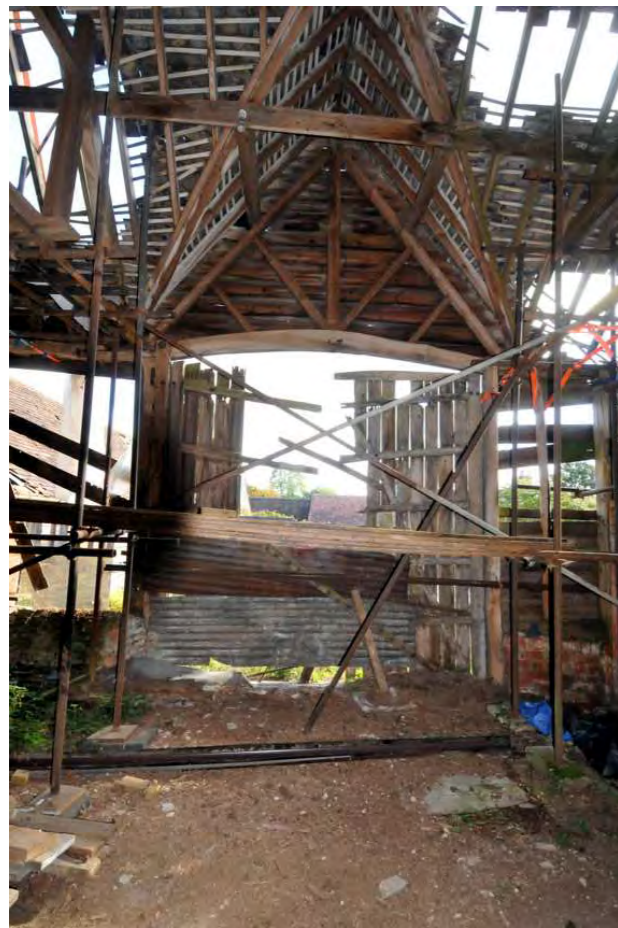
Figure 5: Barn interior - framing includes some re-used elements of a late 17th-early 18th C framed barn but represents a total rebuild with new roof and doorways of circa 1810-30 (Baltic softwood trusses)
