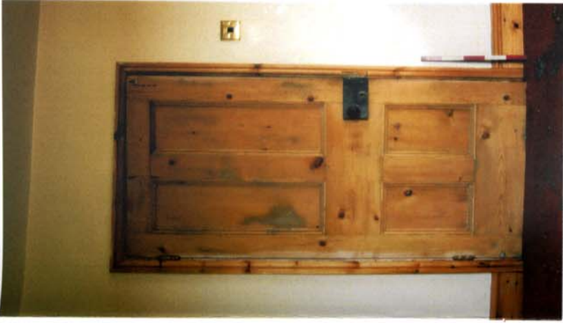
Typical 19th C 4 panel door (Bay 1)
