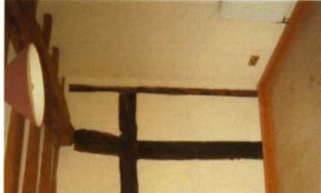
framing (from Bay 3)
