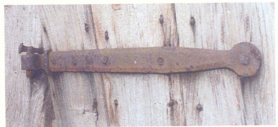
L 17th- 18th C hinges 1st floor doorway, note "anti-lift" nails above pintles
