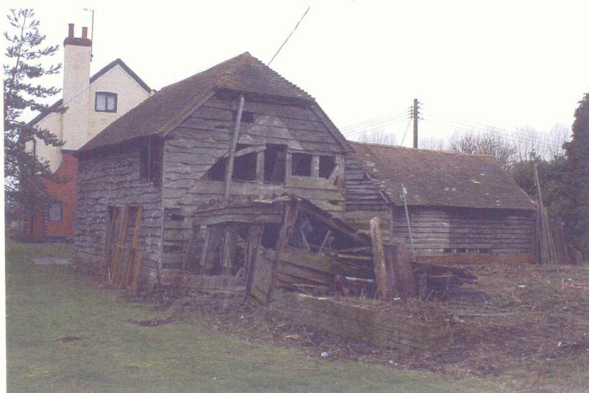
Cider mill-house and other timber framed buildings adjacent to Coventry Arms PH, showing stone plinth of former ?barn (nb: plinth and partially collapsed building in foreground has subsequently been removed to create new drive access)
