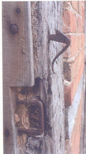
Latch and latch rest 1st floor (L17th - early 18th C)
