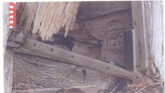
L 17th- 18th C hinges 1st floor doorway, note "anti-lift" nails above pintles
