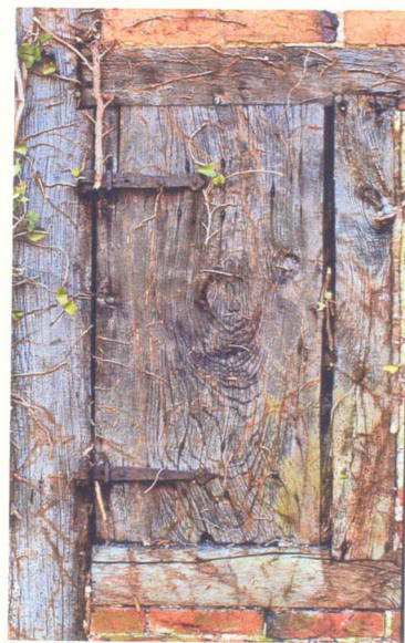
Shutter detail, eastern elevation
