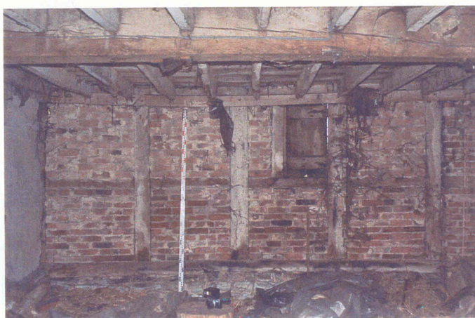
Eastern internal elevation of Bay 2
