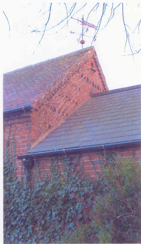
South west gable end - note owl-perch
