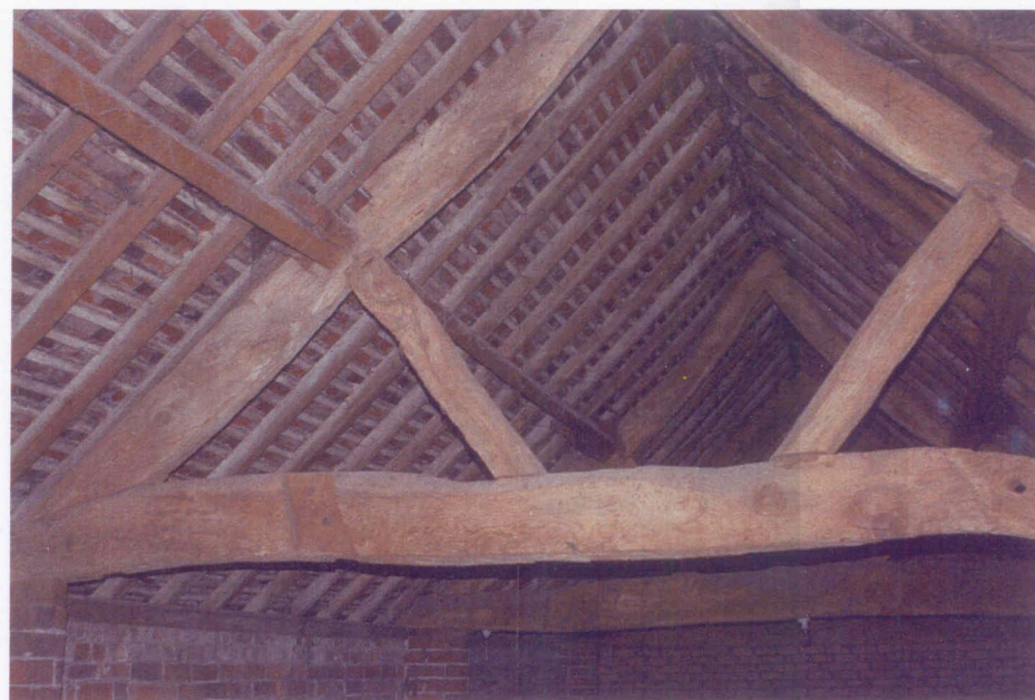
Truss 1 (viewed from hayloft)
