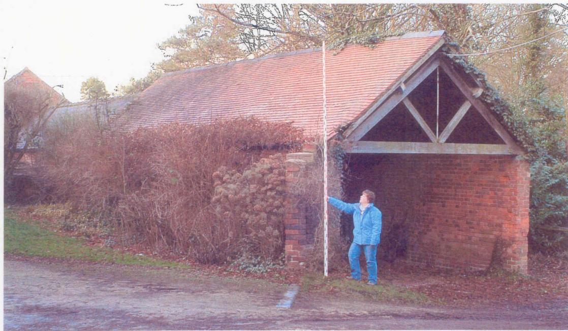
Implement shed from south-east
