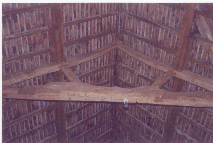
Truss 2 (viewed from below)
