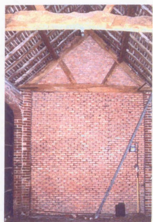
Truss 3, showing blocking wall of Barn Flat
