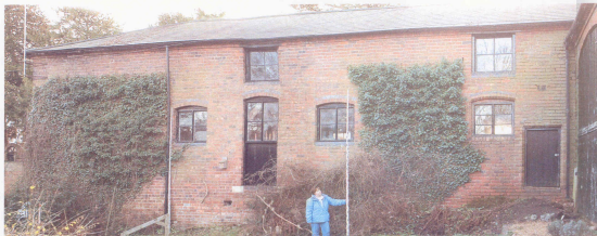
Main stable block - north west elevation
