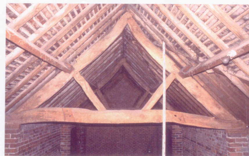
Truss 1 from south
