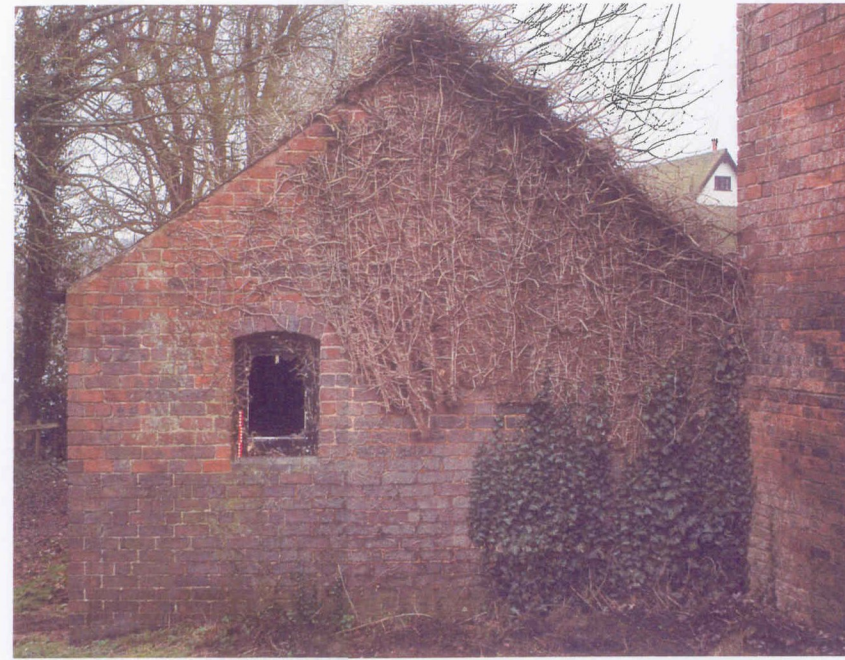
Northern gable end of implement shed range
