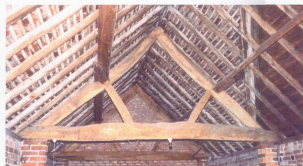
Truss 2 (Truss 3 beyond)
