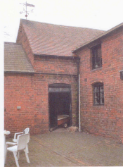
Entrance to stables in barn and west end of stable block
