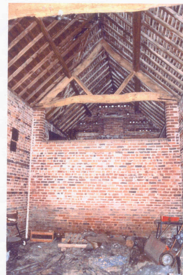
Truss 1 and hayloft
