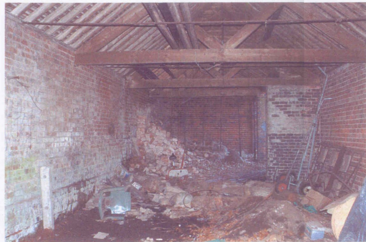
Implement shed - interior
