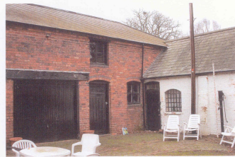
Stable block from courtyard, note inserted garage door and rear door to "Balcony Flat"
