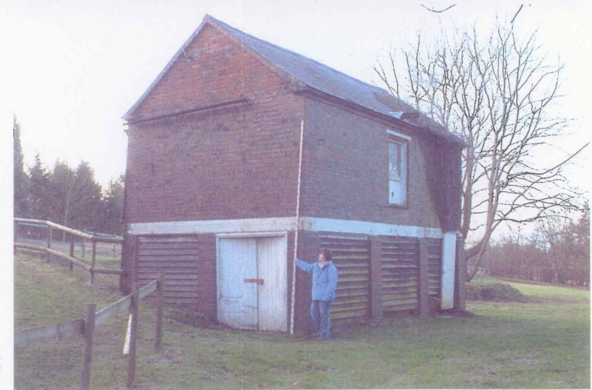
Two storey storage building (on neighbouring property)
