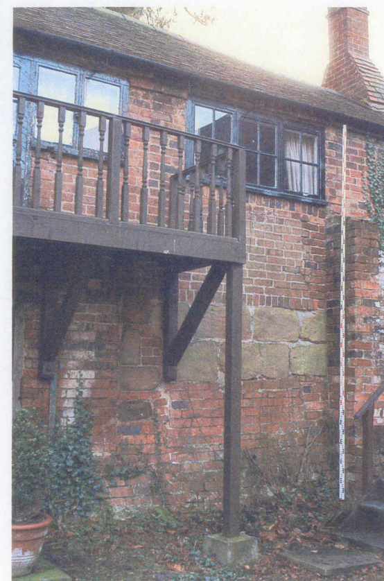
Stone work plinth beneath "Balcony Flat"
