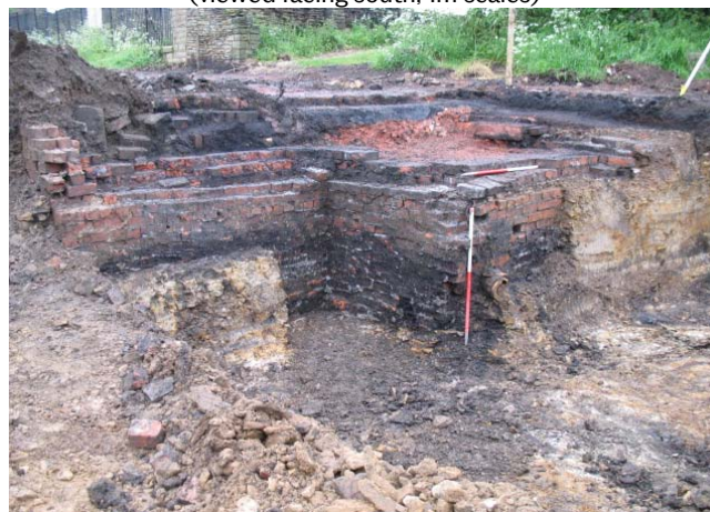
Plate 4 – brick 'soakaway' at west end of cottage (viewed facing southwest, 1m scales)
