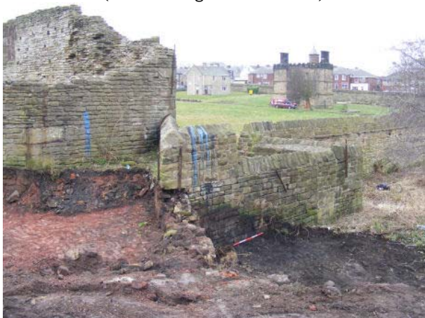
Plate 7 – yard surface 9003 and wall 9002 (viewed facing south, 1m scales)
