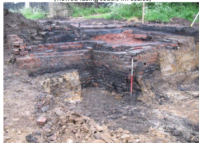
Plate 4 – brick 'soakaway' at west end of cottage (viewed facing southwest, 1m scales)
