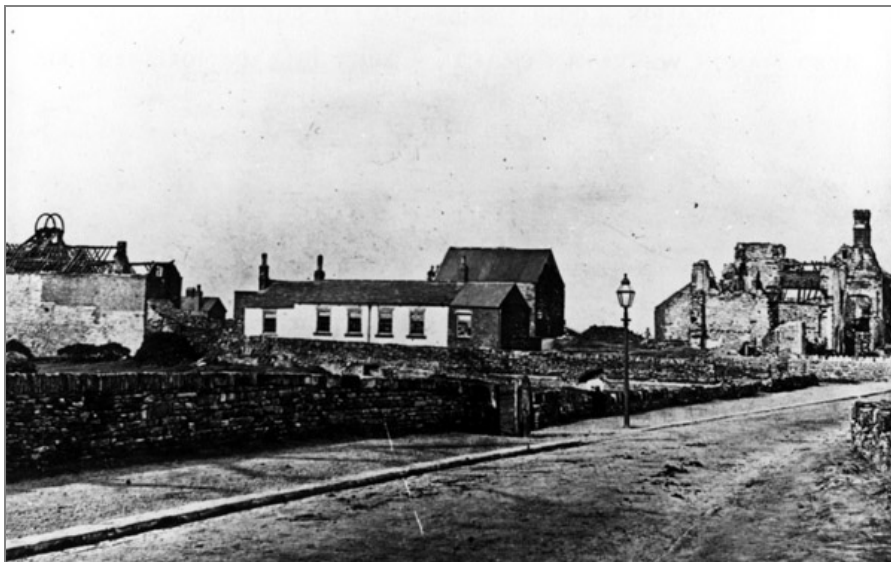
Plate 2 – View east along Manor Lane in the 1870s, showing miners' cottages, the Methodist Chapel (in the centre, with the high roof) and Manor Castle Colliery on the left
