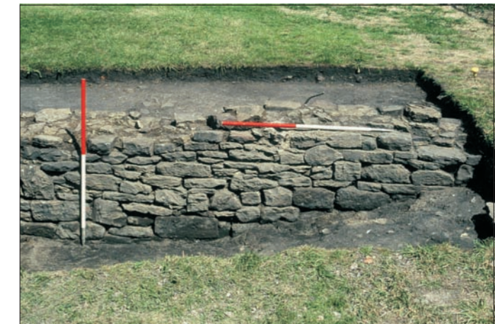
Plate 21: Southern part of wall 14002, viewed from the west
