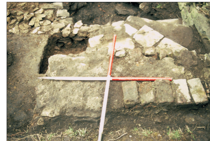
Plate 6: Wall 11007/39/40 and cellar steps 11014, viewed from the north
