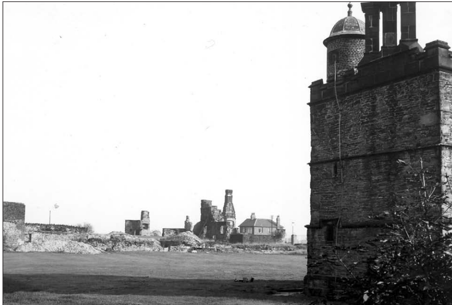
Image 21: Black and white photograph, view from the Turret House, 1970
