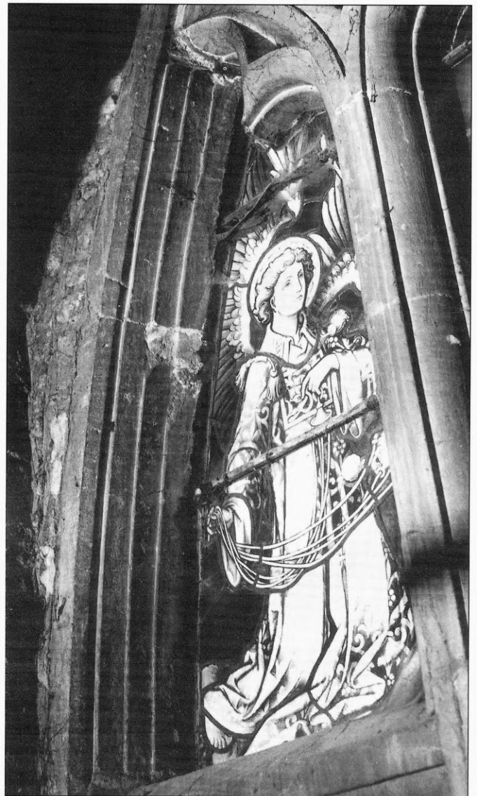
Fig 6 Nave west window, detail of the head; medieval jamb on the left, 17th-century mullion on the right (Photo: R K Morris)
