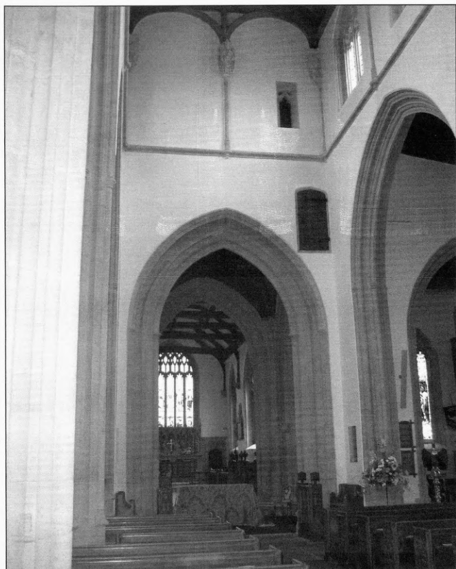
Plate 13: Crewkerne, Somerset - high second door (one of the brackets for the lower loft can be seen on the rear right lower pier)
