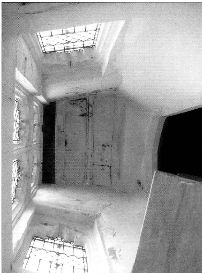
Plate 16: Minehead, Somerset - view of vault of turret & upper door, from stair
