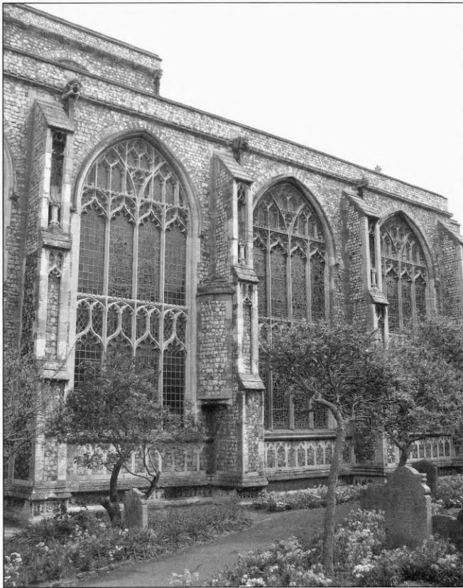
Plate 10: Cromer, Norfolk - shallow multi-angular turret below buttress
