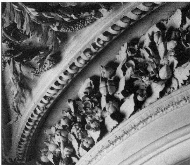
Fig 1: Detail of the nave ceiling.
