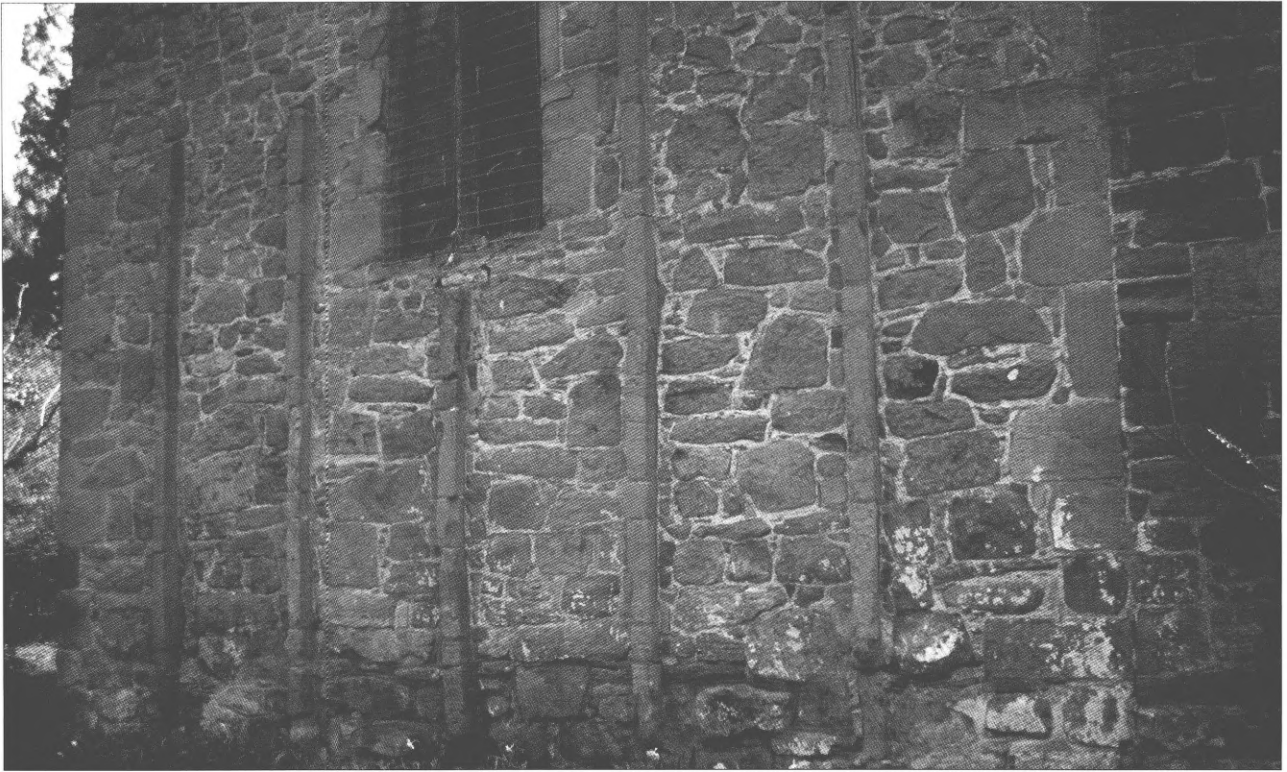
Fig 8 – The west end of the nave at Stanton Lacy church showing five proud, partial pilaster strips, in which a few stones exhibit small cut backs. It should be noted that the quoins, although of Anglo-Saxon age, are flush with the wall; evidence that originally the wall was unlikely to have been rendered
