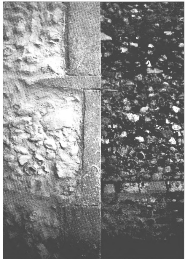
Fig 10 – Detail of part of the north-west quoin, north face, of St Peter, Claydon. Only the 'long' stones have been cut back, apparently to make the sides of the stones parallel for they do not line up vertically in the face. The neighbouring churches of Debenham and Hemingstone possess similar quoins of Barnack Stone and it is possible that all three obtained their stone already worked in this way directly from the quarry. The inserted pen is 145mm long
