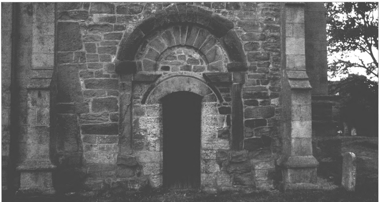
Fig 9 – The north door to the Anglo-Saxon porticus at Laughton-en-le-Morthen church. The north face to the north-east quoin of the porticus in long and short style remains and is noticeably flush to the north wall. The hood-moulding and the voussoirs of the arch to the Anglo-Saxon doorway are constructed of cut back stones to provide both structures with a constant ornamental width. A later medieval door now fills the entrance
