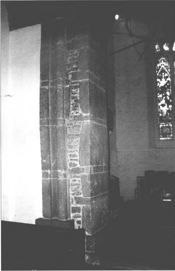
Fig 12 – The south jamb of the Anglo-Saxon tower arch of St Bene't, Cambridge viewed from the east side. Certain stones on the inner side of the strip-work have been cut back to bring them in line with the width requirements of the narrowest stones
