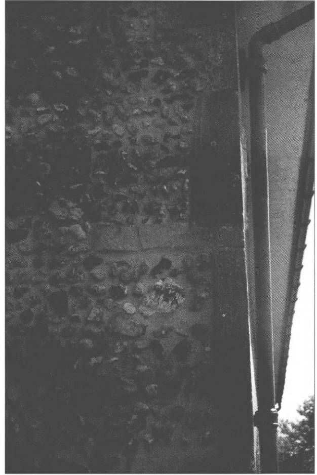
Fig 13 – Detail of an unusually cut back, 'long' stone in the west face of the south-west nave quoin at Hemingstone church. The cut back has been worked parallel to the 'wrong' edge of the stone. It is possible the stone (from Barnack) was cut in the quarry originally for another purpose
