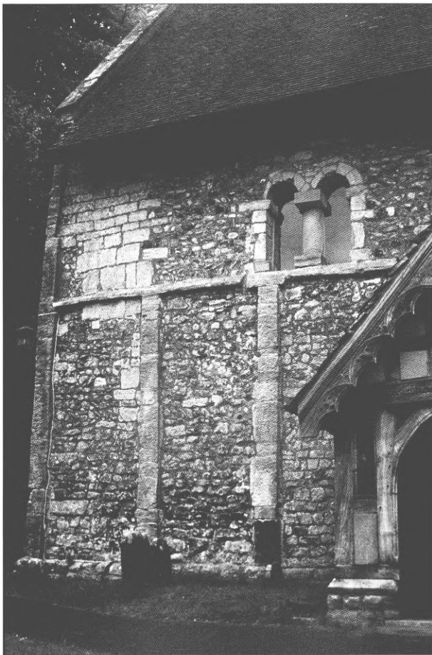
Fig 6 – The south wall of the nave at St Nicholas, Worth, showing a number of cut back stones in the pilaster strips and also the south face of the south-west quoin. In the upper portion of the quoin, where the proud face suddenly changes in width, the quoin and the adjoining wall are of post-Conquest age and the cut back stones are of a different style
