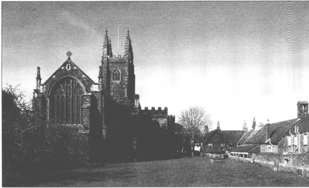
Fig 2 – View of the church from the north-east, with the old priory buildings on the right
