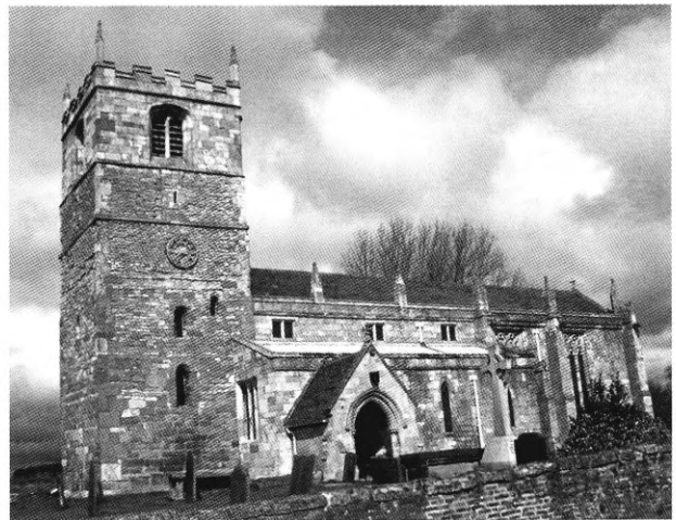
Fig 1 St Helen's Church, Skipwith, North Yorkshire, from the south-west (photograph, Richard Hall)
