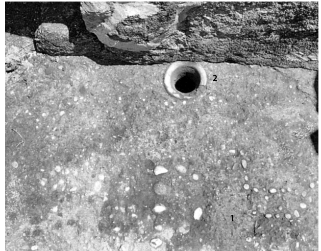
Fig 6 Noli (SV); San Paragorio: detail of floor with inscription in sea pebbles (1) and shown on Fig 3/2 above: neck of amphora inserted in opus signinum floor (2), (Frondoni 1988, 104)
