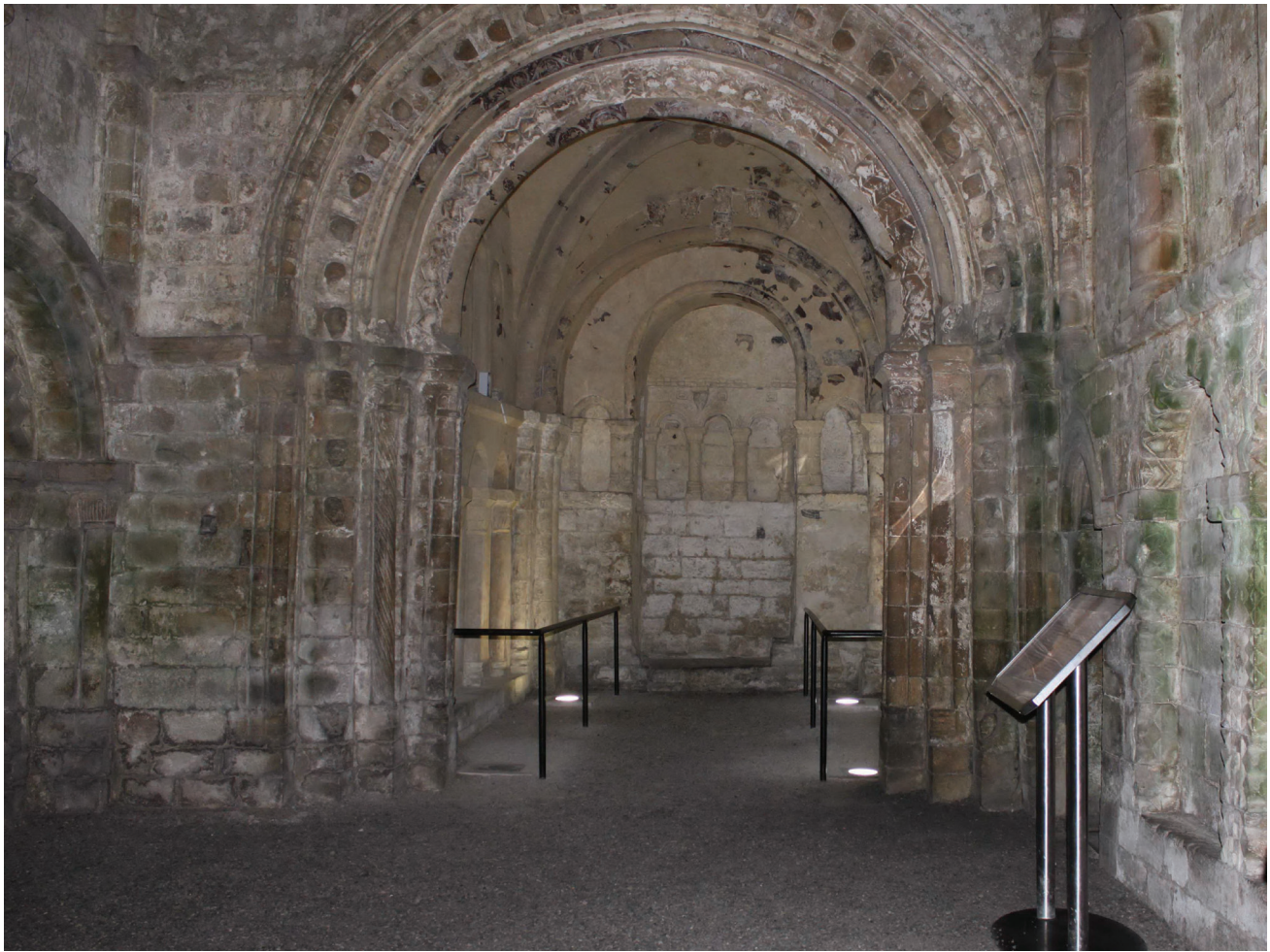
Fig 7 Photo showing the mis-alignment of the nave and chancel of Cormac's Chapel (Photo: author)
