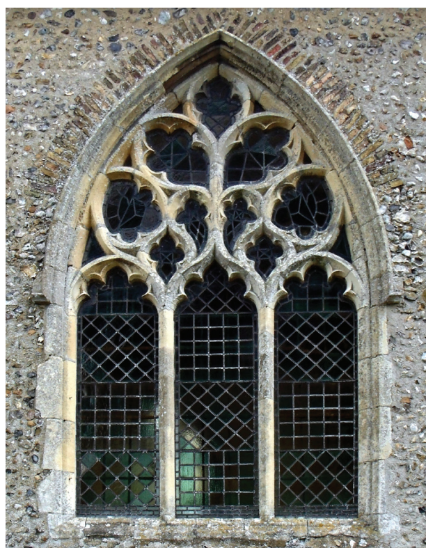
Fig 9 Curvilinear tracery window from the south side of the chancel at Weston Longville, apparently related to one of the small scale architectural designs recorded on the south arcade of the nave (Photo: author)
