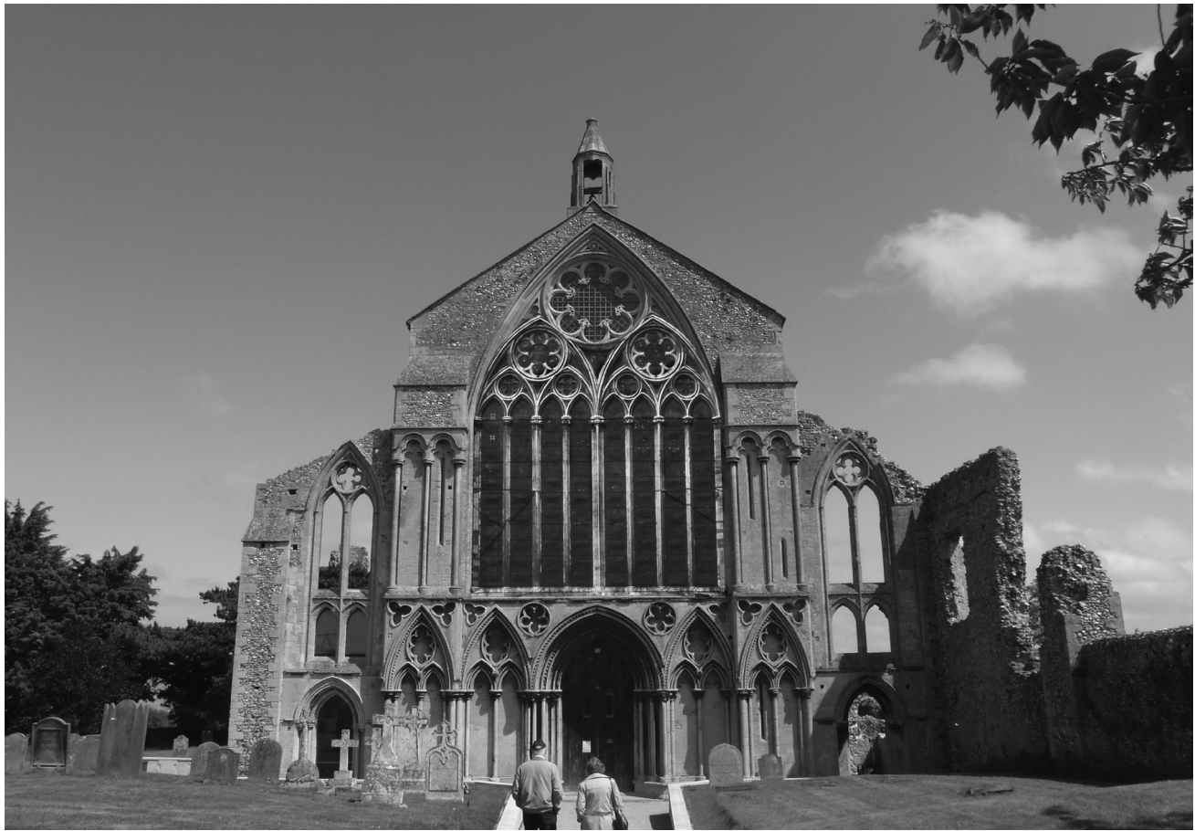
Fig 2 Tentative reconstruction of the original eight light west window at Binham priory as it may have looked prior to its failure in the 18th century (Author)
