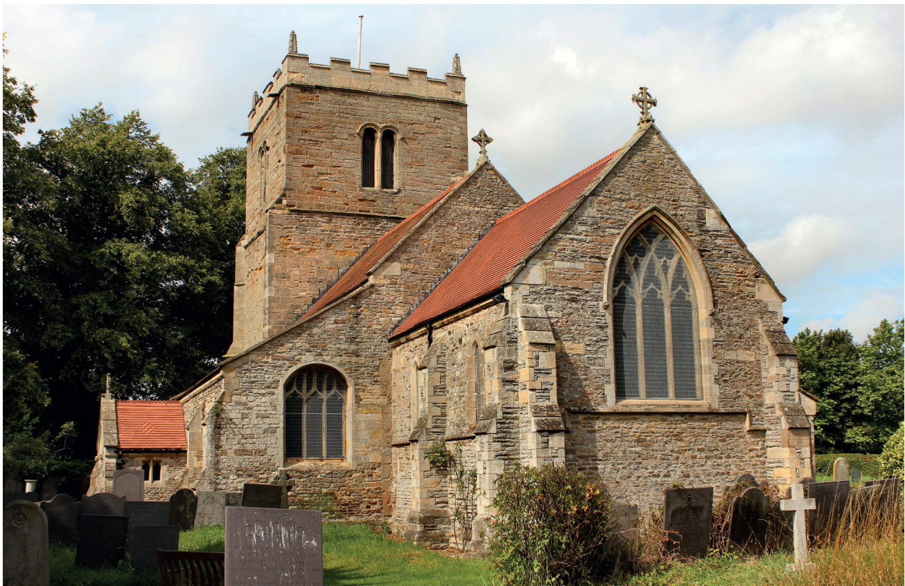
Fig 11 Screveton, St Wilfrid, church and tower from the south-east (Photo: CJ Brooke)
