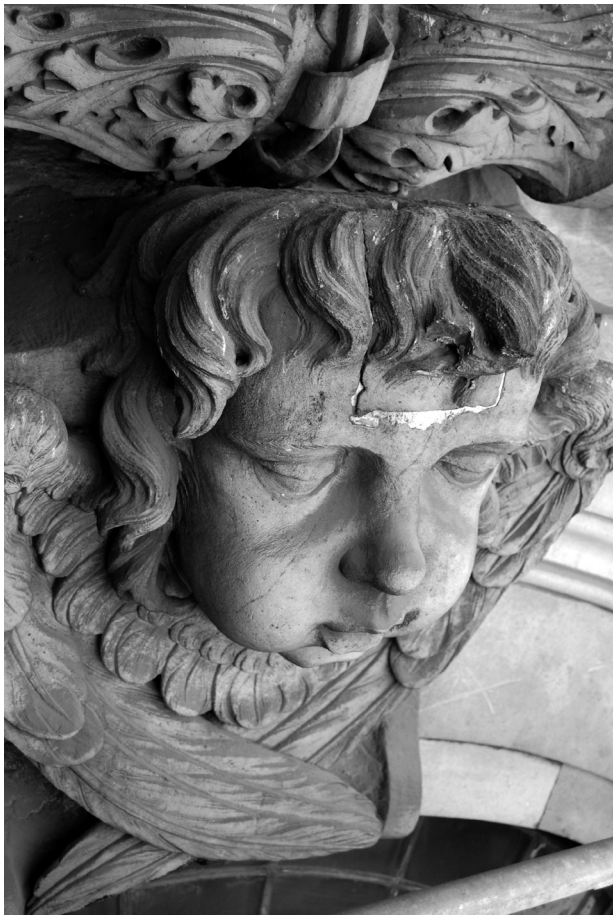
Fig 5 A cherub carving above one of the windows of the choir, before cleaning. In several cases the head has this odd feature, as though part of the stone has been replaced. Or is this to do with the method of attachment of the heavy piece to the wall? (Photo: Author)
