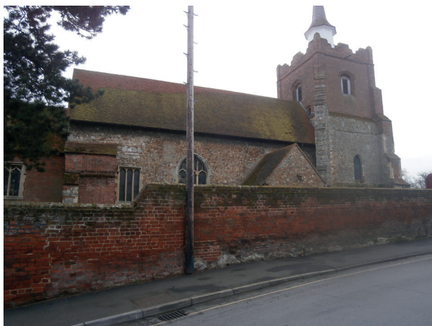
Fig 1 St Mary, Maldon: general view from north (Photo by D. Secker)
